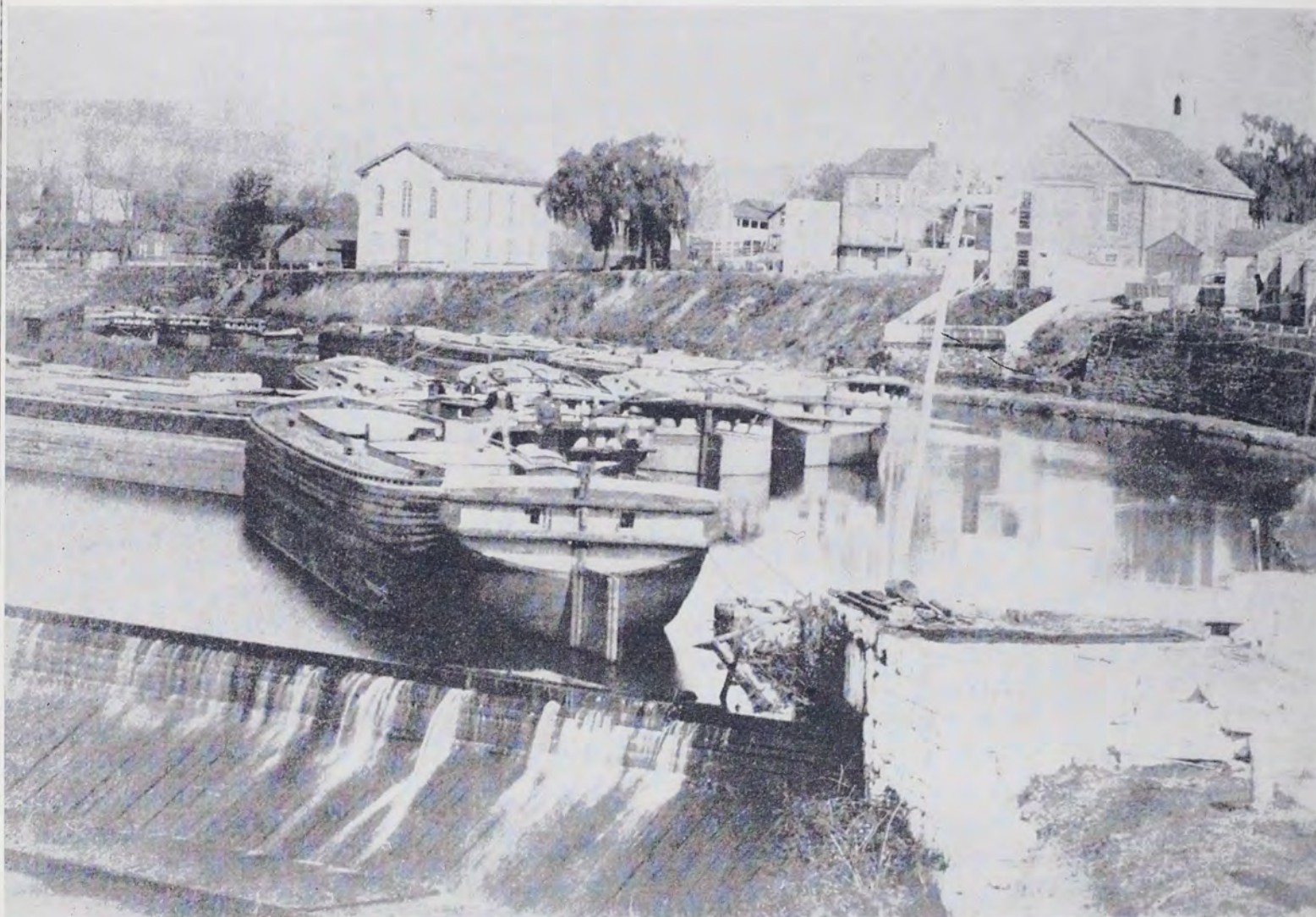
A view of Dam number seven of the Schuylkill Canal at Schuylkill Haven. This photograph was taken about 1880. The boat in the foreground shows no stable, therefore it is a "company boat" of the scow type.
