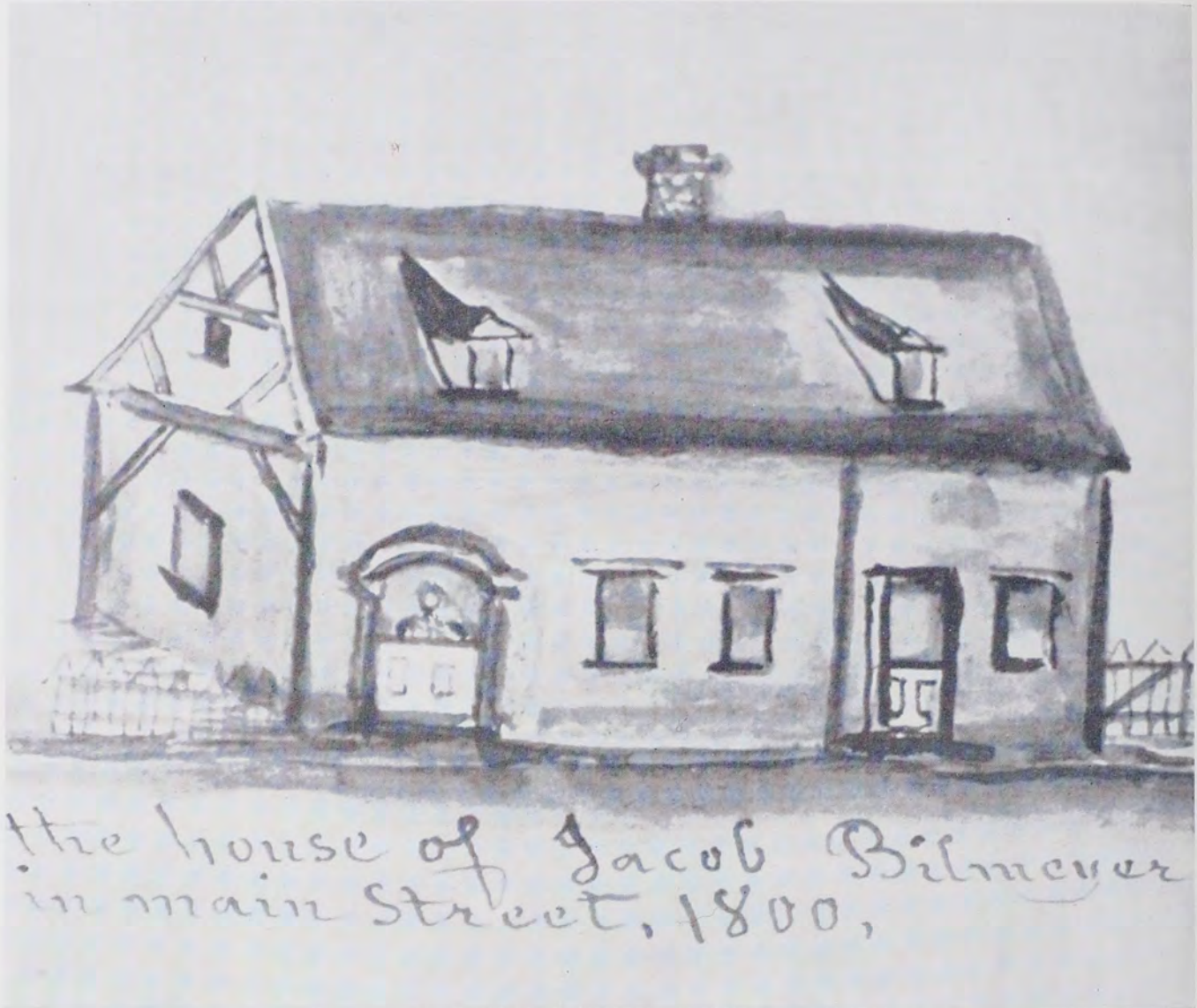
Fig. 7—A house in York with gable-end half-timbering, sketched by Lewis Miller, famous primitive artist.
