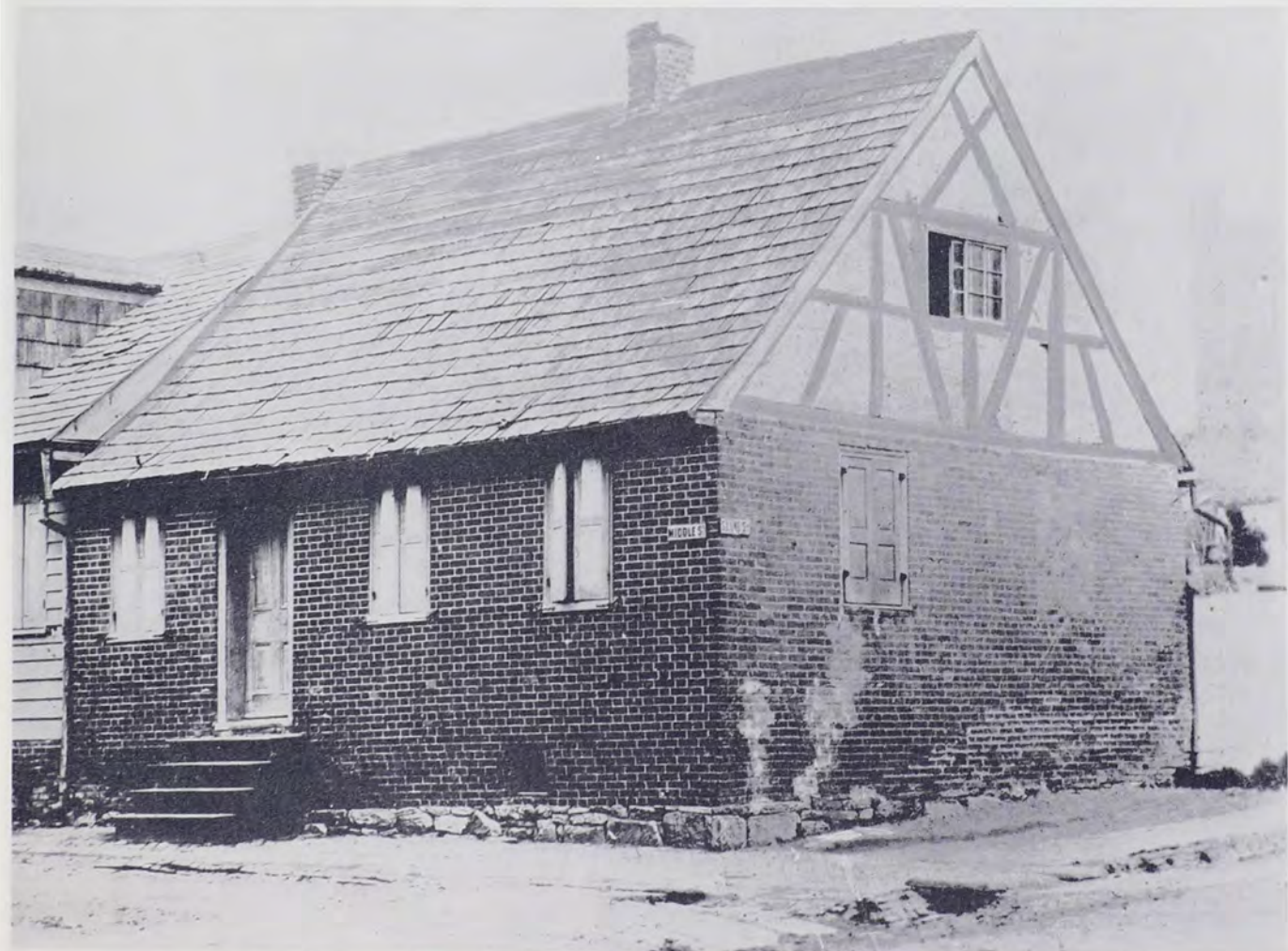
Fig. 2—A one-and-a-half story brick house (no longer standing) with half-timbered gable end in Lancaster.
