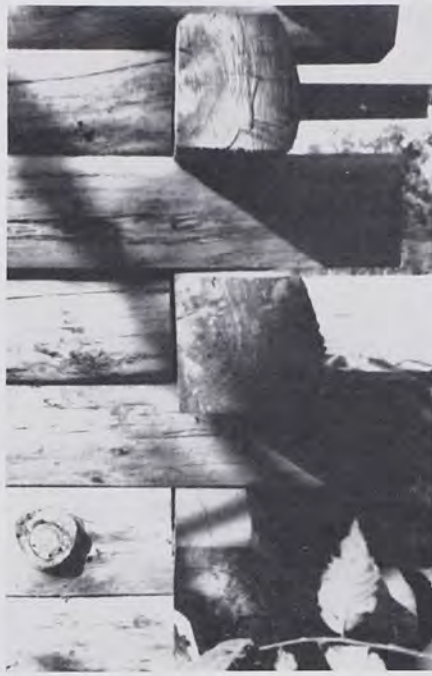
Fig. 17 Butt joint false corner timbering on Cherokee County house under construction in 1991. Logs have been sawed flat on all but the exterior side.
