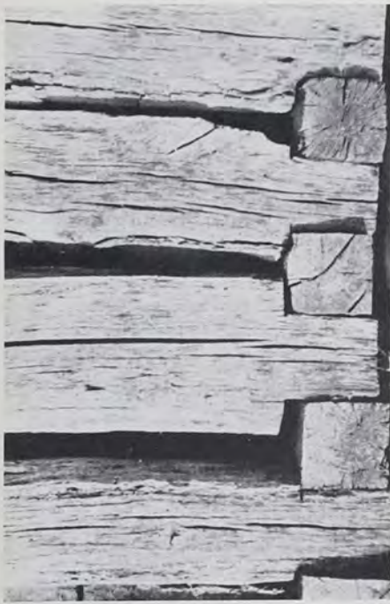
Fig. 13 Hewn logs with square notches, Cherokee County, late 1800s.
