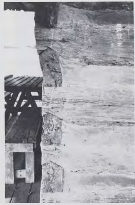
Fig. 15 Boxed V-notches on hewn log dogtrot house, Sequoyah County, 1845.
