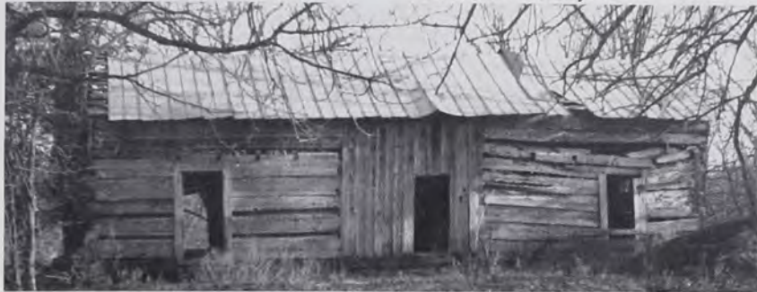
Fig. 4 Central hall log house with enclosed breezeway, Cherokee County. Said to pre-date the Trail of Tears of 1838-1839.
