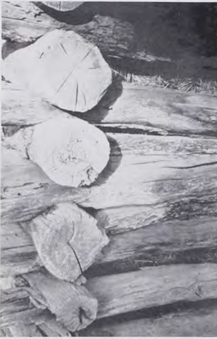
Fig. 16 Round log V-notches with blunted apices and crowns intact on single crib-barn, Adair County.
