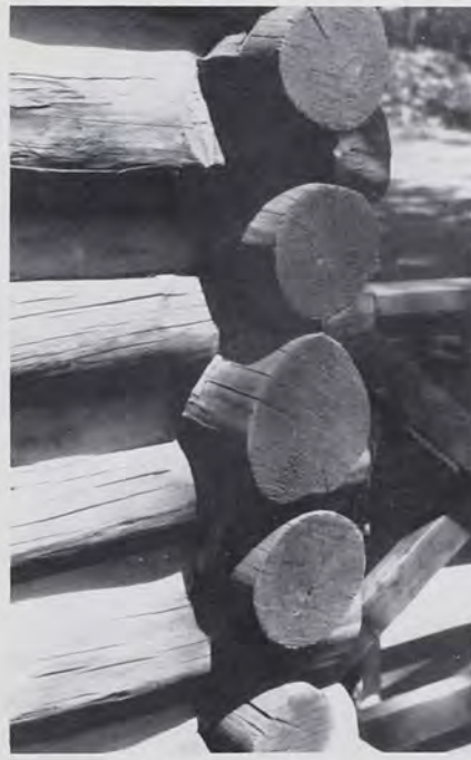
Fig. 14 Peeled round logs with mostly undersided saddle notches, Cherokee County, 1930s.
