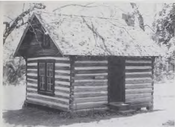
Fig. 2 Single pen log dwelling built in Tahlequah in about 1870 and moved to the nearby Murrell Home Historical Site.
