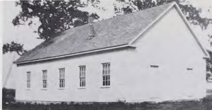
The Lexington Church, built by Thomas Major and Gideon Moore in 1849. Located about two miles south of Lexington (now called Highland) Ohio, it was a 45' x 60' frame structure. (History of the Church of the Brethren of the Southern District of Ohio by the Historical Committee, 2nd ed. [Dayton, Ohio: 1921], p. 65.)
