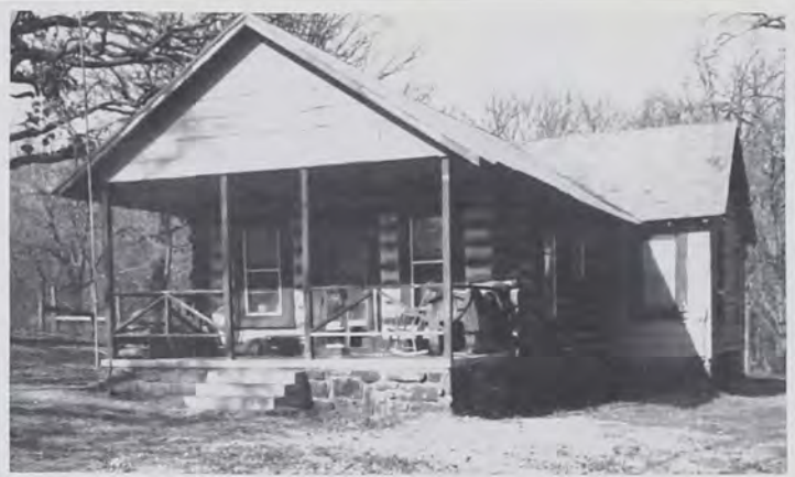
Fig. 3 1930s vintage Finnish plan dwelling with cantilevered frame front porch and later rear addition, Cherokee County.
