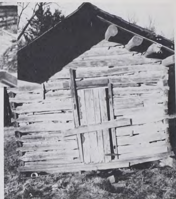
Fig. 11 Adair County kitchen, probably built in the late 1800s. The kitchen was formerly attached to a larger log dwelling. Note purlins, hewn logs, and V-notches.
