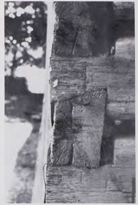
Fig. 18 Half dovetail notches on a nineteenth century kitchen of hewn and scored logs, Cherokee County.
