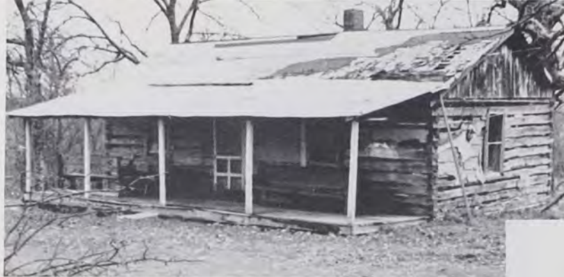
Fig. 5 Central chimney, Beaver Church, Adair County, late 1800s. Central chimney log churches were not uncommon in the pre-statehood period.
