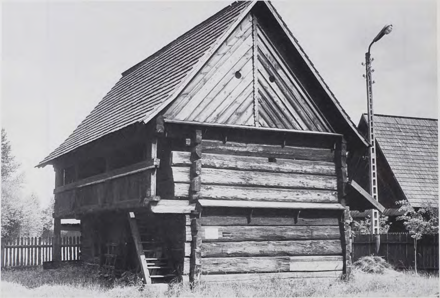
Fig. 30: Galerie forebay on a storage barn in the Opole district of Upper Silesia (field research district 14). The structure, now in the open-air Muzeum wsi Opol-
