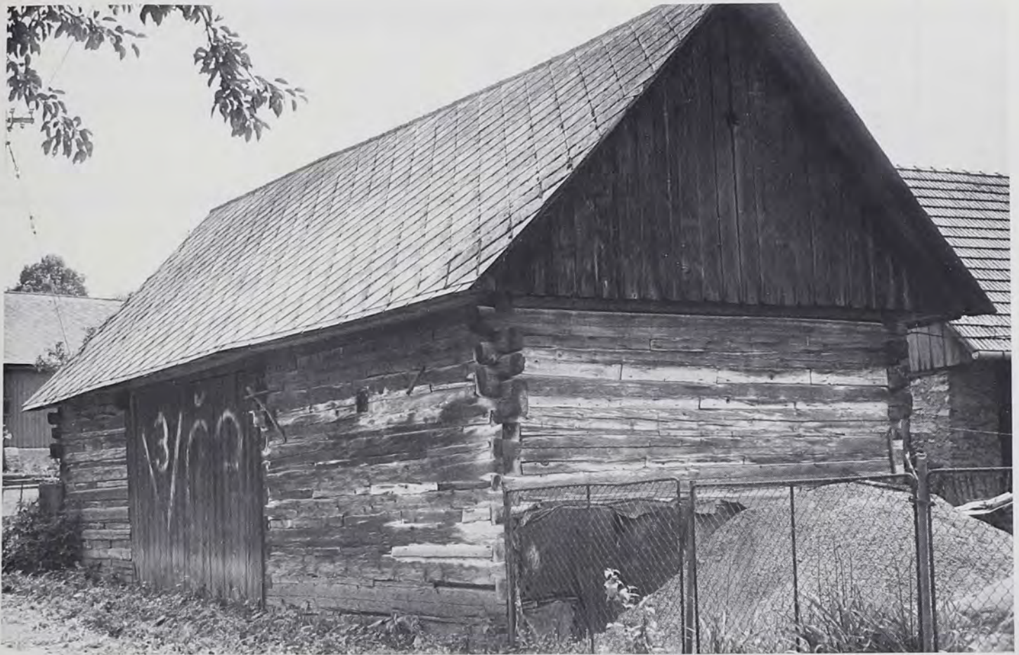
Fig. 27: The simplest of the western Slavic double-crib log barns, in the village of Čičmany, Rajčanka Valley,
