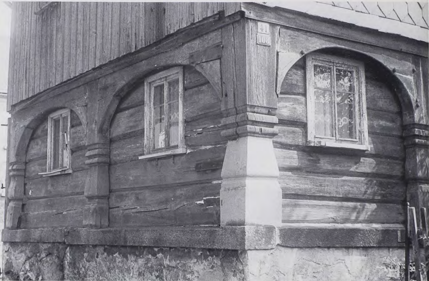
Fig. 13: The false chinking was left off of this house in Neukirch, a Brethren source village in the Lausitzer Hills, Saxony, in the German Democratic Republic (field research district 9), revealing the chinkless nature typ-
