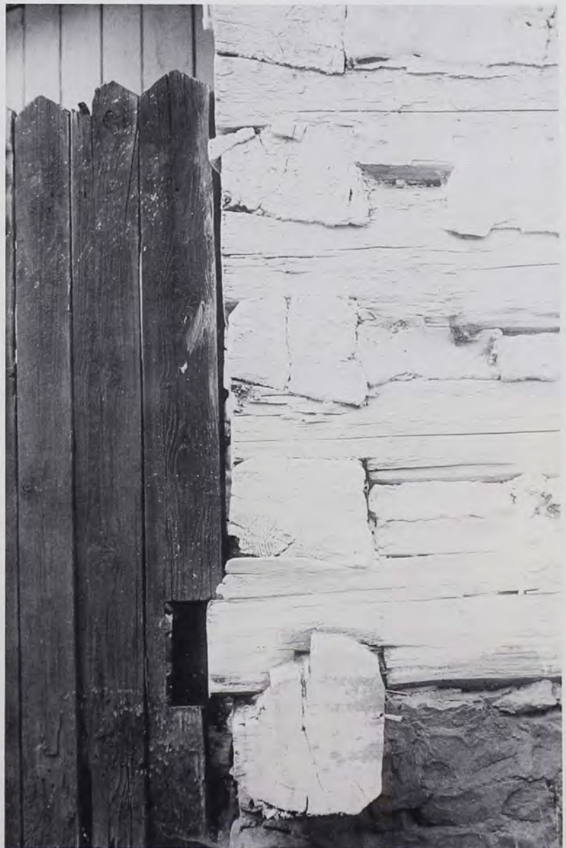
Fig. 19: Inverted half-dovetail notching on a chinked, white-washed log house in Letohrad (Geiersberg), near Lanškroun in northeastern Bohemia (field research district 3).
