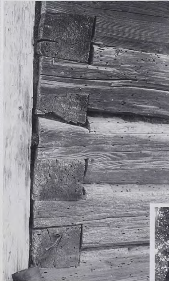
Fig. 15: Chinkless wall of a log house in Životice (Seitendorf), just south of Nový Jičín in the Kineland, eastern Moravia (field research district 5). Note the gently-splayed full-dovetailing, two-sided hewing, and thick logs.
