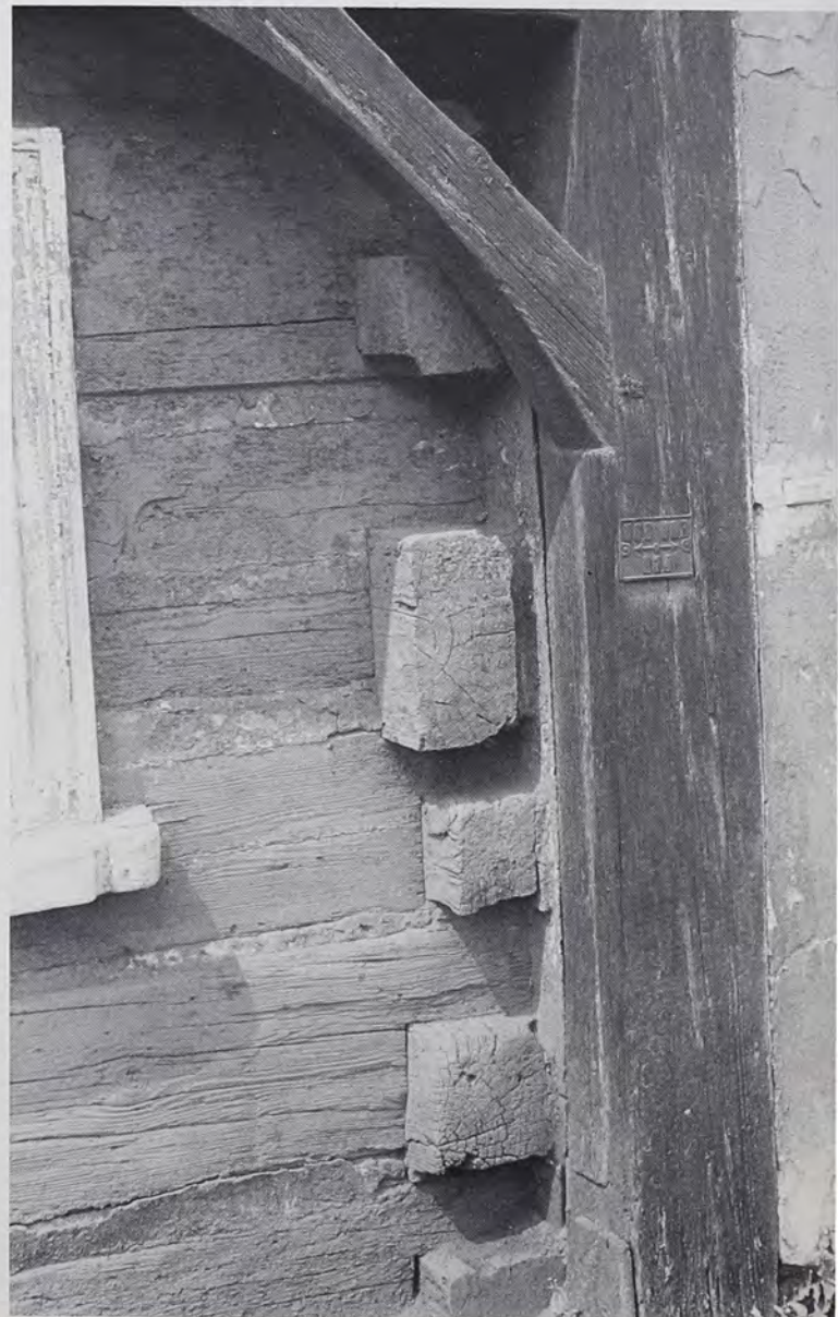
Fig. 21: Half notching on an Umgebinde log house in Hirschfelde, Saxon Upper Lausitz, German Democratic Republic (field research district 1). Similar half notching, without Umgebinde, appears as a minor type in America.
