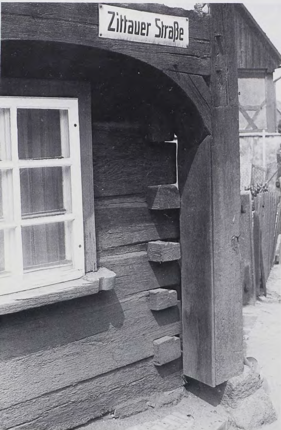
Fig. 1: A log house in Saxony with hook and square notching, false chinking, and Umgebände construction—typical features of wooden dwellings in Upper Lausitz—in Hirschfelde, near Zittau and Herrnhut, German Democratic Republic (field research district 1). All photographs by T. G. Jordan, 1982.
