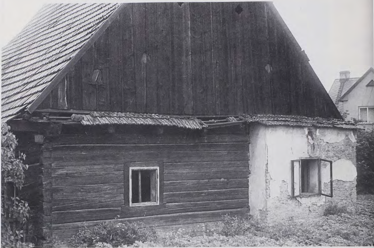
Fig. 5: Log house in Libhošt (Liebisch) in the Kineland (field research district 5). Note the chinkless construction, full-dovetailing, board gable, pent roof, and masonry covering a portion of the wall. Liebisch is a family name found among Pennsylvania Brethren de-
