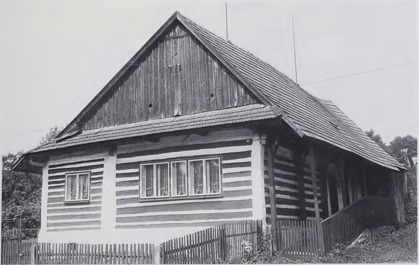
Fig. 22: Corner posting on a log house in Libchavy (Lichwe), near Litice nad Orlicí in northeastern Bohemia (field research district 4). This method of corner
