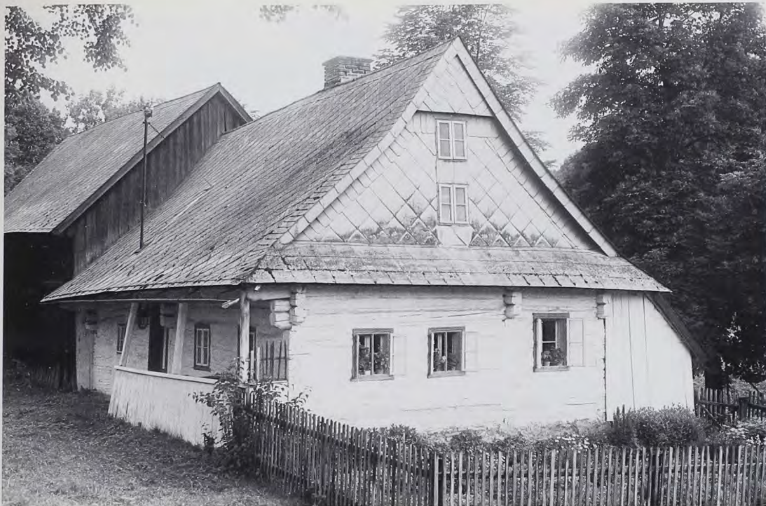
Fig. 25: A “continental,” story-and-a-half log house in Koburk (Koburg), near Výprachtice (Weinersdorf) in the region of Lanškroun, northeastern Bohemia (field research district 3). Note the attached stall, a Frankish
