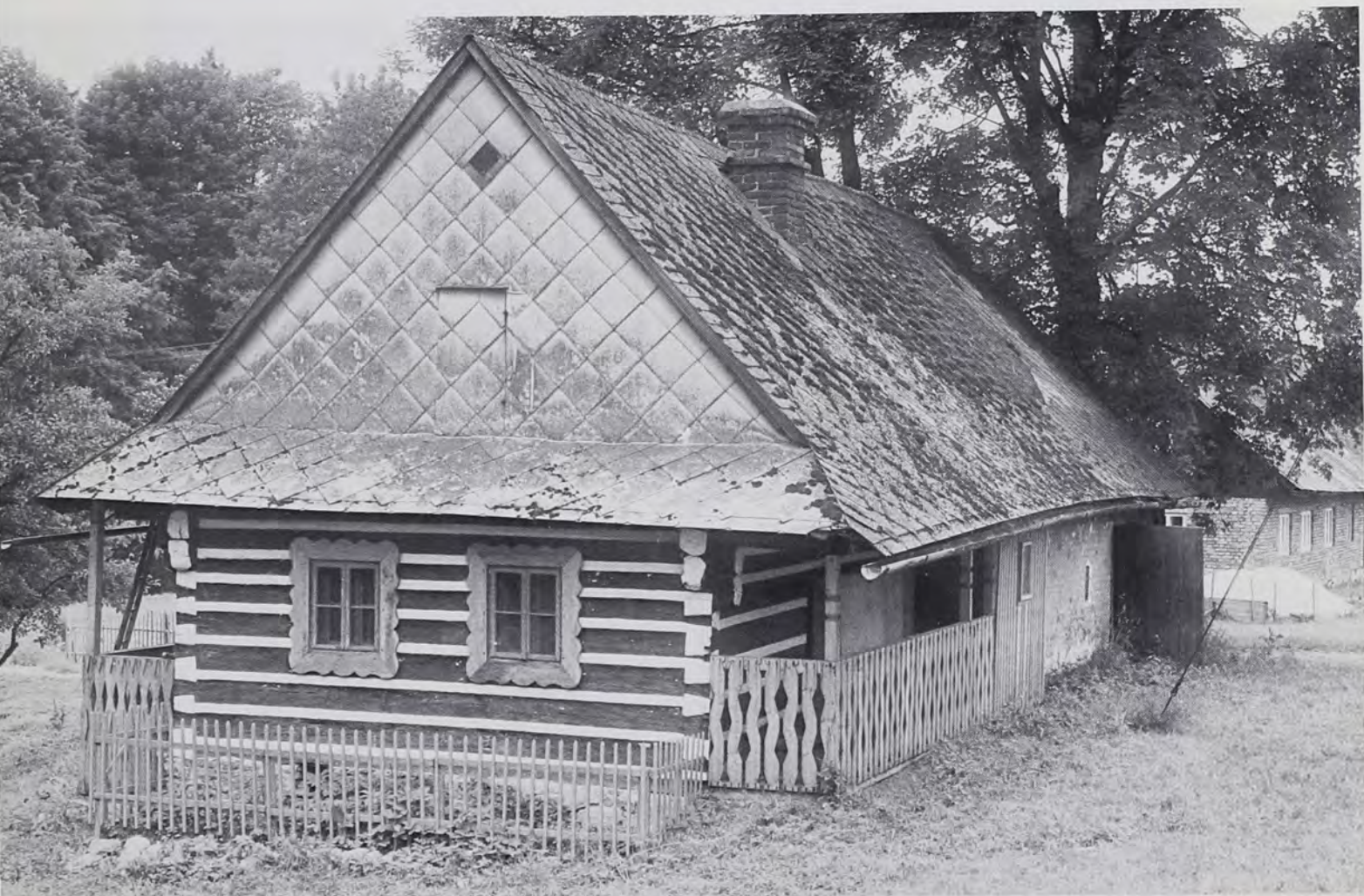
Fig. 2: A chinked "continental" log house with attached stall, at Horni Heřmanice (Ober-Hermanitz), a Brethren source village near Lanškroun in far north-eastern Bohemia (field research district 3). Note the full-dovetailing, gable pent roof, and decoration.
