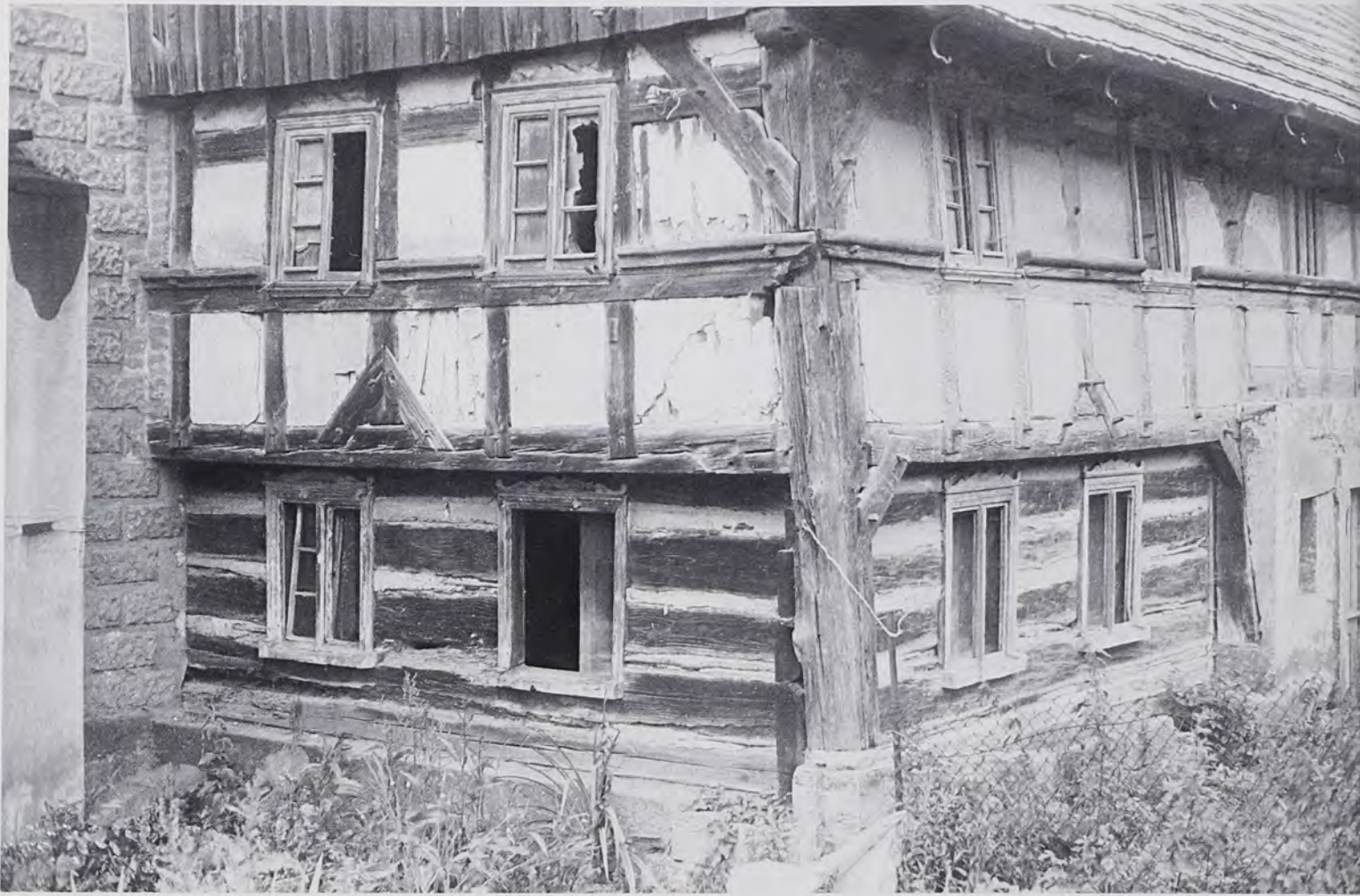
Fig. 7: Abandoned log and half-timbered Umgebnde house in the village of Raciborowice (Gross Hartmannsdorf) in the Schwenkfelder source region of Lower
