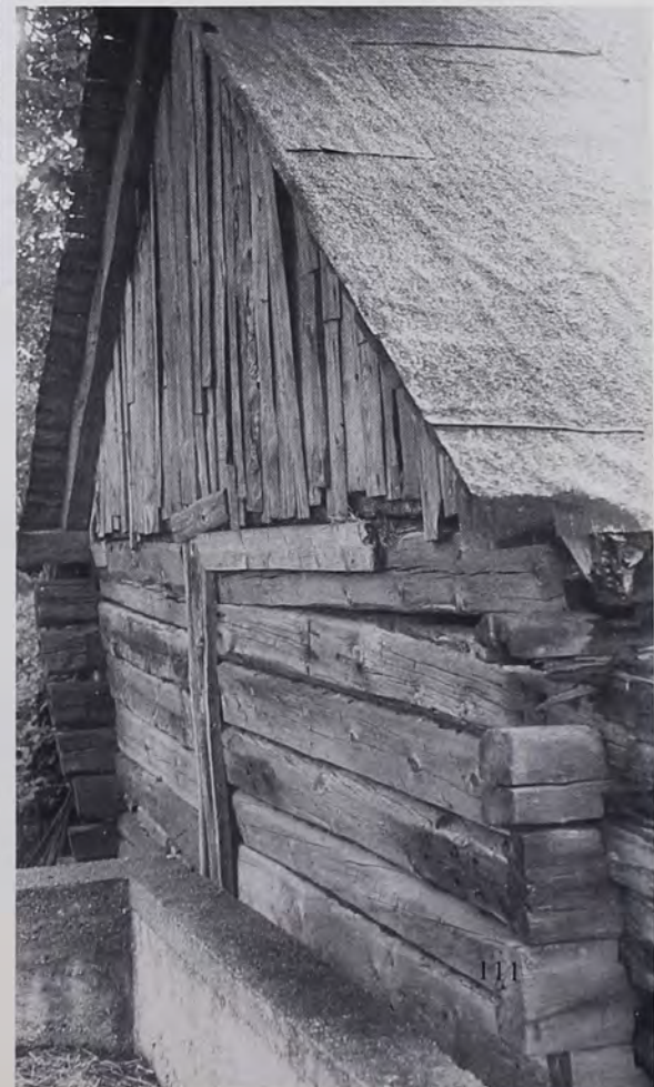
Fig. 16: Double-notched, chinkless log outbuilding in the Schwenkfelder source village of Nowa Wieś Grodziska (Neudorf), Lower Silesia, Poland (field research district 7). Note the vertical boards in the gable.
