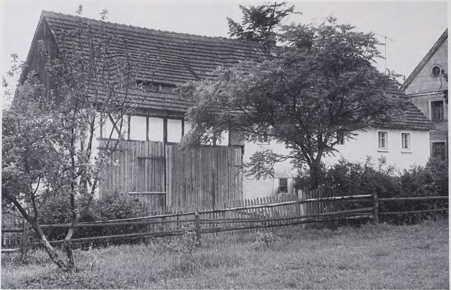
Fig. 26: A two-story "continental" house with attached stall in the Schwenkfelder source village of Czapple (Hainwald) in Lower Silesia, Poland (field research
