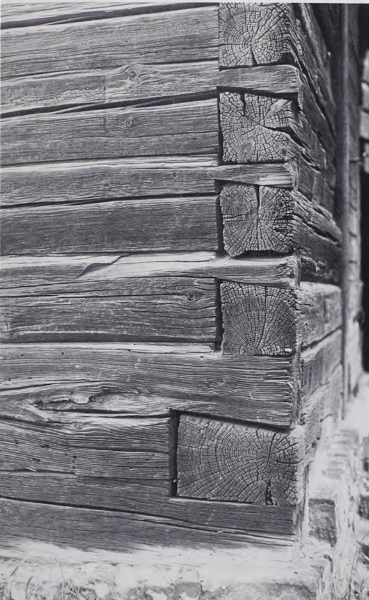
Fig. 18: Half-dovetail notching on the venerable log church at Koszęcin (Koschentin), located between Częstochowa and Katowice (Kattowitz) in Upper Silesia, Poland (field research district 17). Half-dovetailing, assumed by many to be an Americanism, occurs widely in the German-Slavic borderland. Note also the typical Upper Silesian chinkless construction.
