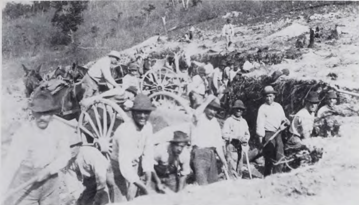
These southern and eastern Europeans constructed a reservoir on the west branch of the Schuylkill in Forestville, Schuylkill
