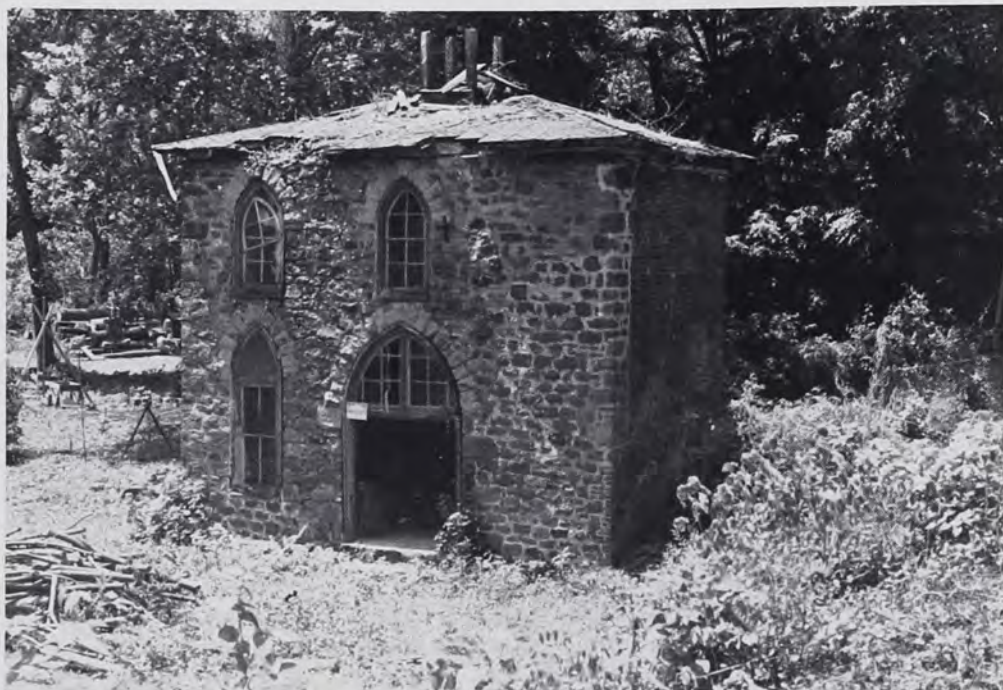
The blower engine house as it appeared in 1980, before restoration.
