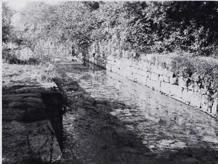
Lock on the Schuylkill Canal at Auburn (1950).
