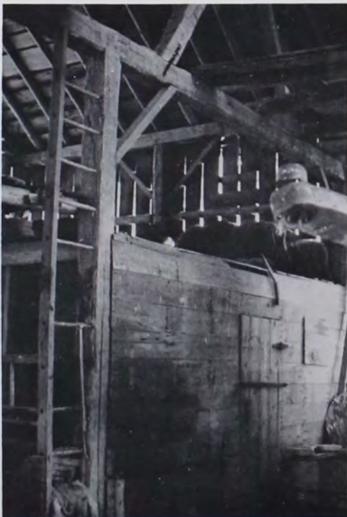
Granary in forebay; Martin barn, Washington County, WI (c. 1885).
