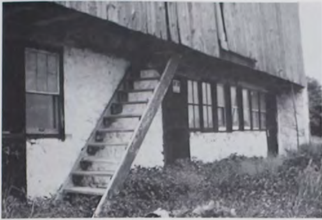
Type H forebay barn, Washington County, southeastern Wisconsin (c. 1890) with stairway to forebay.
