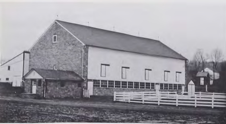
Reifsneider barn, Berks County, PA (c. 1845) showing enclosure of under-forebay area resulting in basement barn form.
