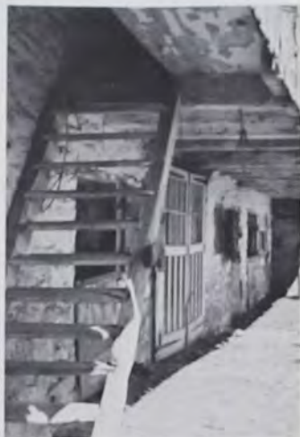
Bertolet-Coker barn, Berks County, PA (1787); stairway to forebay.
