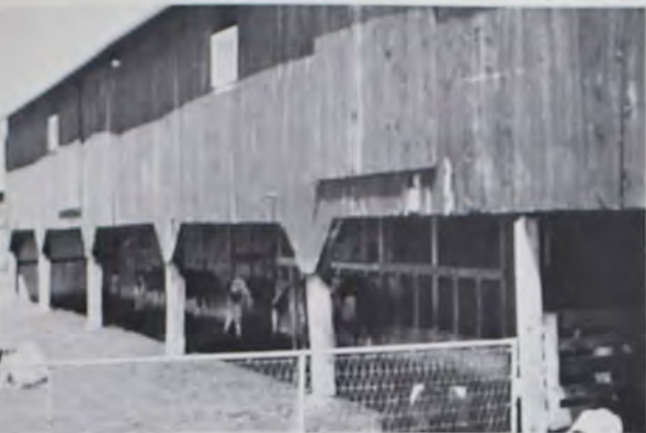
Herman Schield barn, Lincoln County, WI; supported and arcaded forebay with under forebay stable doors.
