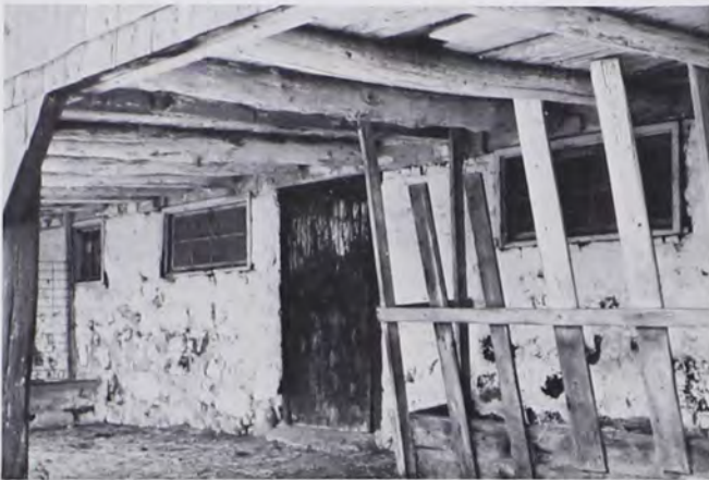
Forebay barn near Jefferson, Jefferson County, WI showing under-forebay stable door and forebay joists mortised into sill above stable wall (c. 1870).
