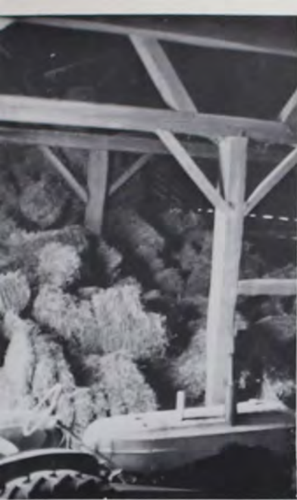
Herman Schield barn (1908), Lincoln County, WI showing threshing floor, mows, and heavy mortised and pinned frame.
