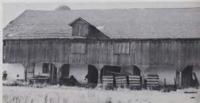
Krausie barn (1912), Marathon County showing under forebay double "Dutch" doors and dormer gable.
