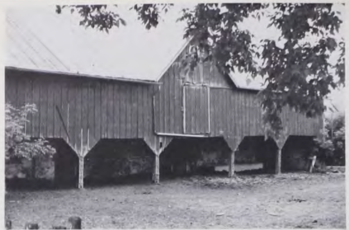
Votsis barn, Jefferson County, southern Wisconsin showing supported and arcaded forebay and dormer above (c. 1870).
