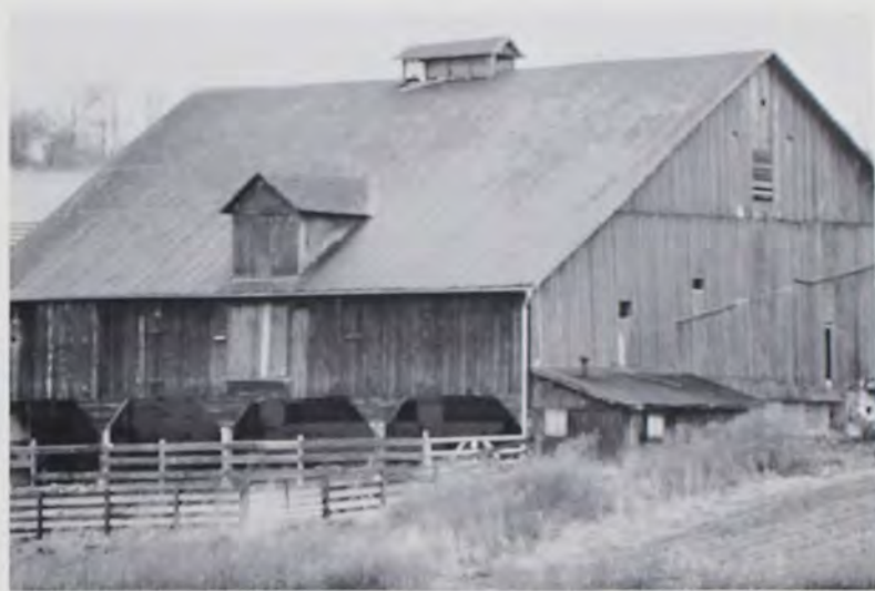
Nelson barn, Blair County, PA (c. 1860); dormer gable above supported and arcaded forebay.
