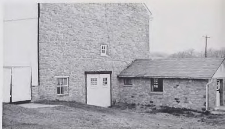
Reifsneider barn showing conversion to centered gable end stable access and central nave basement plan.
