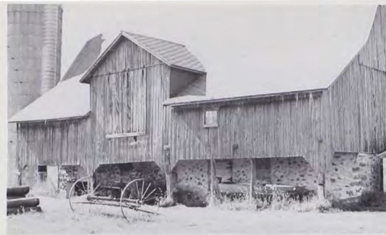
Marathon County porch (forebay) barn with supported and arcaded forebay and dormer gable.
