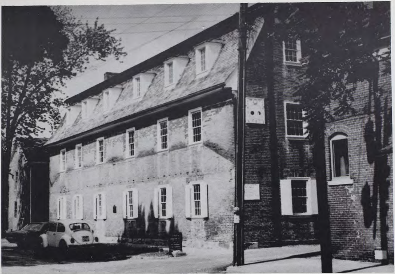
Dormitory at New Harmony, Indiana. By the early 18th Century variations of the mansard roof were common in Germany, especially in the public buildings of more than two stories where the architect wanted to emulate the classical style. The striking difference between the Harmonists' classically influenced dormitory and the medieval dormitory at Ephrata is indicative of the more sophisticated aesthetic philosophy of the Harmonist architect.
