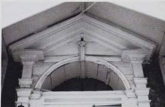
Georgian doorway of Frederick Rapp's house at Harmony, Pennsylvania. Indicates the emergence of the classical strain in Harmonist architecture. F. Rapp was the community architect and financial leader.
