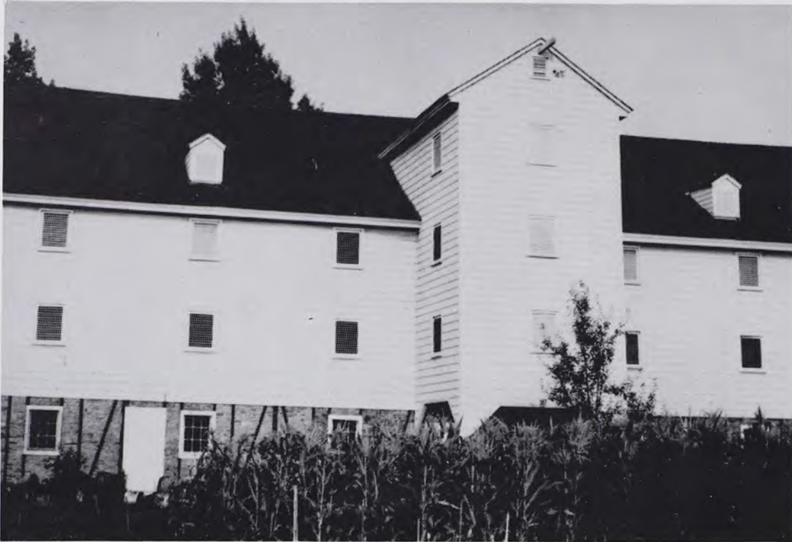
Granary at Economy. Note the half-timber first story.
