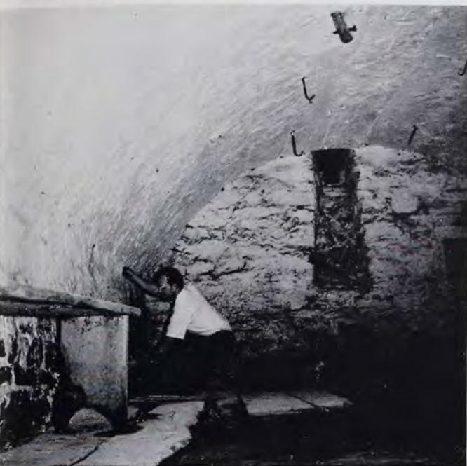
Full end-view, arched cellar. Ulrich-Steimetz Farm. Note whitewashed arch and walls, hooks on the ceiling, air vent and cooling closet.
