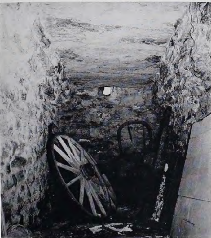
Interior view of ramp-type cellar, Royer property, Lebanon County. The interior of this one measures fifteen feet long, four and one-half feet wide, and five feet high.
