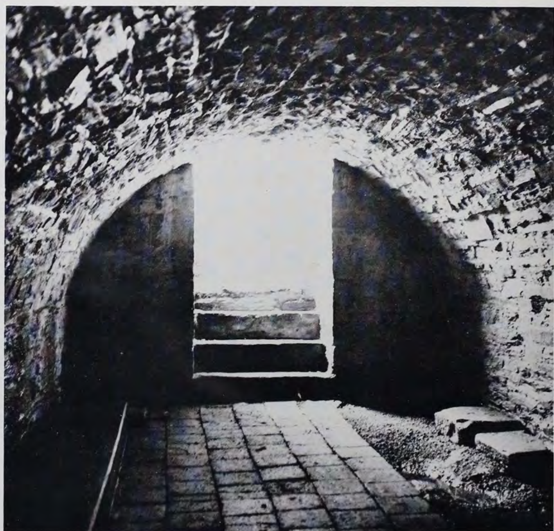
Interior of cave-cellar, Keith-Moyer homestead, Schaefferstown. Measurements: twenty feet long, nine feet wide, and six feet high. This view is on the inside looking out.
