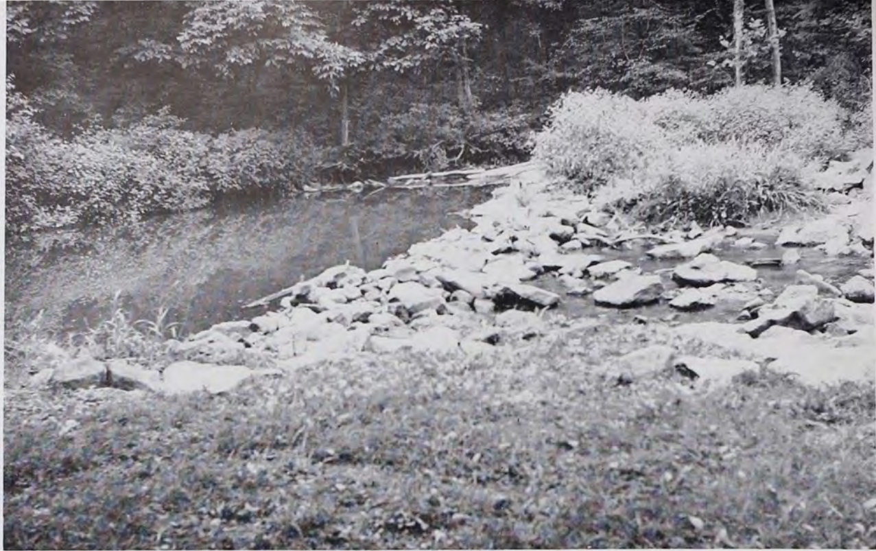
The "lower" dam, main source of water for the Denver irrigation system.
