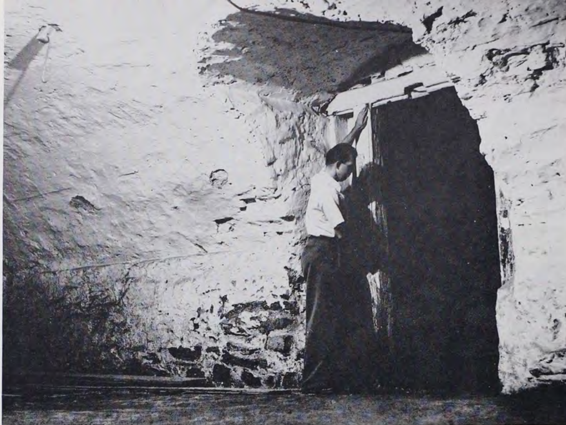
Stone-arched cellar located under the Ulrich-Steimetz farm-house north of Anville, Lebanon County. The arch is built under the original portion of the house. The cellar houses a spring, and tradition has it that it was used as a refuge during the Indian Wars of the 1750's. The door of the house itself bears the inscription:
