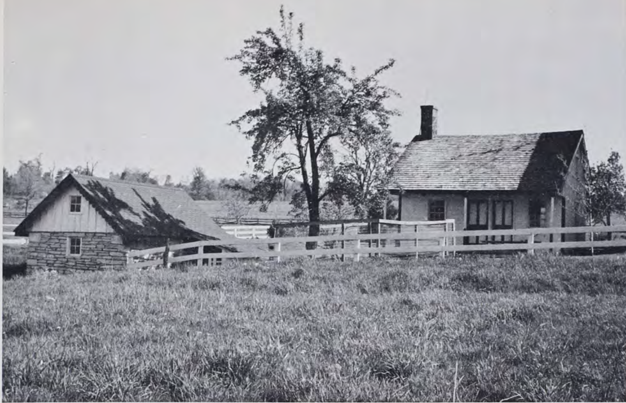
Detached Log Summer-House on James Monteith Farm near Kauffman's Church, Lebanon County, with springhouse at left. Note two front doors, for entrance to separate rooms.
