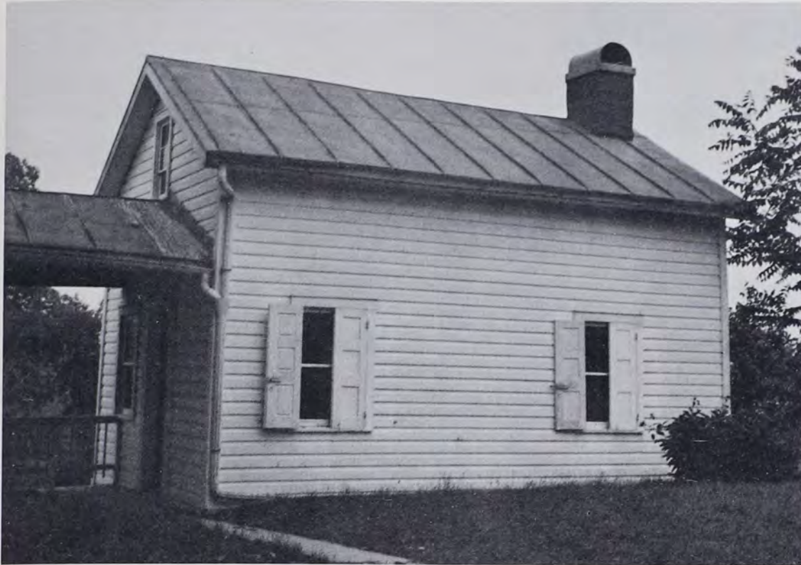
Semi-Detached Summer-House on William Siegfried Farm near Bernville, Berks County. Note breeze-way arrangement attaching summerhouse to main dwelling.
