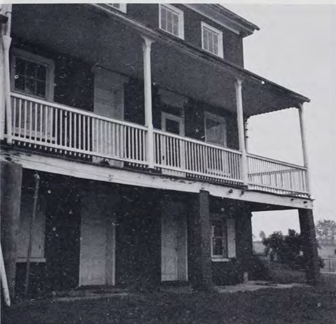
Detail of Basement Summer-Kitchen on William Siegfried Farm, near Bernville, Berks County. This is a common pattern of brick farmhouse in Pennsylvania in the 19th Century.
