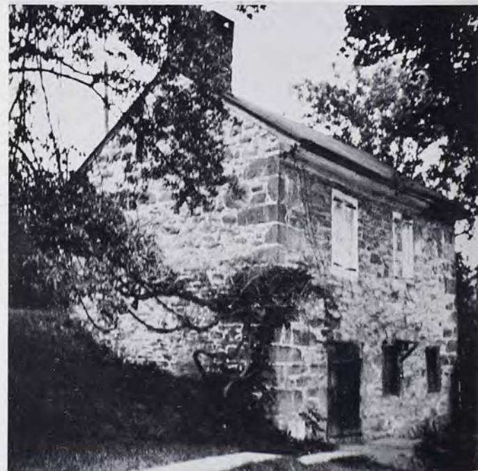
Summerhouse-Springhouse on Paul Blatt farm near Bernville, Berks County, with entrance on upper and lower levels; now used for storage.
