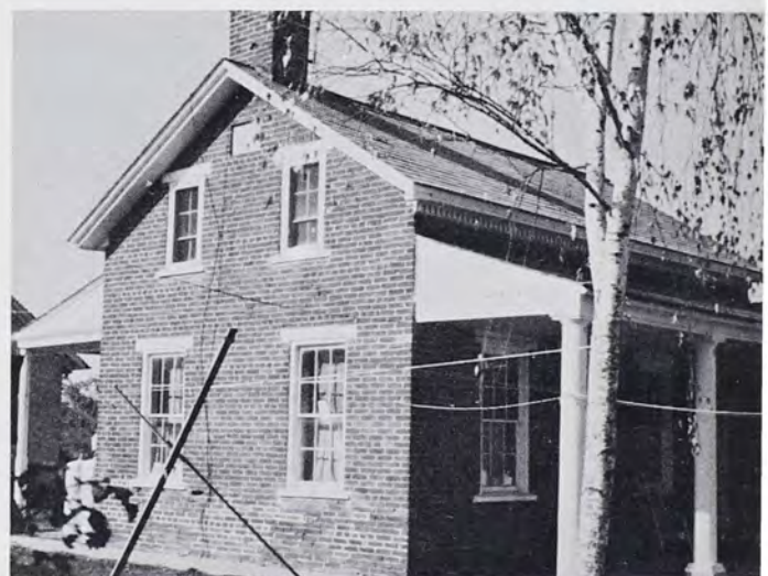
Two-story Brick Summer-House with two porches, Cyrus Winter Farm, North Annville Township, Lebanon County
