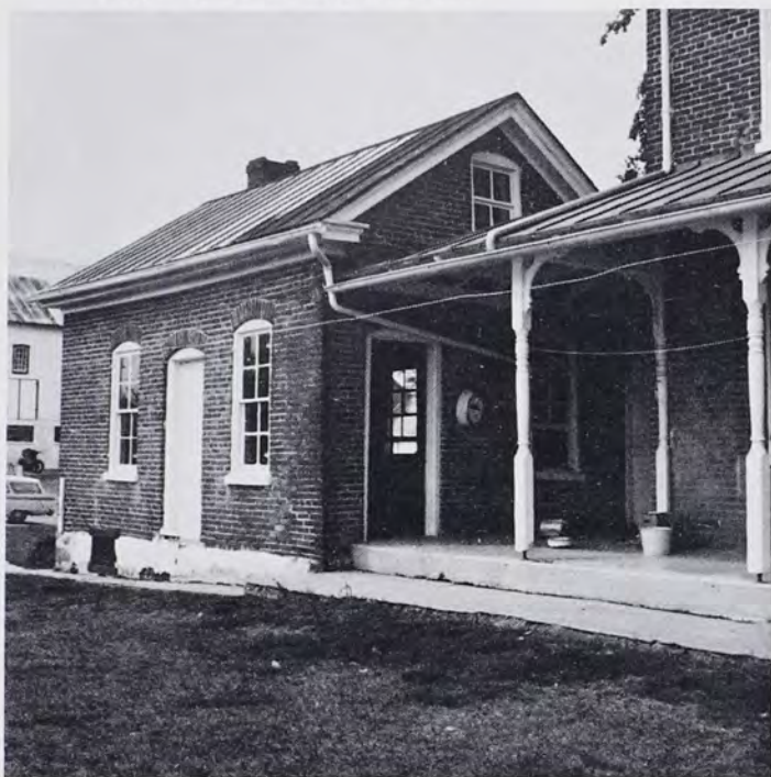
Semi-Detached Brick Summer-House on Levi Mast Farm in Oley Valley, Berks County, built 1897. Note arched windows.
