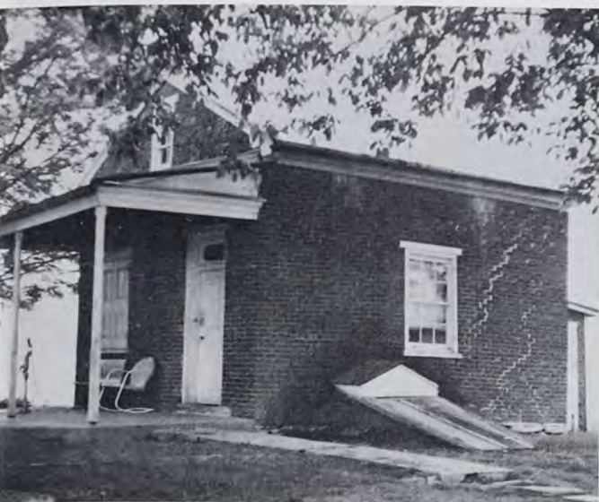
Detached Brick Summer-House on Carl Hefflinger Farm, between Myerstown and Frystown, in Berks County. Constructed of roughly hewn timber and pegged throughout, this summer-house contains an arched cellar and an attached woodshed.
