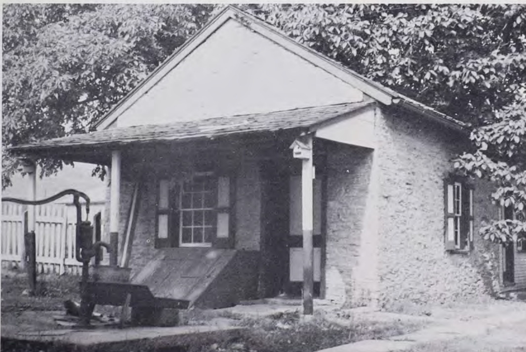
Summer-House on Arthur Kunkle Farm near Jonestown, Lebanon County. This stone and frame structure is 30 feet long and 20 feet wide and has underneath it a stone arched cellar 6½ feet high reached by 12 steps.
