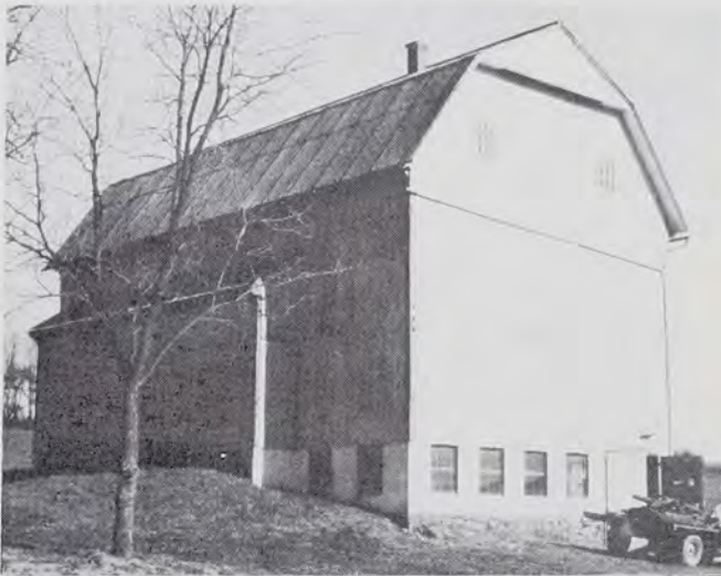
Tobacco shed with gambrel roof. Stripping room is in the gable. A gable ventilator is built out from the cornice to facilitate air movement at that level.
