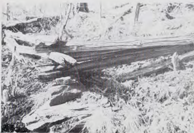
The bottom rails of a deteriorated rail fence, located east of Lynn. This fence had rock supports at the juncture of the rails.
