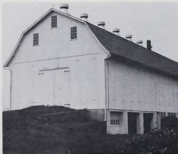
Tobacco shed with gambrel roof in Denver, Lancaster County. Stripping room is on the side of the shed next to the large doors.
