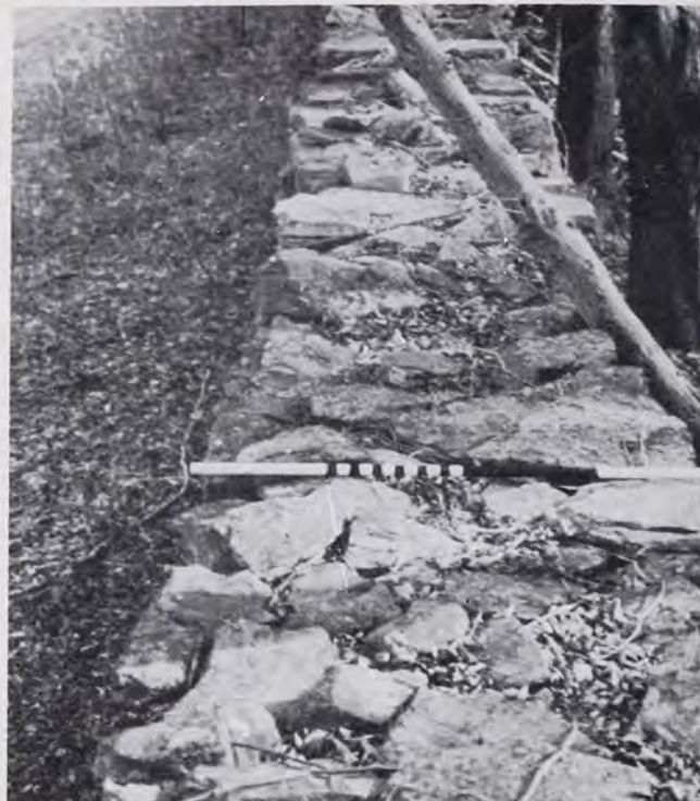
Top of stone wall on the Dietrich farm near Springville. This wall is over four feet in width at the top, with a wider base.
