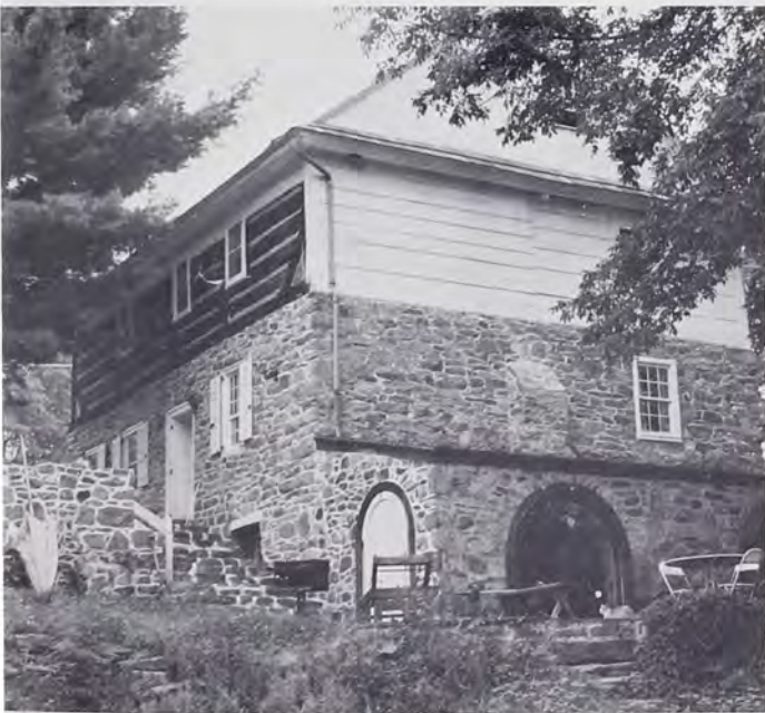
Gehman House, eastern Berks County, near Seisholtzville. Large stone and log bank house with upper and lower fireplaces on lower gable. Outside stone stairs still connect the two levels. There are several bank houses on the farmstead of this Swiss family. The stone patio with arched doors is not a part of the original house.
