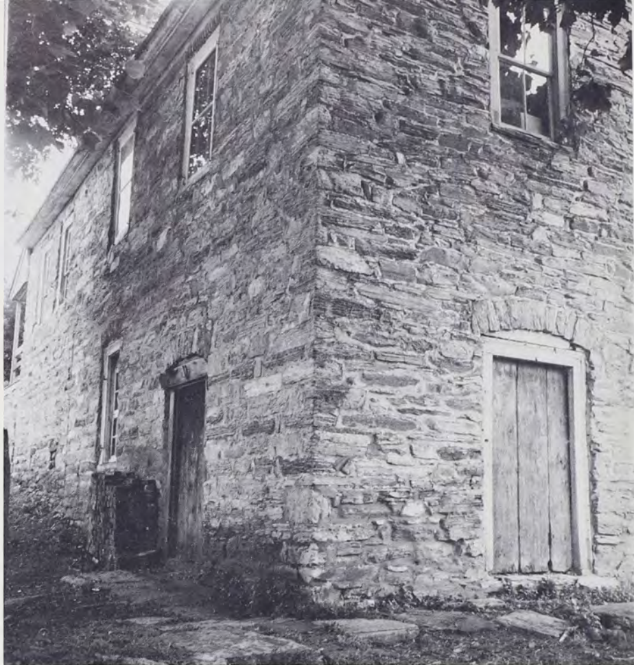
The Schaeffer house built by John Miley, circa 1736. Limestone construction with red tile roof originally, fits the Weinbauern tradition. Arched doorway on left leads to cooking fireplace, arched door in gable leads to distilling area behind fireplace.
