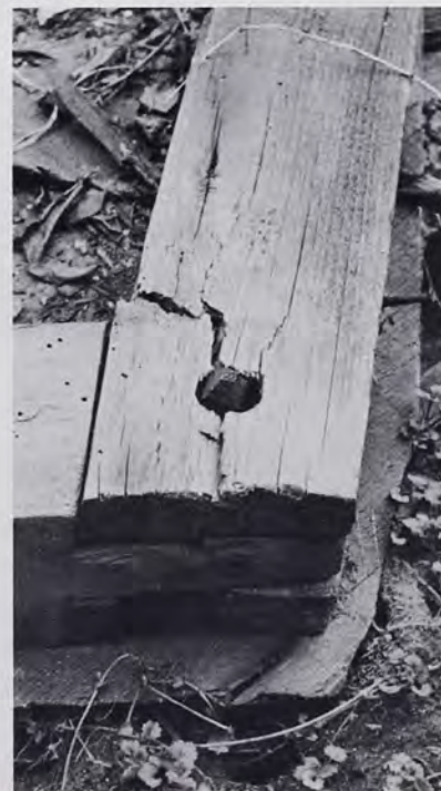
Open Mortise Rafter Joint.
