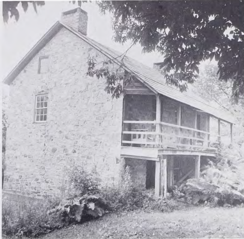
Ulrich Beitler House near Berk-Montgomery County line, fifty miles east of the Lebanon County houses. Typical stone construction with gable fireplaces. Large arch cellar in the bank (right side) with doorway near gable at lower level leading to large cooking kitchen fireplace. Spring water flows through trough along rear wall of house from upper level on right to lower level and trout pool on left, just below the house (left). Note similarity of fenestration and doorways in Beitler and Spangler Houses.
