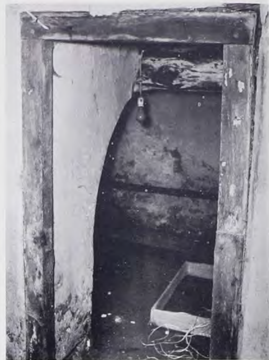
Looking into arched cellar of Beitler House. Trough at rear of this room carries spring water for cooling milk and other food.
