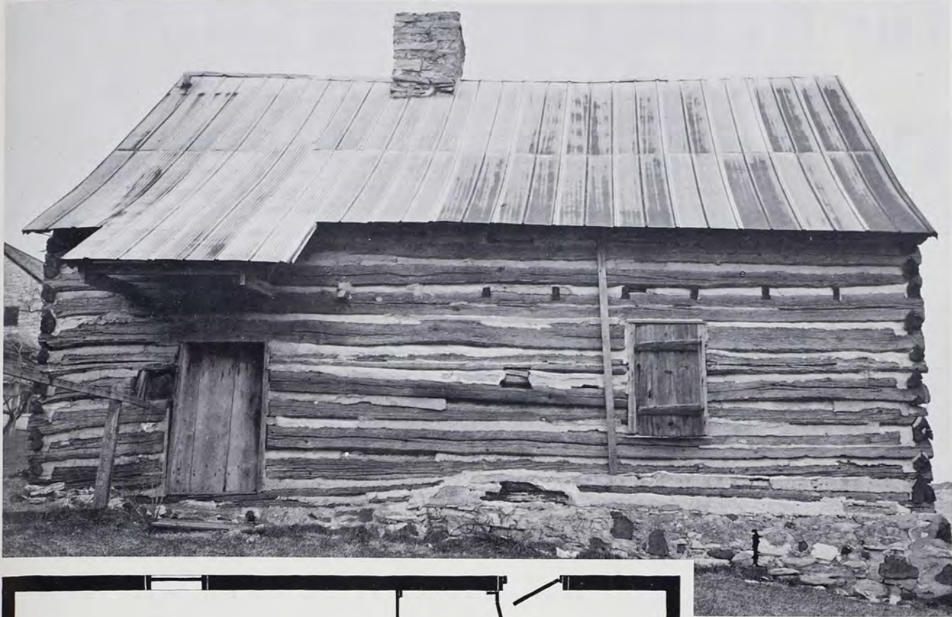
The Bertolet House. Above, Pennsylvania Historical and Museum Commission photograph of the house on its original site in the Oley Valley of Berks County. Note the tapered battens on the window shutter, the full stone chimney, and the V-notched corner-timbering. Left, Plan of the first floor redrawn from the detailed plans made by D. F. Smith of the Historical and Museum Commission staff. This is the house which Bucher in "The Continental Log House" calls "the Schneider cabin," pp. 14, 16; although he states that it has no cellar, there was a cellar under half of the house which was entered through the door next to the chimney.
