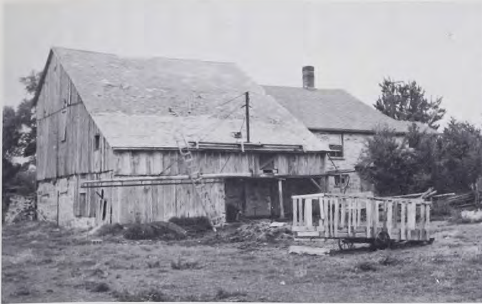
Huntsperger House-Barn Unit, St. Clemens, Ontario, Canada, a combination half-timber house with frame bank barn, built into the bank and facing South. Central fireplace with cooking area in the cellar, carries much of the spirit of the Schaeffer House in Schaefferstown, Pennsylvania. Not visible on the photograph is the front barn foundation wall of 10-inch diameter trees dug into the ground, and forming a vertical, closely fitting wall. Known as "Ständerbau" in Europe, this primitive construction is similar to the outside barricades of our early forts in America.
