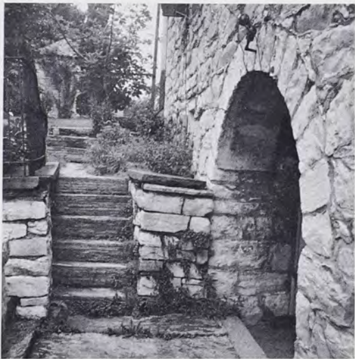
Outside stone stairway from upper level of Ley House. Inside the archway are found the ground cellar (left) and the large cooking fireplace on the right. The spring provides water in all three cellar areas.
