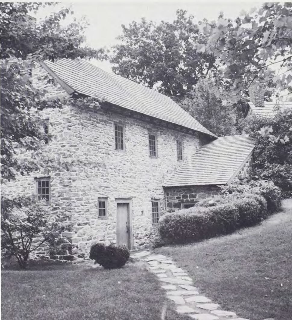
The almonry at the Ephrata Cloister, also built by John Miley, circa 1738. Large arch cellar in the bank, outside stone stairway (Freitreppe) connecting main door on upper level to cellar door on lower level near gable end.
