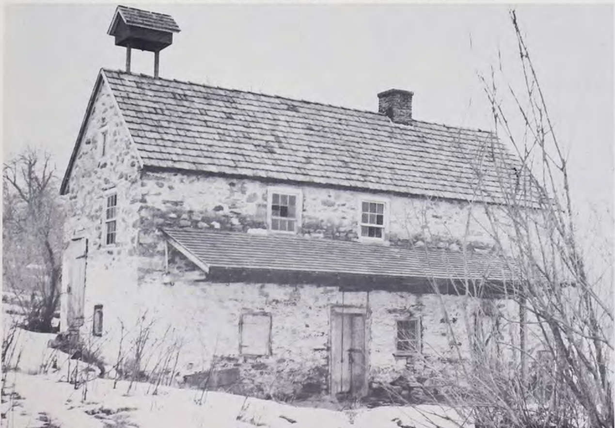
Knabb-Bieber House, Oley Valley, Berks County, Pennsylvania. Bank house type, with cooking fireplace, arch cellar and spring in lower level. "Freitreppe," the outside stone stairway to upper level located on left in photograph. Upper level has living and sleeping areas. Tile roof is traditional.
