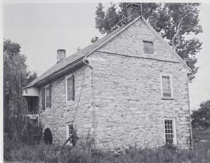
Spangler House, almost a copy of the Ley House, located 300 feet from the Ley House and built into the same steep bank along the Tulpehocken Creek. Sketches of floor plan show similarity of the Spangler and Ley Houses, except for main doorway and rooms oriented to the east in the Spangler House and to the west in the Ley House. Outside stone stairway from arch to upper level is still in use.
