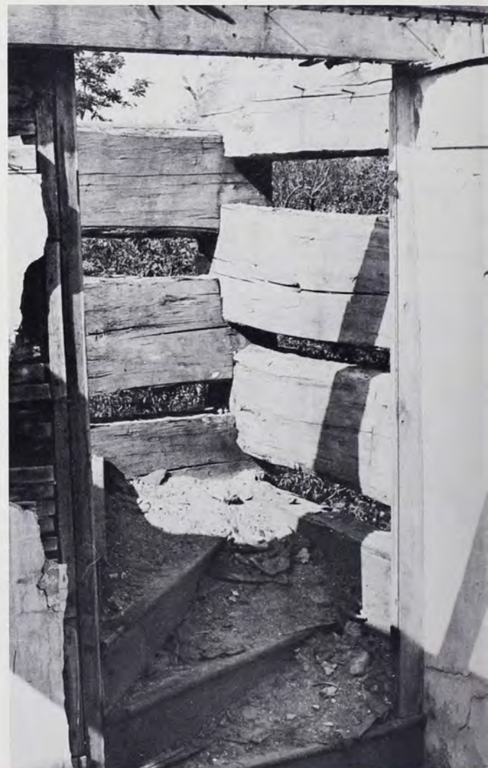
Stairway to the Loft. Note the horizontal lath of the wall, the nails driven into the logs for hanging clothes and the fact that the tops of the logs are roughly hewn.
