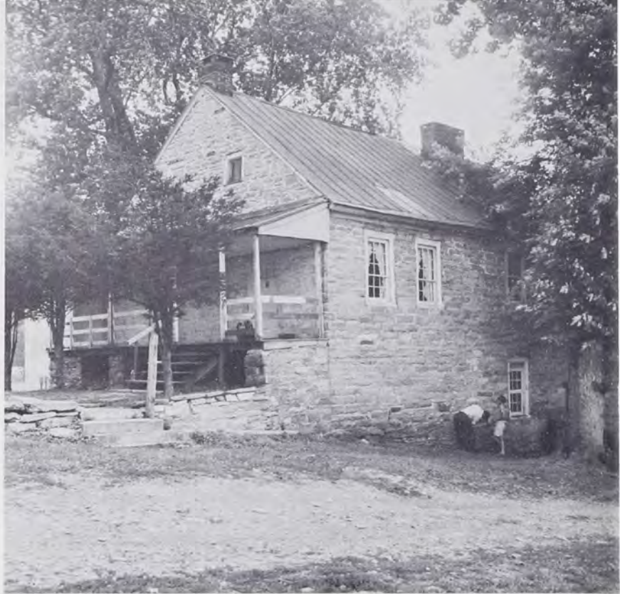
Upper level of Schaeffer House. Schaefferstown, Lebanon County, Pennsylvania. Front door is in traditional location. Solid stone wall area under two side windows marks location of large arched cellar inside.
