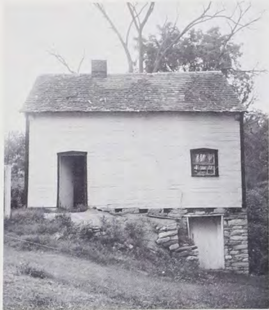
Riedt log bank-house built into a steep bank with upper and lower cooking areas and outside stone stairway connecting the two levels. Located near Stouchsburg, Lebanon County, Pennsylvania.
