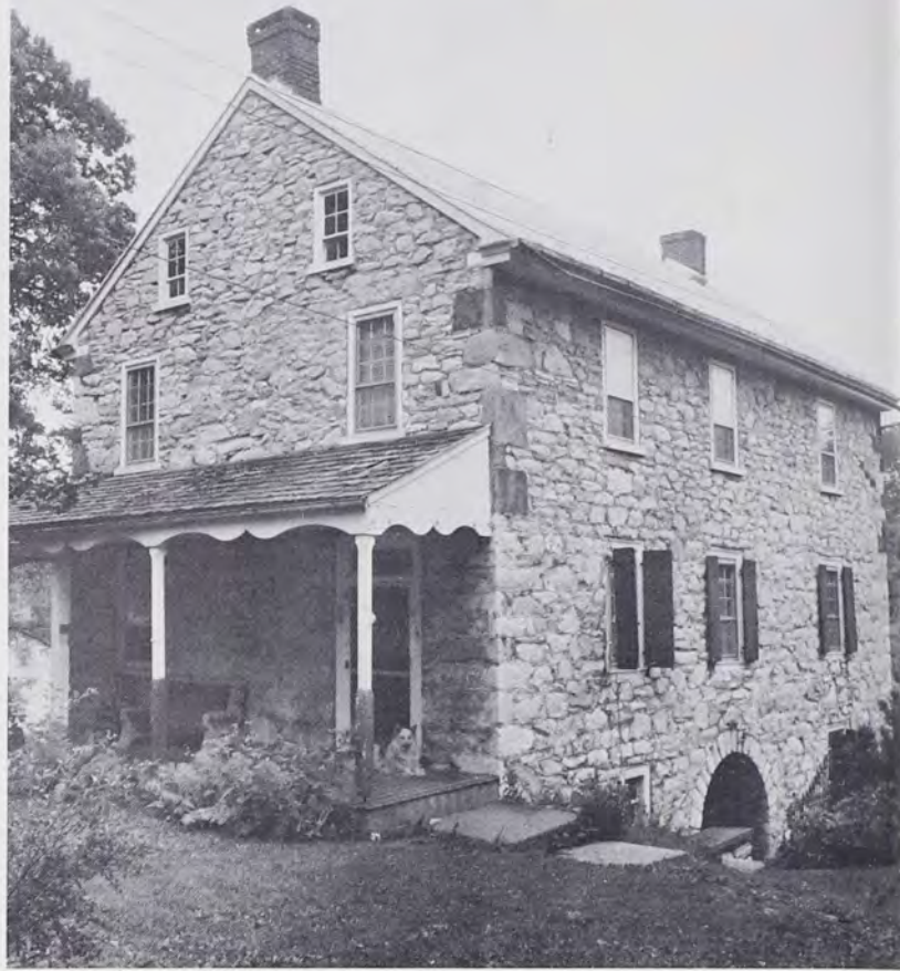
Ley House on Tulpehocken Manor, Myerstown, Lebanon County, Pennsylvania. Very similar in appearance to Schaeffer House and almonry, but with unusual arched entry way through entire width of building. Entering archway the door to the root cellar is to the left, in the bank, and the door to the large cooking kitchen fireplace is to the right, out of the bank. Large spring discharges through the root cellar and kitchen along far wall. Outside stone stairway leads from arched area to front door on upper level. Red sandstone quoins mark addition of full second story, circa 1850.
