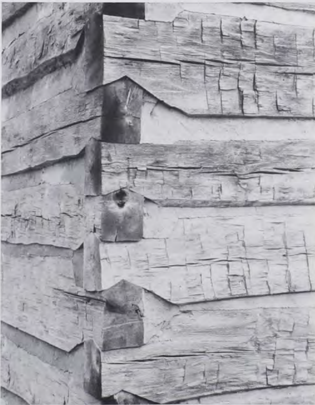
Fig. 1: Hewn, boxed V notching from Monroe County in upstate New York, now in the Genesee Country Village and Museum at Mumford. Clearly, Pennsylvania carpentry spread north by the Susquehanna and other routes to influence New York. It represents type H in Fig. 15. (Photo by T.G.J., 1984.)
