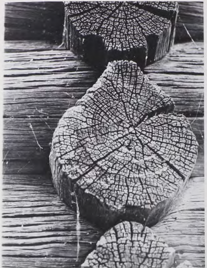
Fig. 8: Blunt-apex, crownless, round-log late medieval Norwegian V notching, in the Hallingdal, now in the Hallingdal Folkemuseum, Nesbyen, Buskerud province, Norway. It represents type C in Fig. 15. (Photo by T.G.J., 1981.)
