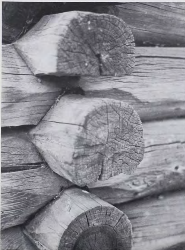
Fig. 13: Crowned, round-log, blunt-apex V notching from a mill at Ulvsjötorp near Grasmärke in the Finnskog, western Värmland province, Sweden. (Photo by T.G.J., 1985.)
