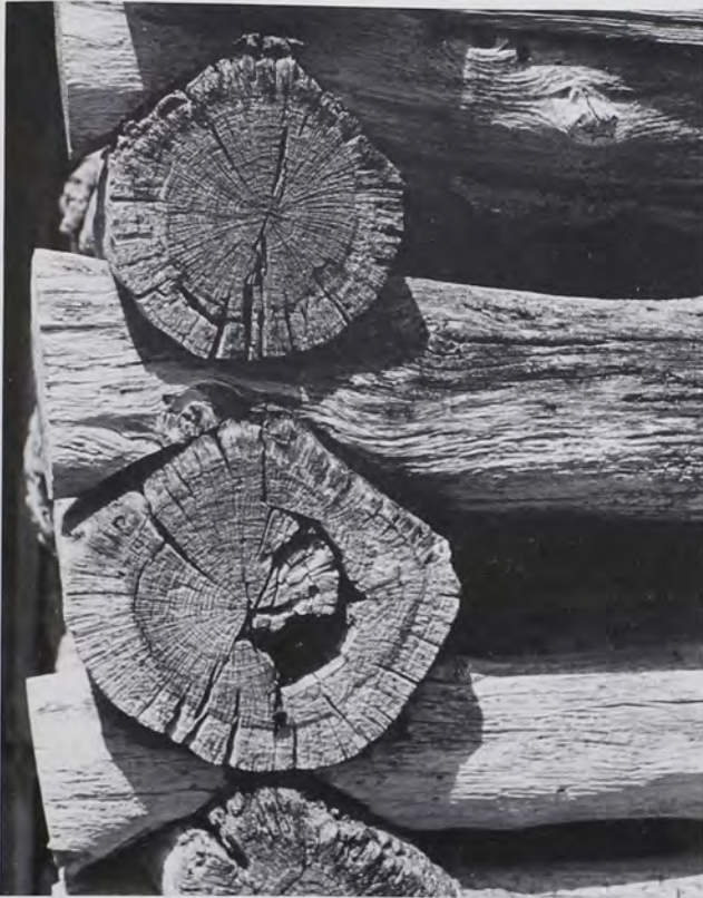
Fig. 3: Blunt-apex, round-log V notching on a barn in Cooke County, Texas. Compare it to the Norwegian structure in Fig. 8. It represents type D in Fig. 15. (Photo by T.G.J., 1981.)
