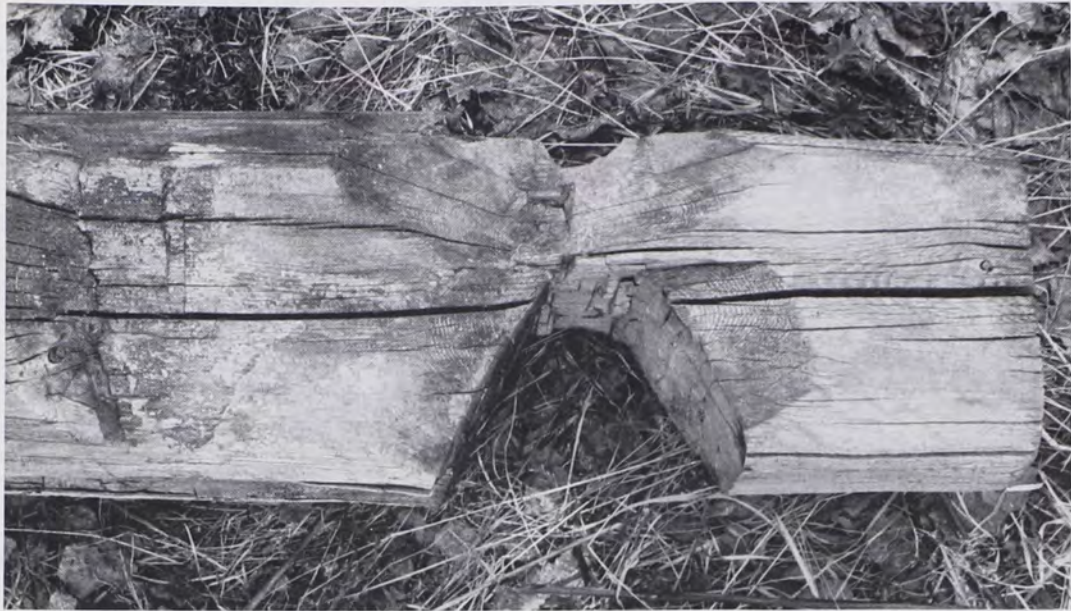
Fig. 12: Crowned, blunted V notch from a demolished building in an abandoned Finnish farmstead called Östra Tysketorpet, near Svullrya in the Finnskog,
