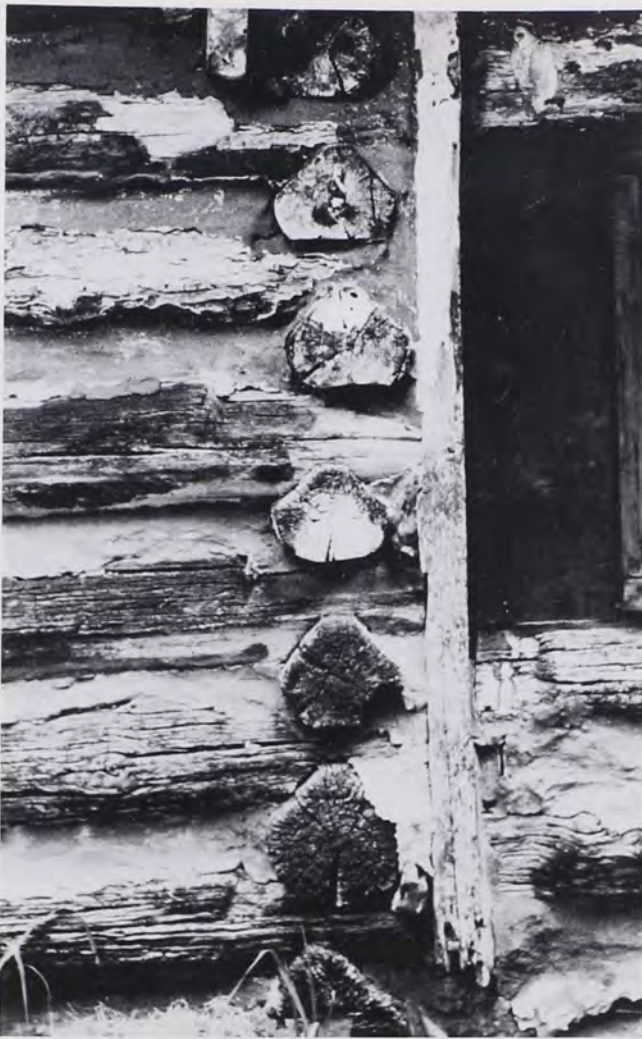
Fig. 18: Blunt-apex, round-log V notching on the Lower Swedish Cabin, Creek Road, Clifton Heights, Pennsylvania. This house firmly links Scandinavian and American V notching. (Photo by T.G.J., 1980.)
