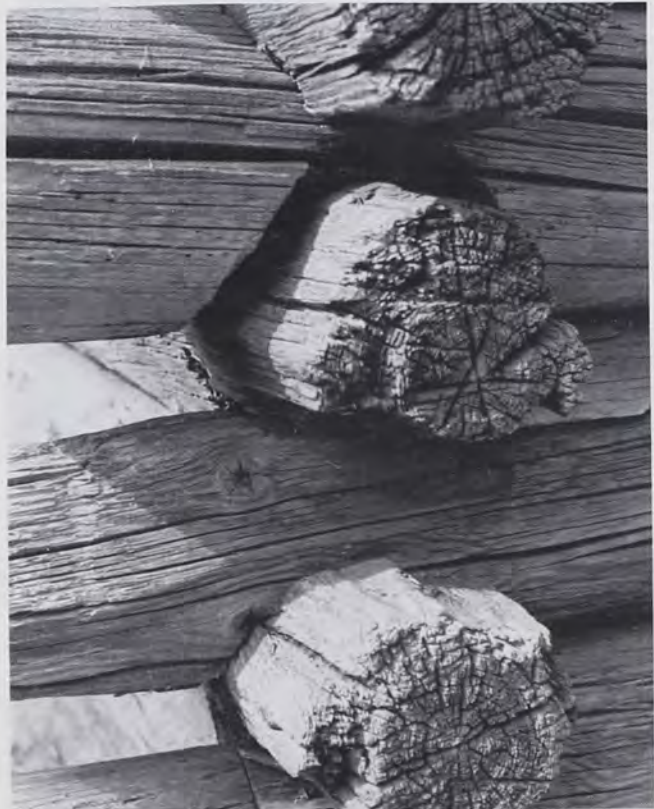
Fig. 17: Undersided saddle notching with similarity to blunt-apex V notching; near Rautalampi, Keski-Suomi (Tavastland) province, Finland, now in the Rautalampi Museo. The area around Rautalampi was the principal source region of the Finns who settled central Sweden in the 1500s and 1600s and whose descendants later colonized the Delaware Valley. (Photo by T.G.J., 1985.)
