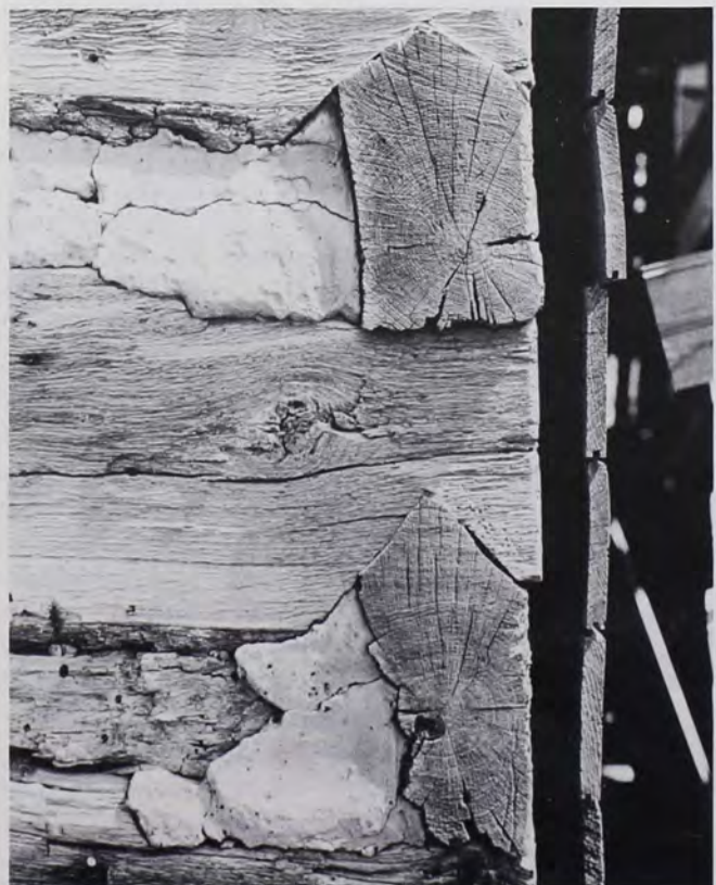
Fig. 5: Hewn, boxed V notching on thin or plank-shaped logs, on a house built about 1860 in Cooke County, Texas. (Photo by T.G.J., 1981.)
