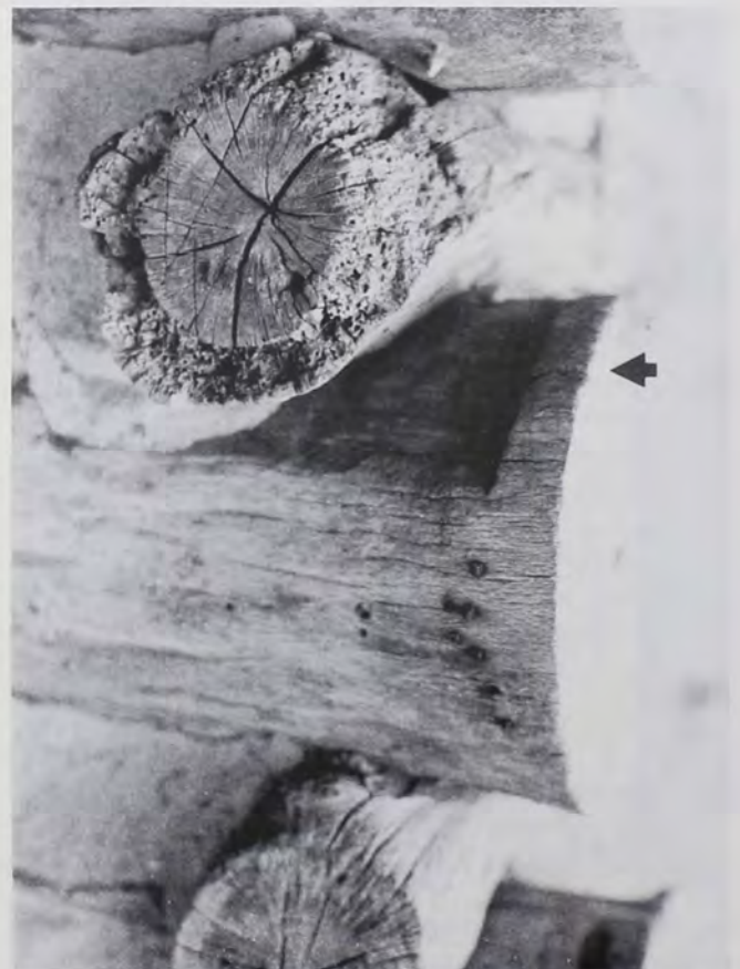
Fig. 14: Round-log V notching with surviving crown (arrow), on a house built in the middle nineteenth century in Mason County, Texas, now at the Ranching Heritage Center Museum of Texas Tech University, Lubbock. (Photo by T.G.J., 1984.)
