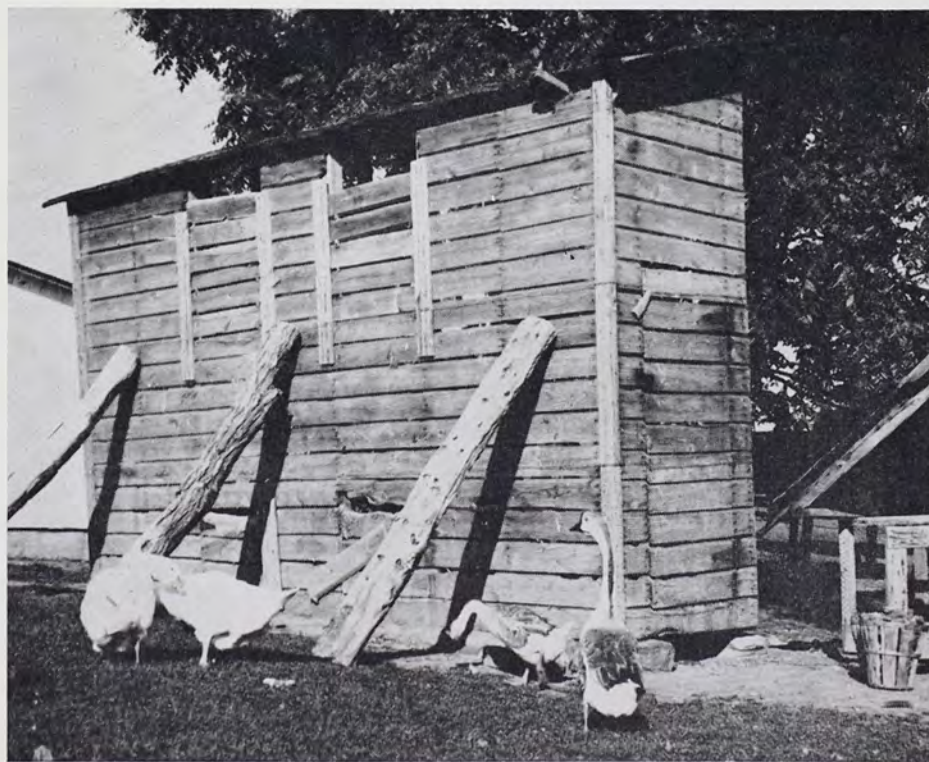
Empty corncrib, temporarily propped against heavy winds, is an auxiliary crib on author's farm, Lebanon County.
