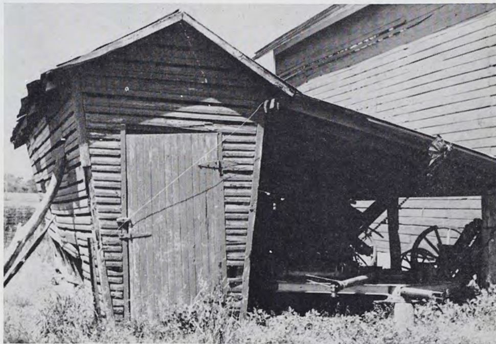
Corncrib with attached implement shed on Roy Dundore farm, Route 5, Lebanon.
