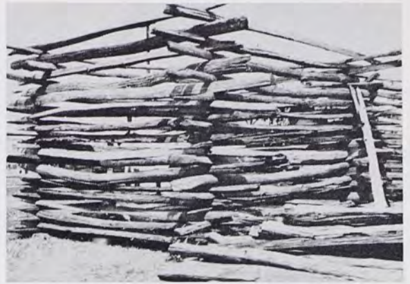
Fence-rail stacks were used in earlier days to store corn temporarily, holding many tons. Photographed at Pennsylvania Dutch Folk Festival, Kutztown.
