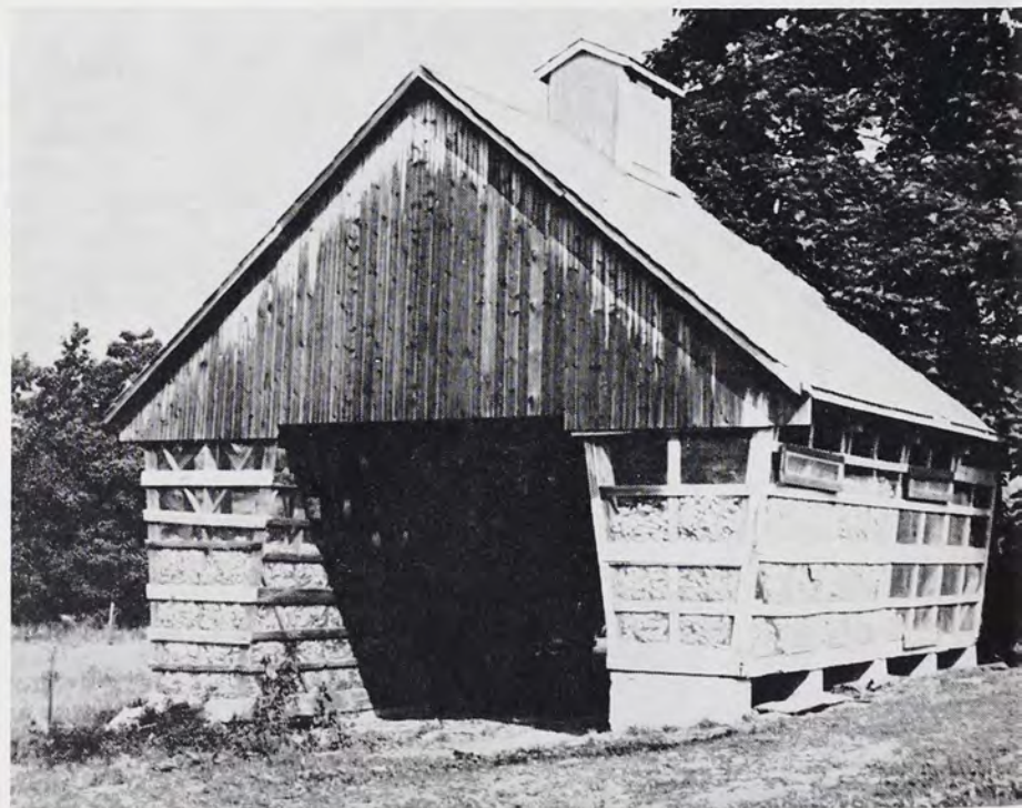
Rear-view of corn shed on property of William Reichel, Route 1, Lenhartsville, Berks County. Dimensions: 24-ft. length, 20-ft. width and 20-ft. height.
