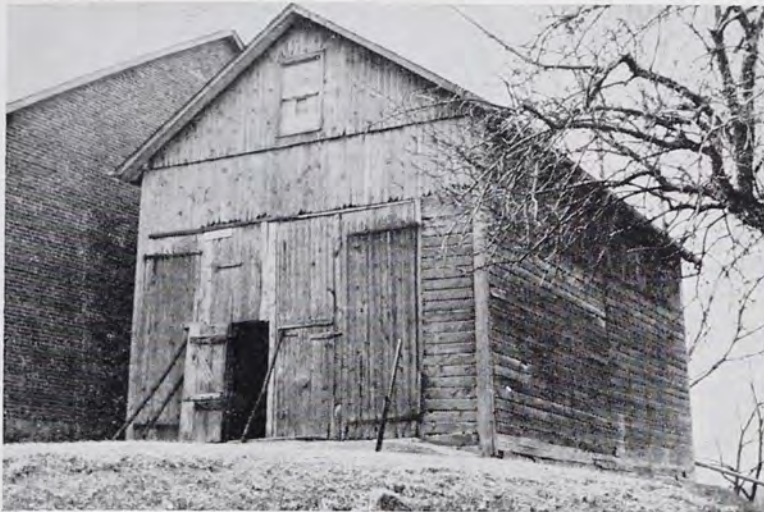
This wagon shed contains a corner crib on one side. Many sheds of this type have cribs on both sides. Note smaller doors in the large doors. Located on Paul Hartman farm, Route 1, Sheridan, Lebanon County.
