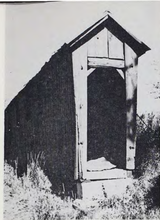
Corncrib on the property of Mrs. Alfred W. Lake, R. D. 1, Lenhartsville, Berks County. Frame of crib is constructed entirely of hand-hewn timber, pegged, with vertical slats and side openings.
