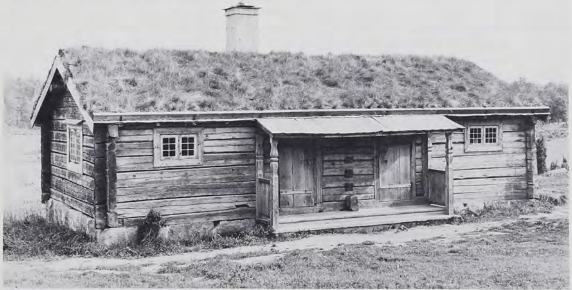
Fig. 15: The log saddlebag house, or stuga av celltyp, of central Sweden, at the Vallby open-air museum (see Fig. 2C). (Photo courtesy Nordiska Museet, Stockholm, no. 190.B.ak.)
