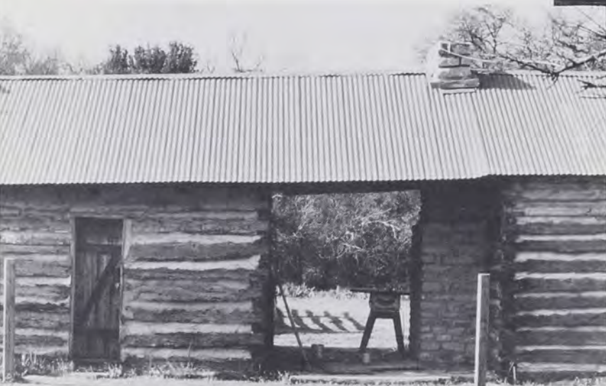
Fig. 17: Double-pen log house displaying traits of both the dogtrot and saddlebag plans, located in the outdoor museum at Stephenville, Erath County, Tex. In common with the Mortonson house (Fig. 16), this structure suggests the kinship of the two plans. (Photo by T.G.J., 1992)
