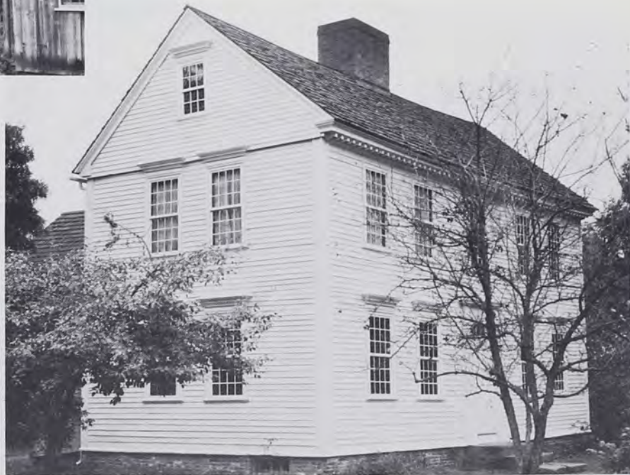
Fig. 11: The widespread Yankee colonial two-story timber-frame saddlebag I house. This is the second Wells-Thorn house in Old Deerfield, Mass., and dates to 1725. It has two full-sized rooms on each floor. Note the placement of the chimney largely behind the roof ridge. (Photo by T.G.J., 1992)
