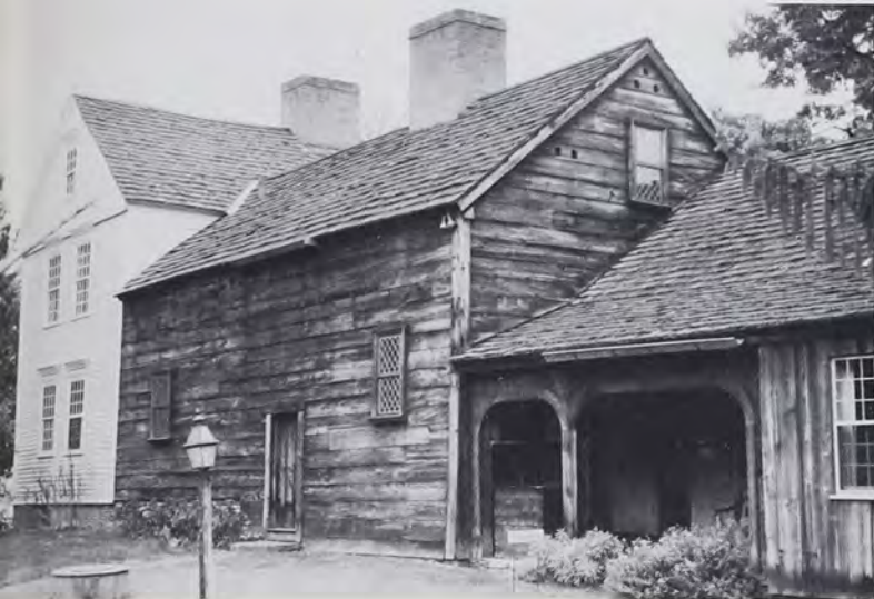
Fig. 10: The prototypical one-and-one-half story Yankee timber-frame saddlebag, or “hall-and-parlor,” house of colonial New England. This is the original Wells-Thorn house, built in 1717 and located in Old Deerfield, Mass. It was later demoted to the status of kitchen, when the house was enlarged. (Photo by T.G.J., 1992)
