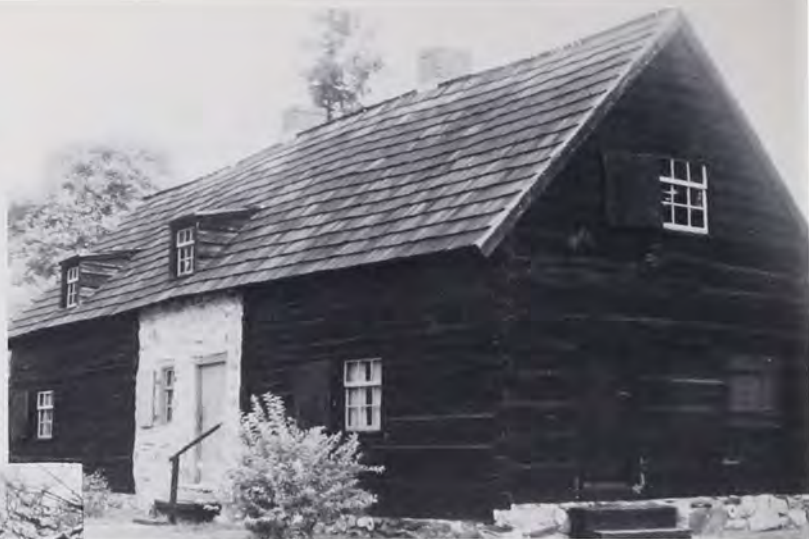
Fig. 16: Mortonson house, Prospect Park, Pa., built in the 1740s by a family of Finnish ancestry rooted in the old colony of New Sweden. Originally the passage between the two log pens was open, as a "dogtrot." The Fenno-Scandian custom of placing two fireplaces adjacent to the passageway strongly suggests a genetic link between dogtrot and saddlebag plans. (Photo by T.G.J., 1980)
