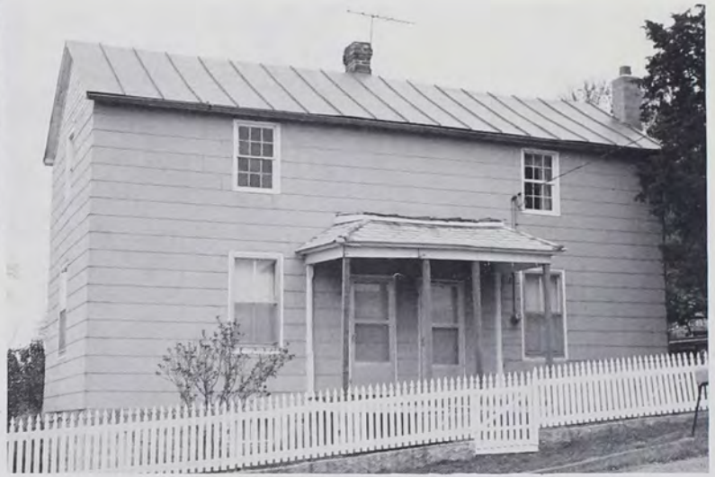
Fig. 6: Saddlebag I-house of frame construction, Rich Fountain, Osage Co., Mo. (Photo by T.G.J., 1990)
