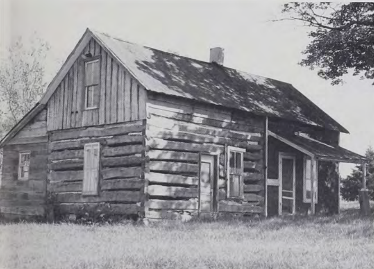
Fig. 7: Saddlebag consisting of log and frame pens, Boone Co., Mo. Logs are V-notched. (Photo by T.G.J., 1990)
