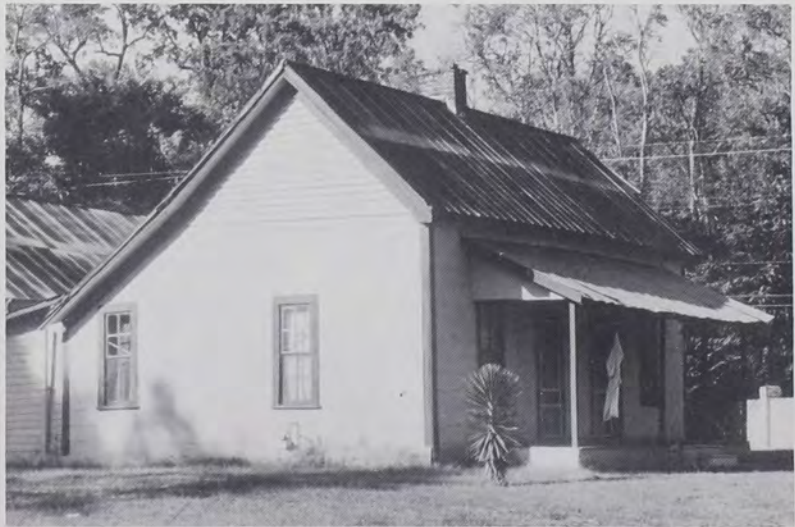
Fig. 8: Frame saddlebag with stove and flue instead of hearth and chimney. This house is in the lowland southern tradition and stands in the African American neighborhood of Nacogdoches, Tex. (Photo by T.G.J., 1991)
