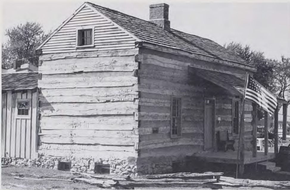
Fig. 3: Log House Museum, Lexington, Mo. (see Fig. 2F), a saddlebag with one front door and a single span of logs across the long dimension.
