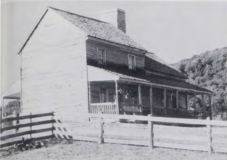
Fig. 5: Asymmetrical saddlebag house, with broken roof ridge line, combining 1 1/2- and 2-story pens, Botetourt Co., Va., now at the Museum of American Frontier Culture, Staunton, Va. Logs are V-notched. (Photo by T.G.J., 1991)
