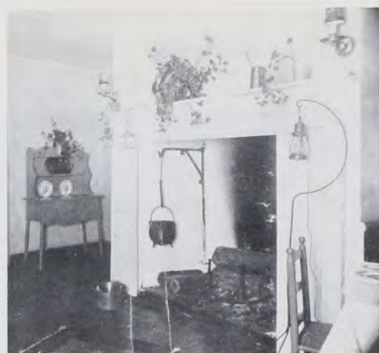
Interior view, Manor House, Croasdale River Farm.
