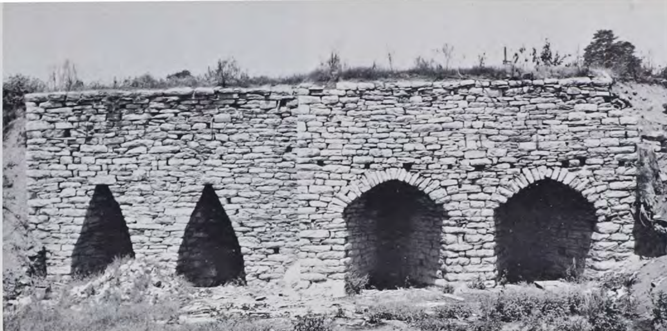
Multiple limekilns located on farm of Leroy O. Schoener, near Long's Church. Dimensions: overall length 51 feet, tapered kilns 22½ feet, height 15 feet, oval kilns 28½ feet. Tapered openings: 6 feet wide, 9 feet high; oval openings: 9 feet wide, 9 feet high. 3½' by 6' by 3½' by 6' by 7' by 9' by 3½' by 9' by 3½'. Photograph taken 1965, after front roof structure and undergrowth was removed. Multiple structures such as these were built primarily for commercial lime production.
