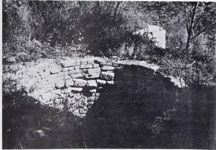
View into shaft of one of the kilns located on Leroy Schoener farm between Myerstown and Stouchsburg, Berks County. Dimensions of shaft: diameter approximately 12 feet, depth approximately 15 feet. Note deterioration of firebrick lining. Photo taken 1962.
