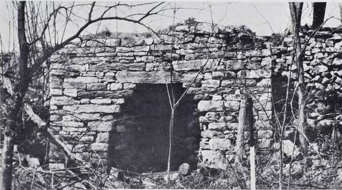
Front view of limekiln near Buffalo Springs, Lebanon County. Note how stones are corbelled to support large flat stone lintel over main opening. Stone wall on right built to support roadway in rear (1963).
