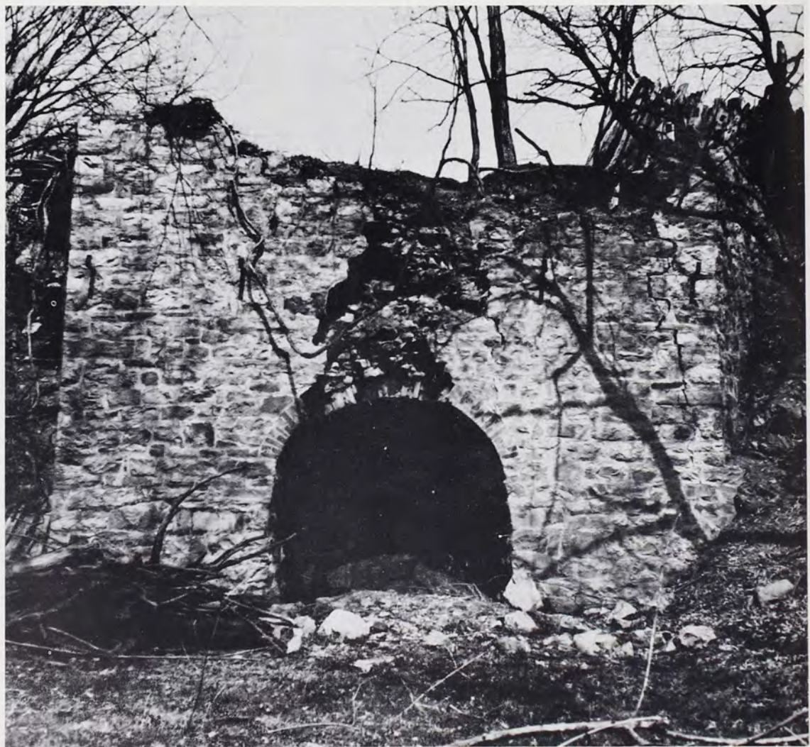
Beautifully proportioned arched main opening of limekiln located on farm of Alexander Bamberger on the Lebanon-Cornwall road. Dimensions of arched opening: length 8', width 8'. Photo taken 1962.
