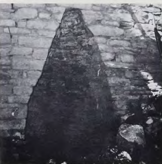
Closeup view of tapered opening in multiple kilns on Schoener farm. Note smaller or inside opening leading to shaft—outlined in white. Dimensions: 9 feet high, 3 feet to beginning of arch, one foot across top of arch, 6 feet wide at bottom. Inside opening: one foot high and 16 inches wide. Photo taken 1962.
