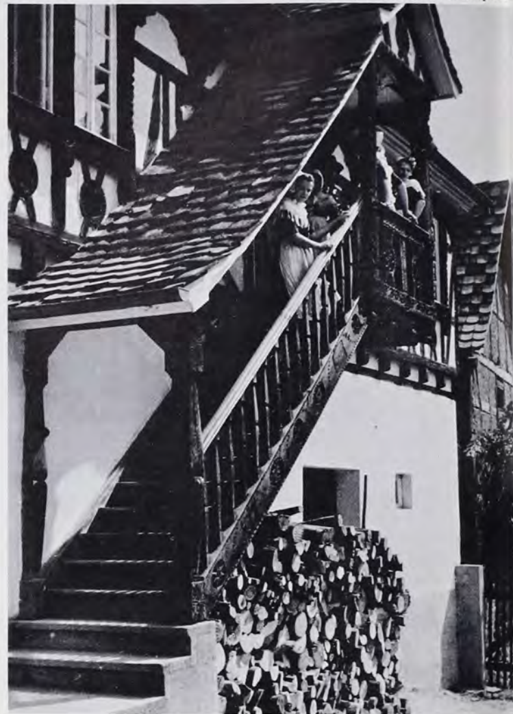
Tile-roofed stairway to ornate second-floor landing, Dörrenbach on the Weinstrasse.
