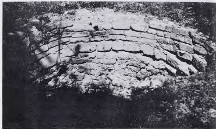
Another view of shaft opening on Schoener kilns. Note residue from lime-burning still clinging to sides of shaft. Photo taken 1962.
