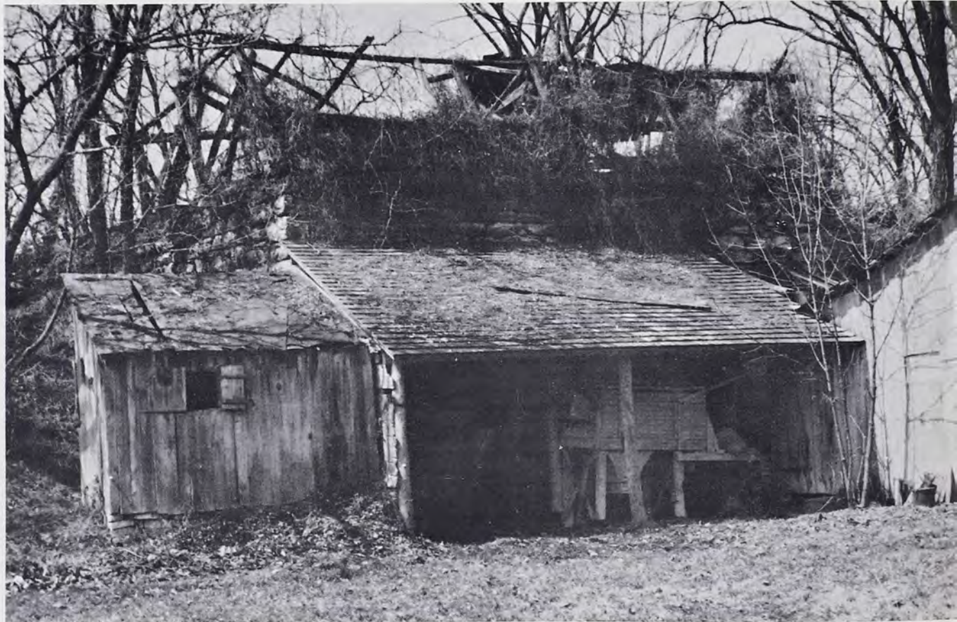
Double limekiln and attached shed roof and storage sheds, located on farm of Raymond J. Emerich near Harpers, Lebanon County. Shed on right used to house equipment and wagon for hauling limestone from nearby quarry-hole. Shed on left used to store lime. Note lime separator used to separate lime after it had been slacked, operated with gasoline engine. Note at top of photograph remains of roof structure built over shaft openings. Photo taken 1962.
