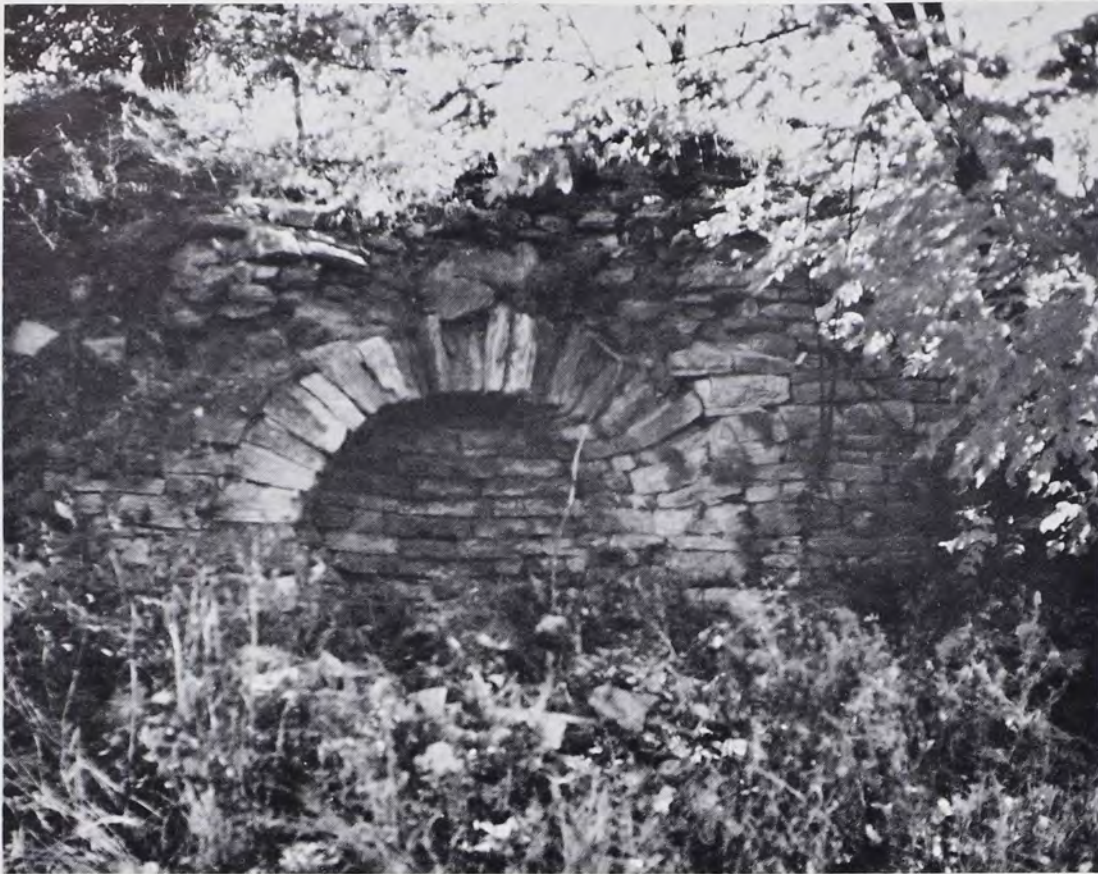
Beautifully proportioned arched main opening of limekiln located on farm of Alexander Bamberger on the Lebanon-Cornwall road. Dimensions of arched opening: length 8', width 8'. Photo taken 1962.
