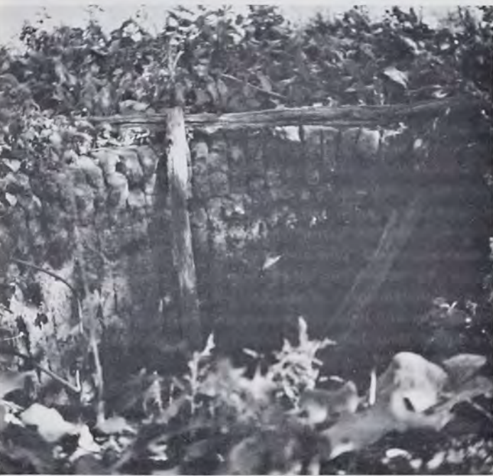
Looking into shaft of limekiln on the Elwood Houser farm. Note vertical position of firebrick in lining of shaft (1963).
