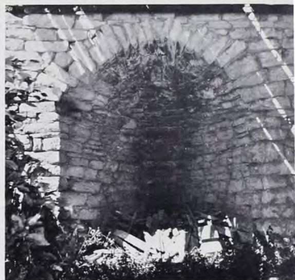
Closeup view of one main oval-arched opening in multiple kilns on Schoener farm. Note smaller or inside opening leading into shaft (partly hidden with timber). Dimensions: 9 feet high, six feet to beginning of arch, 6 feet wide; smaller opening one foot by one foot. Photo taken 1962.
