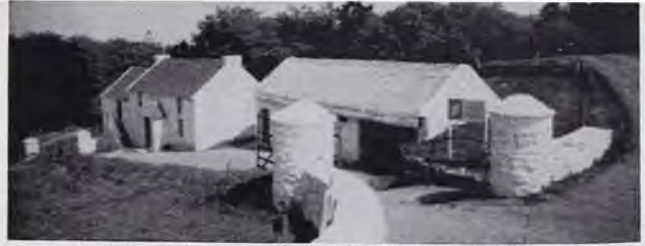
Ulster hill farm from Cushendall, County Antrim, as reconstructed at the Ulster Folk Museum in 1965. The dwelling has been rebuilt in the developed two-story form it assumed around 1900. Following the Land Acts at the end of the 19th Century by which many tenant farmers acquired ownership of their holdings, the dwelling house was raised from its original single-story form and had a slate roof applied in place of the original thatch. The detached (upper) suite of outhouses has had its original thatched roof reinstated. Note the heavy round gate pillars – a feature of Ulster farms particularly in Counties Antrim and Down.
