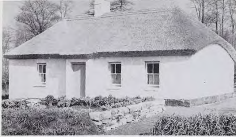
Farmhouse from south-west Ulster (County Fermanagh) showing in the centrally-placed hearth and hipped thatch, two features which distinguish it from the gable hearth, two-sided roofs of the majority of traditional Ulster houses.
