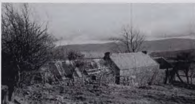
Ulster hill farm, near Cushendall, County Antrim, showing the way in which the dwelling and outhouses in rural Ulster farms are often built at right angles to the slope of the ground.
