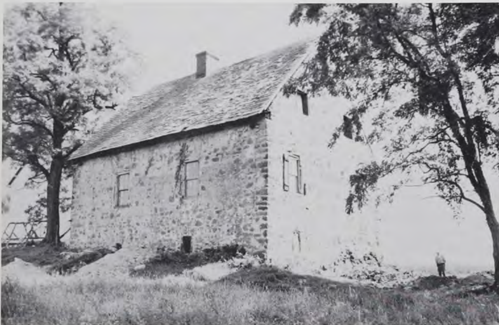
Plate 3 View of rear of Herr House with two stone-framed casement windows at ground level clearly shown. These open into the root cellar. Excavations at these points were made to expose the foundation and bedrock on which the house is built.
