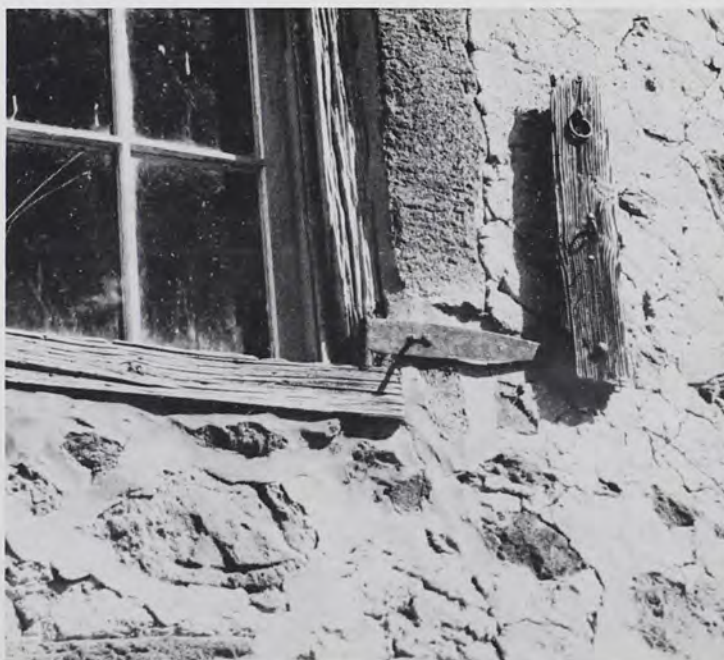
Plate 12 A view of the front side window on the Herr House with remains of a shutter. Note that the original stone frame is in place with wooden frame set into it.
