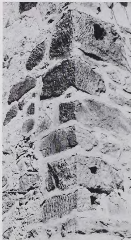
Plate 13 A view of the south corner of the Herr House with its finely dressed limestone quoins. Note the holes on the upper stone; these may have been used to hold supports for a pent roof. The lower ones may have been used to support a grape arbor.
