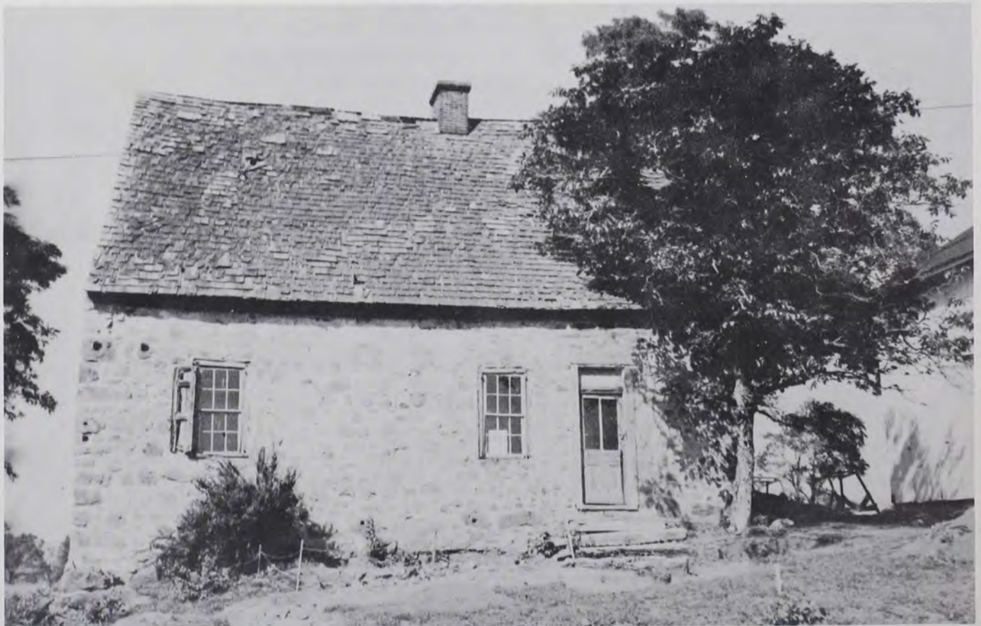
Plate 1 Front view of the Hans Herr House. Note the offset door, wood-framed windows and door, high pitched roof, central chimney, and holes in corners just left of and above south window.
