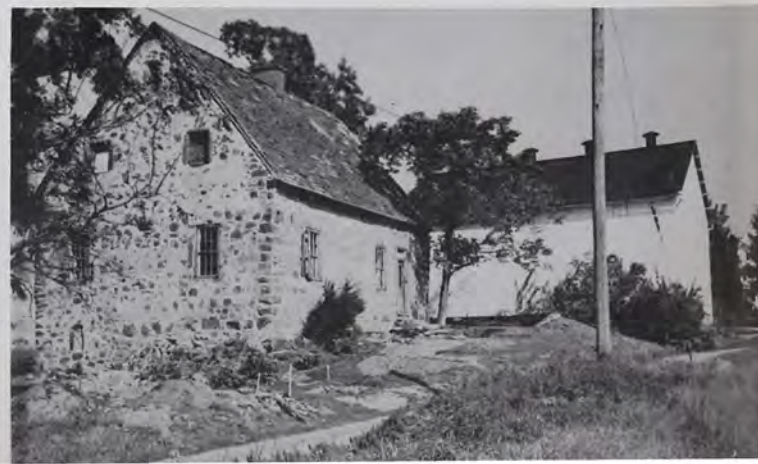
Plate 2 View of Herr House from south showing southwest gable and relation of house to tobacco barn and driveway. Finely dressed cornering can be seen as well as stone-framed casement windows in southwest gable on the second and third levels. A small stone-framed window can be seen at lower left that leads into root cellar.
