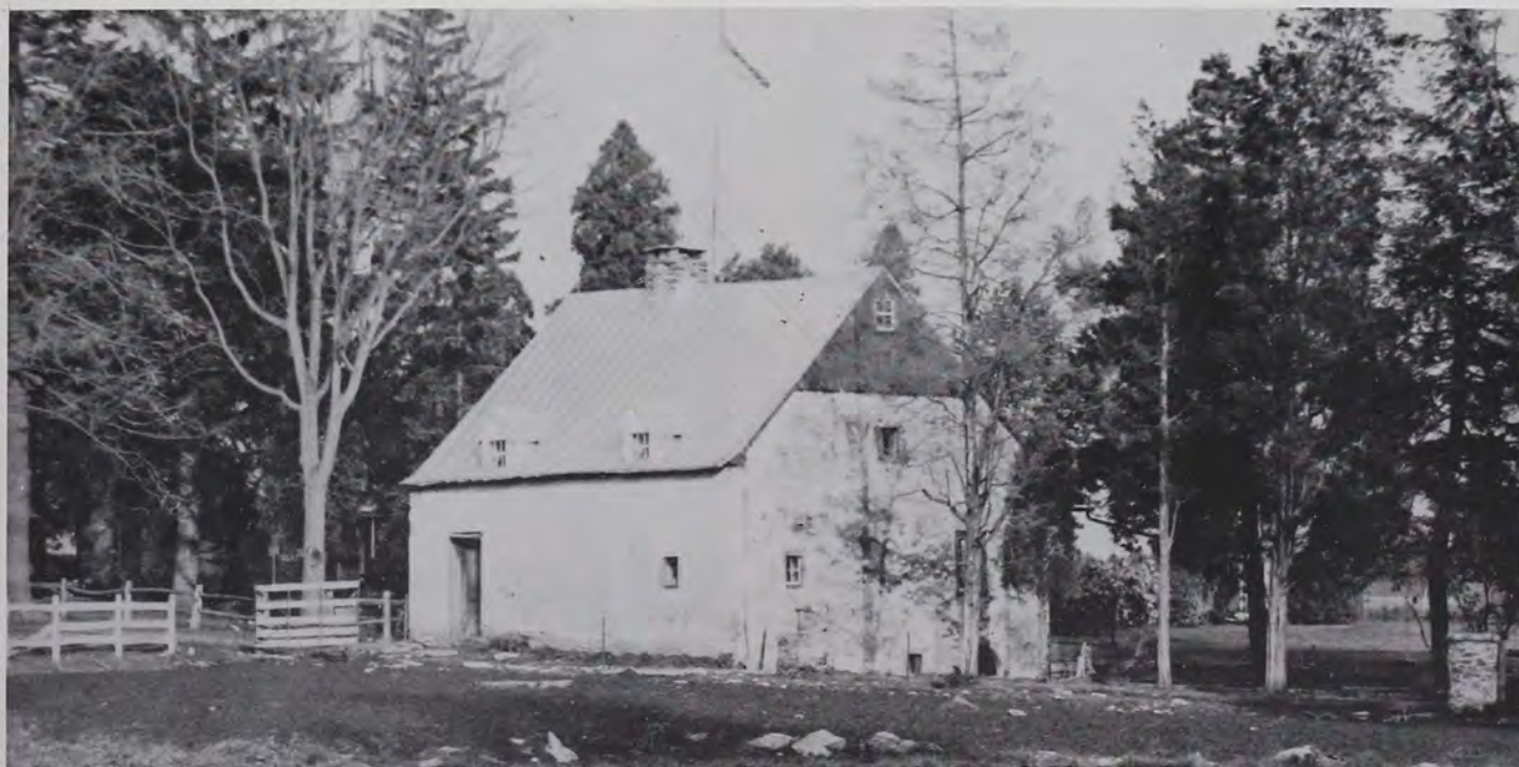
Plate 16 A view of the rear of the Zeller House with its offset rear door, stone-framed casement windows, vertical sheathing on the gable and a slight “kick” of the roof.
