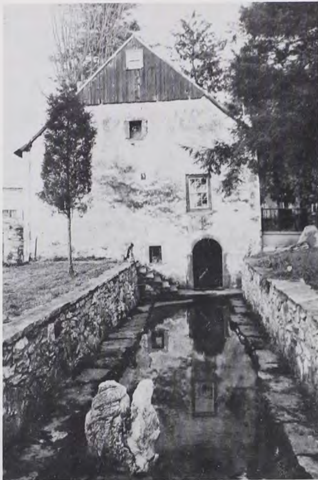
Plate 17 A view of the south gable of the Zeller House with its spring room and stream running from that room. The window above the door is not part of the original building but the window to the left is. The stone walls on either side of the stream were added during the 1940's. Note also the vertical sheathing and nicely finished door frame.
