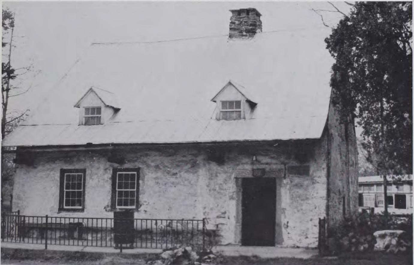
Plate 15 A front view of the Zeller House. Several features of the house can be seen, including the offset front door with inscription, central chimney, dormers, wood-framed windows, high pitched roof, and the "kick" of the roof. A cement porch, added in the 1940's, is also shown with an iron fence around it.
