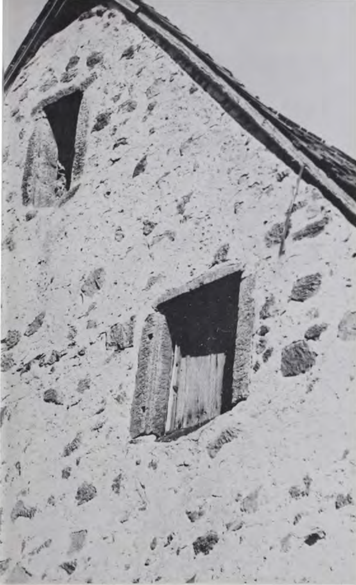
Plate 11 Stone-framed casement windows on the south gable of the Herr House are shown in this photograph. Rabbets for a shutter can be seen in the lower window.
