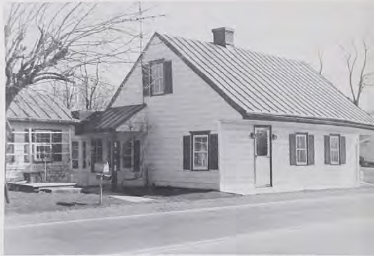
Toll House. Near Middletown, Pa.
