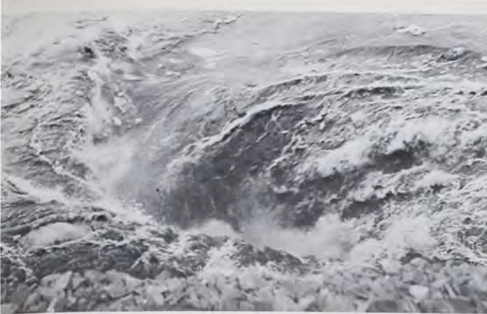
The Susquehanna River swirling into the collapsed Knox mine in January 1959 ended the era of deep mining in the Wyoming Valley.
