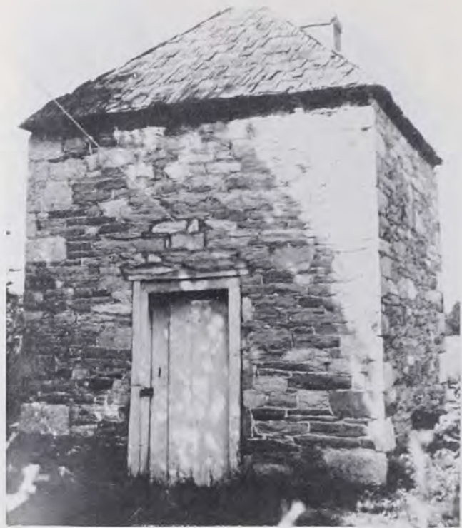
Early stone smokehouse in Pennsylvania's Lebanon Valley.
