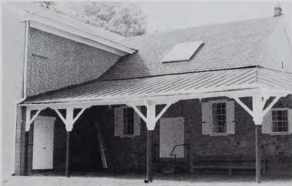
Side Porch at West Chester (1974).
