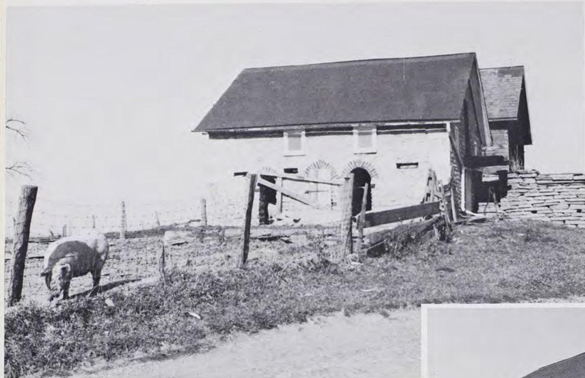
Side-frontal view of early stone pigsty (left) with beautifully proportioned brick-arched entrances, and side view (below), located on the Ulysses Mays Farm, south of Lebanon, Pennsylvania.
