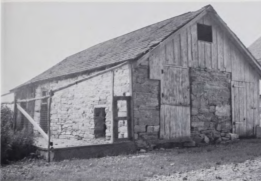
Combination masonry and frame pigsty on the old Schaeffer farmstead, now the property of Historic Schaefferstown, Inc.
