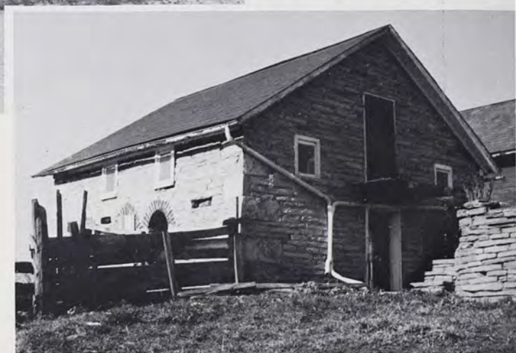
Side-frontal view of early stone pigsty (left) with beautifully proportioned brick-arched entrances, and side view (below), located on the Ulysses Mays Farm, south of Lebanon, Pennsylvania.
