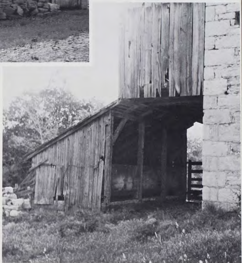
An unusual pigsty arrangement, being attached to the front of the forebay of a bank barn on the farm of Victor Lehman, Marion, Franklin County, Pennsylvania.
