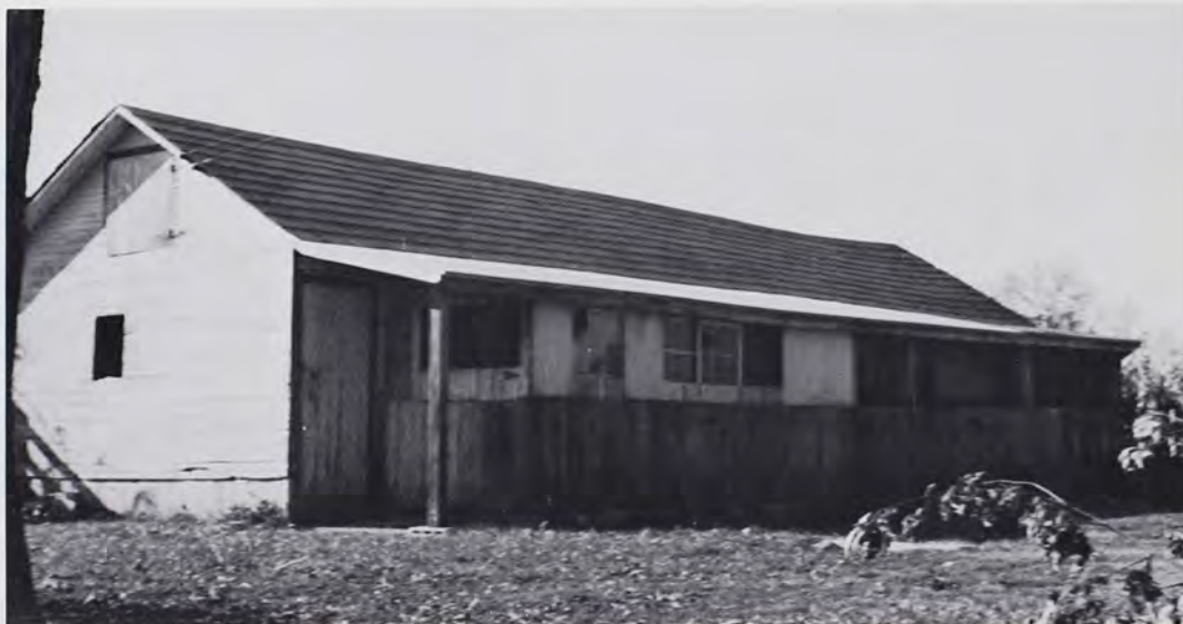
This large pigsty of frame construction with loft stands on the farm of Bertha M. Kline, Myerstown.
