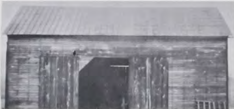
Front of barn as it appeared in 1920, with one of the huge sliding doors open. An earthen ramp led hay and wagons up to the barn threshing floor. The stables were below.
