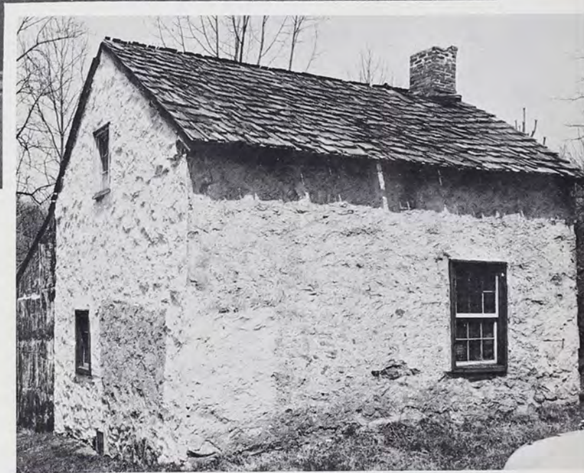
Day's home with cedar-shingled roof located in the forests of Rockland Township, Berks County.
