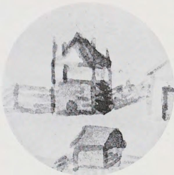
Detail of the barrack in the Lititz painting.
