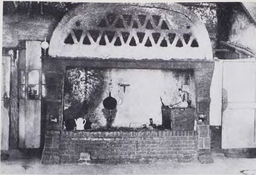
Raised hearth in a jamb-type fireplace in a farmhouse near Kiel in Schleswig-Holstein.
