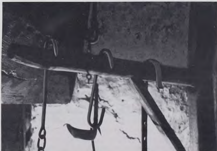
The wooden fire crane in the 1719 Herr House did not swing out of the fireplace as did the iron or steel cranes used by the English. It served to support pots in position over the raised-hearth fires.
