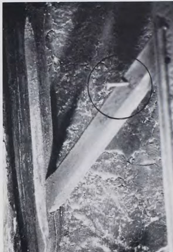
A nail, driven into the diagonal brace of the fire crane in the Herr House, supported a fat lamp used to illuminate raised-hearth cooking.
