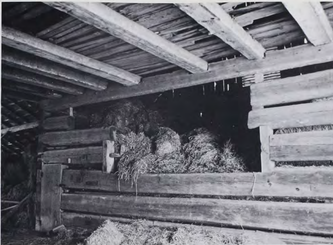
North log-crib mow of Barner barn; note the granary entrance door on left and the log joists above which support the overden.
