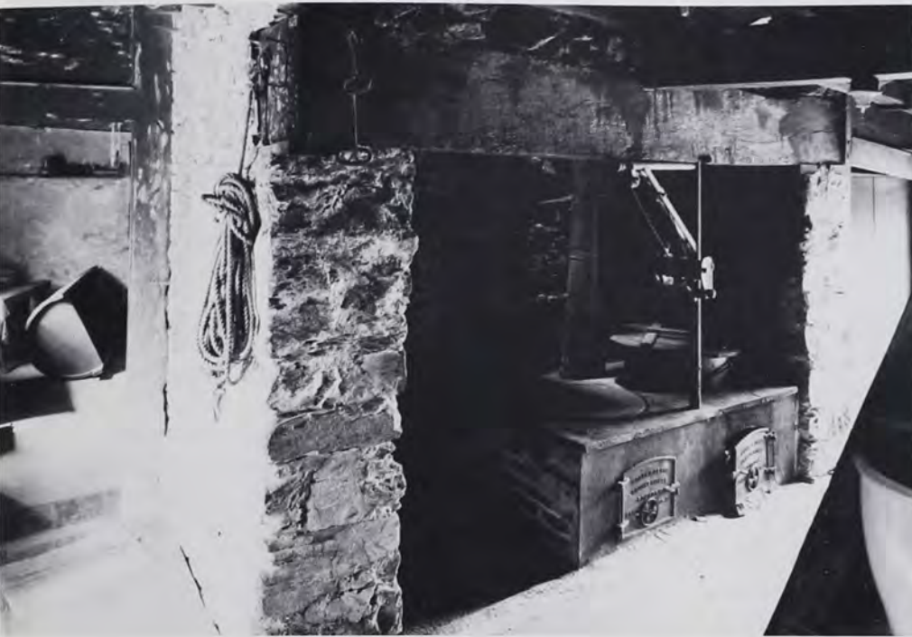
Butchering furnace photographed by HABS in 1958 in the Bertolet cabin. Today no trace of this furnace remains in the cabin, now at the Daniel Boone Homestead.
