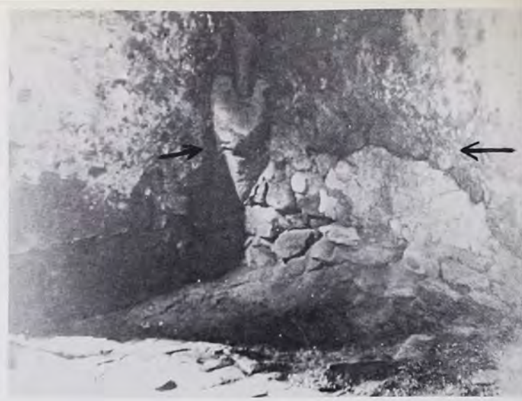
This detail of the ca. 1925 photo of the Herr House fireplace shows a mark on the fire crane support and carbon deposits on the back wall at the two foot height customarily occupied by a raised hearth.
