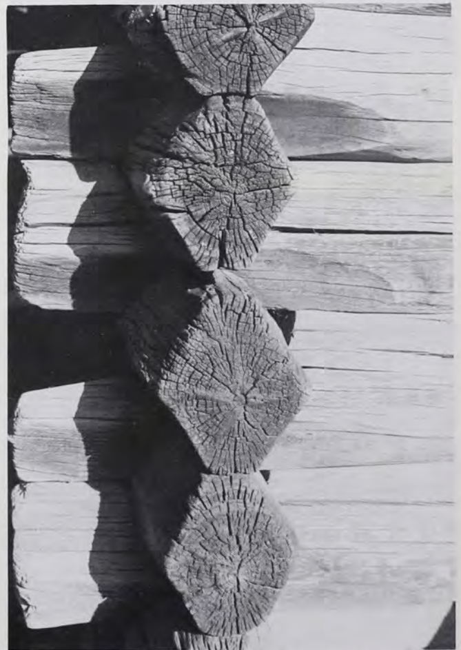
Fig. 11: Diamond-like hexagonal notching dating from 1574, central Dalarna province, Sweden, now in the Skansen open-air museum, Stockholm. It represents type C on Fig. 10. (Photo: T.G.J., 1985.)
