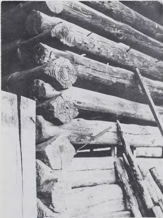
Fig. 1: Round-log diamond notching on a barn in Tuscaloosa County, Alabama. It represents type D on Fig. 10. (Photo 1978, courtesy of Eugene M. Wilson, University of South Alabama.)
