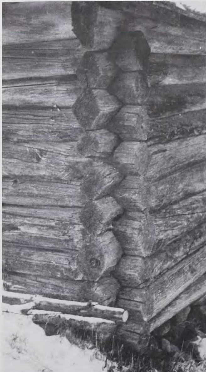
Fig. 14: Diamond-like hexagonal groove notching on a chimneyless hut in Finland. The structure is in Levijoki community, Alajärvi Parish, Pohjanmaa (Ostrobothnia), east of the city of Vaasa. (Photo: Väinö Tuomaala, 1955, courtesy of the National Museum of Finland, Helsinki, photo no. 3195:4a.)
