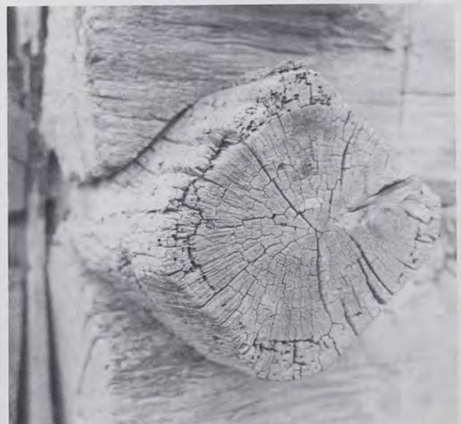
Fig. 2: Hewn, undersided diamond notching in Franklin County, North Carolina, representing type F on Fig. 10. (Photo by T.G.J., 1983.)
