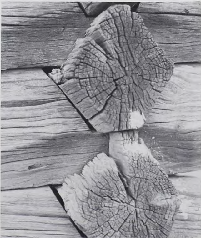
Fig. 9: Hexagonal notching ( sexkantsknut ) on a structure built about 1590 in central Dalarna province, Sweden. It represents type C on Fig. 10. The building is now in the Skansen open-air museum, Stockholm. (Photo: T.G.J., 1985.)
