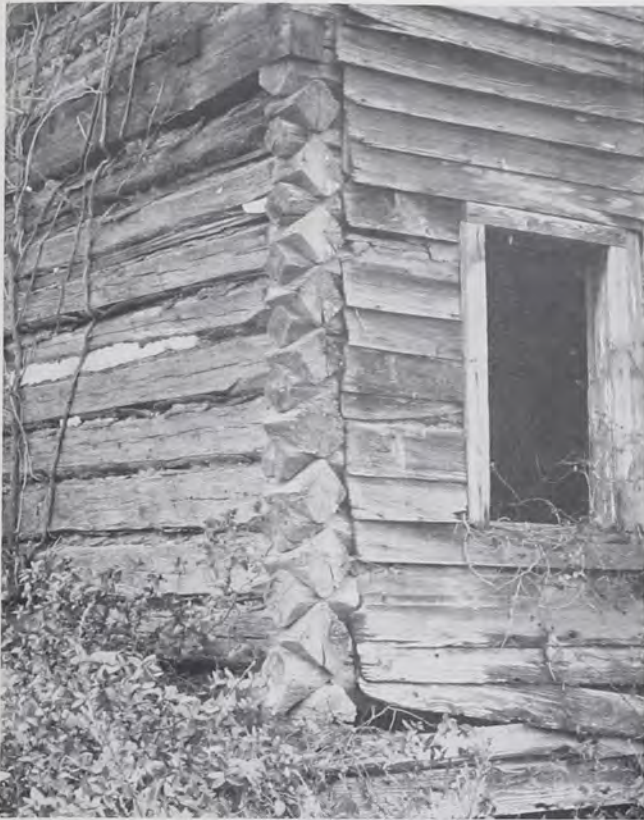
Fig. 6: Hewn diamond notching, on a house built about 1800 in Franklin County, North Carolina. (Photo: North Carolina Division of Archives and History, Raleigh, Catherine W. Bishir, 1974.)
