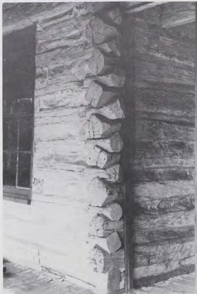
Fig. 4: Hewn diamond notching, mixed with V notching (at bottom), on the Harding house in Davidson County, Tennessee. (Photo: Historic American Buildings Survey, Library of Congress, 1940, by Lester Jones.)
