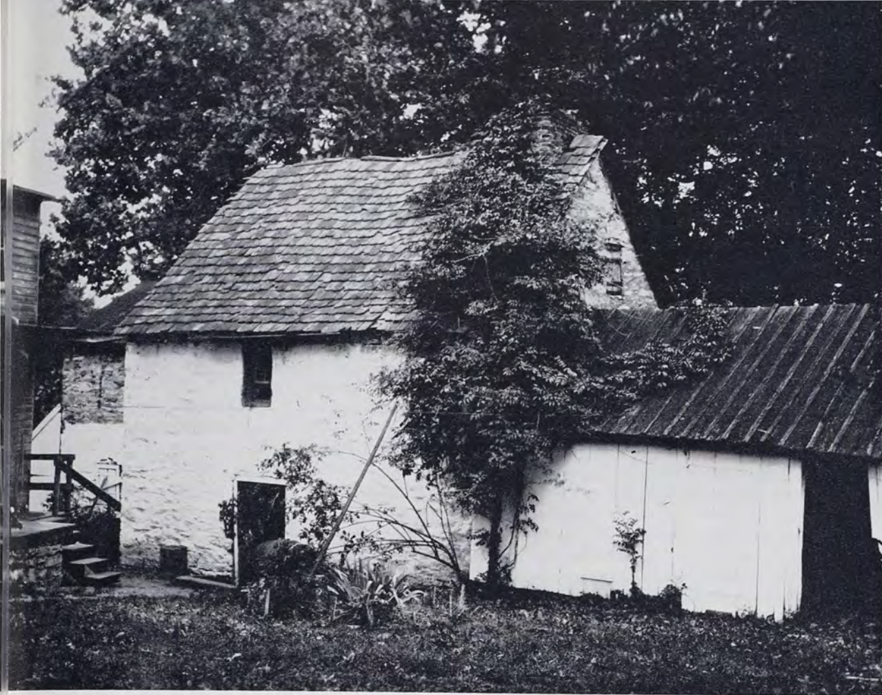
Tile-covered Oley Valley spring-house.
