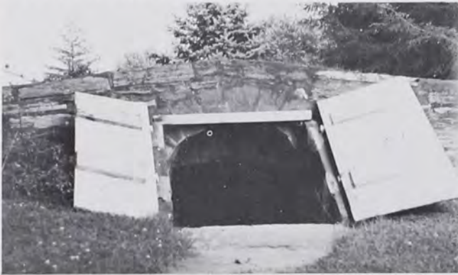
Exterior view of typical and very interesting 19th century cave cellar located in Schaefferstown, Lebanon County, Pa.
