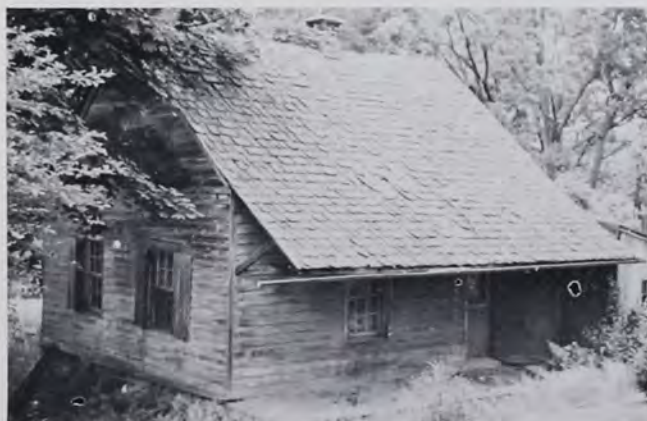
Primitive log cabin structure earlier located north of Main Square in Schaefferstown, Lebanon County, Pa. Note steep roof and central chimney. Now demolished.
