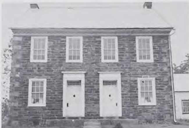
Early stone dwelling with two door front typical of numerous Pennsylvania German houses. Located in Berne area (Hamburg) Berks County, Pa.
