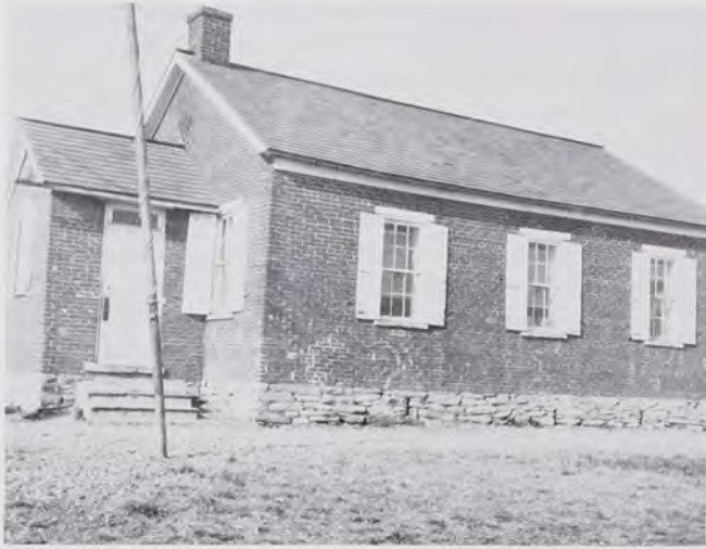
Washington School, presently renovated into a dwelling, located in South Annville, Lebanon County, Pa. Both farm and village children attended such one room schools.
