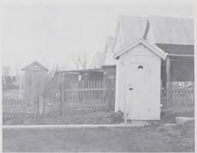
Outdoor privies and sheds in backyard area located in Midway, Lebanon County, Pa. Note crescent design in privy door (foreground) to provide light and air.
