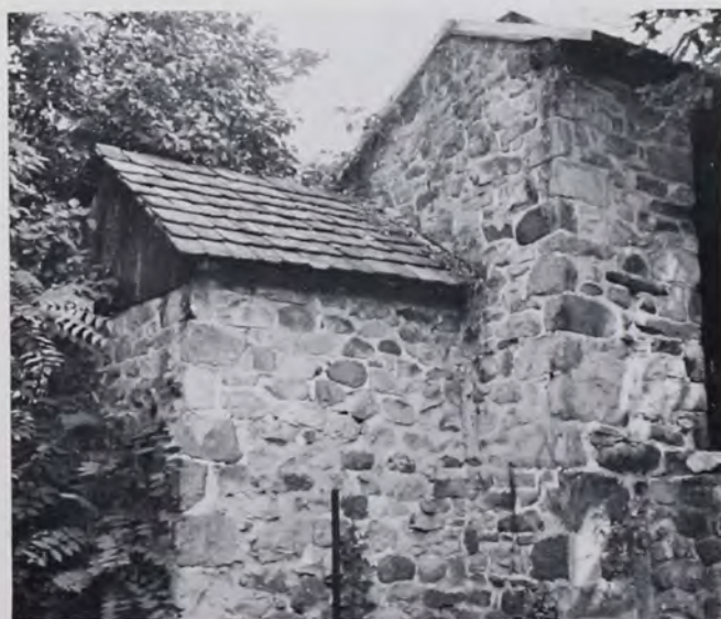
Attached stone bakeoven with red tile roof located in Blandon area, Berks County, Pa.
