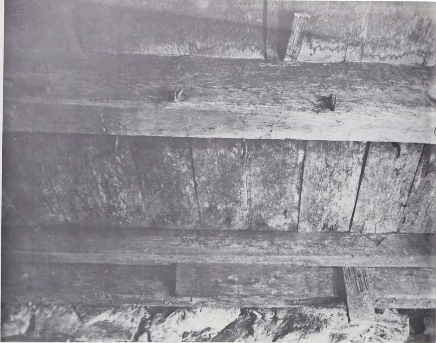
Figure 10. Meat hooks in basement food storage area.
