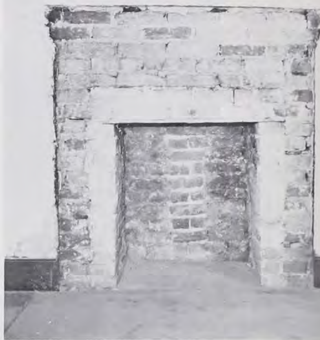
Figure 14. Brick fireplace. They were found in the remodeled sitting rooms.
