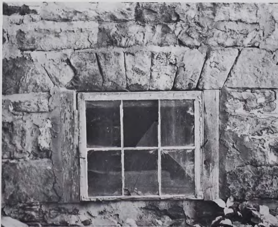
Figure 8. Basement or cellar window showing radiating and keyed stone lintel.
