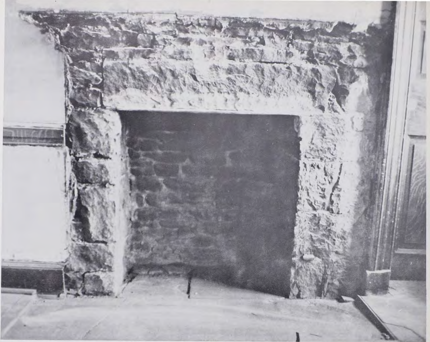
Figure 16. Fireplace with rectangular sandstone block for a lintel.
