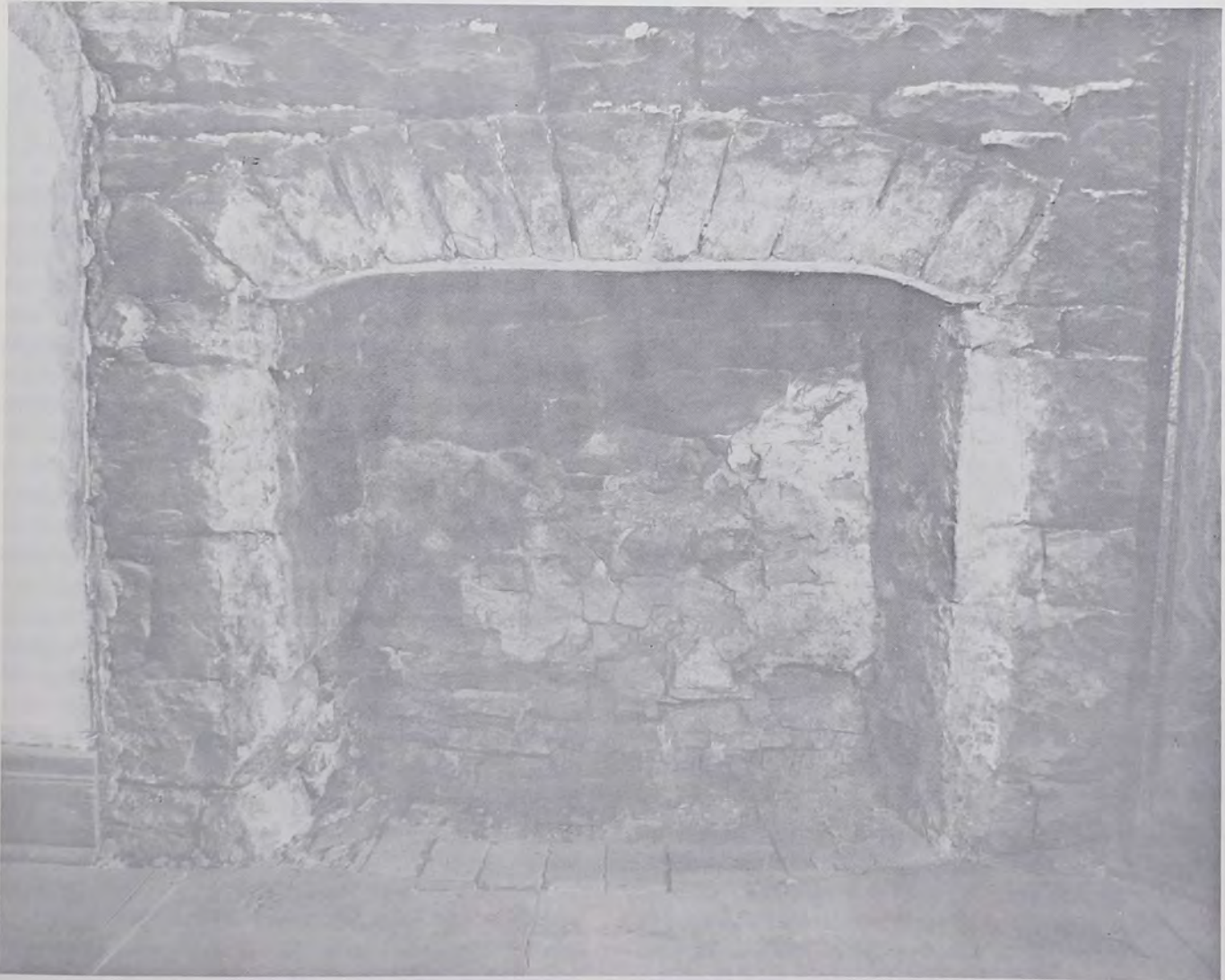
Figure 13. Barroom fireplace. Note the radiating and keyed stone lintel.
