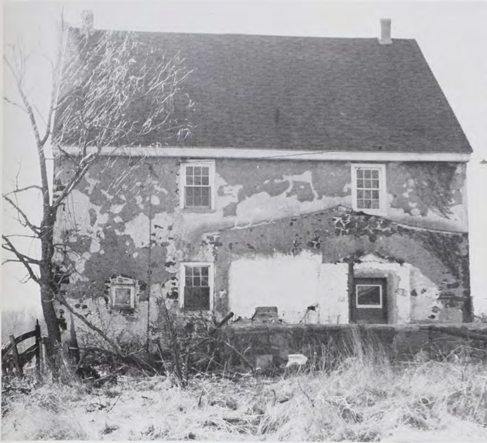
The rear wall of the Antes House. Note the small Seelenfenster on the left-hand side.
