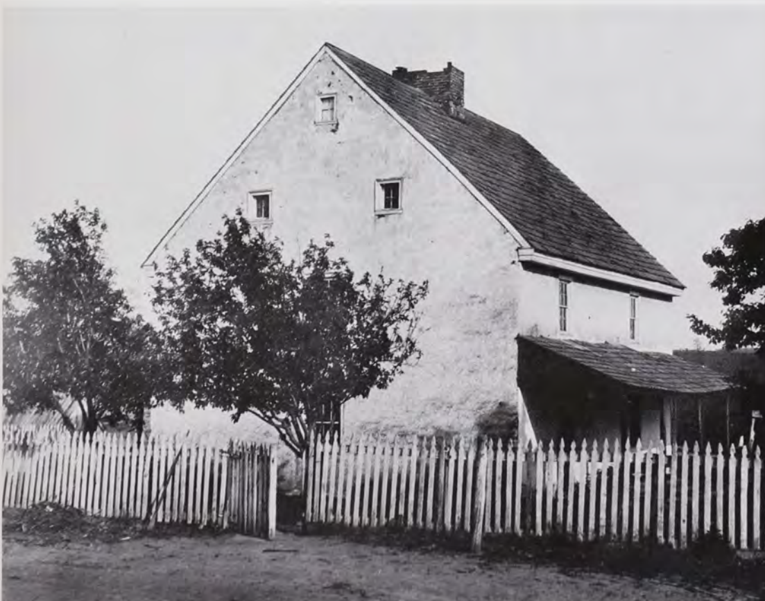
This early photo of the Heinrich Antes Homestead demonstrates the central fireplace and the double attic common to its type. All houses of this type (all houses mentioned in this article are of this type) measured thus far indicate the thirteen-inch foot. This photo probably dates from 1880-1890 and is preserved in the Schwenkfelder Library in Pennsburg, Pennsylvania.
