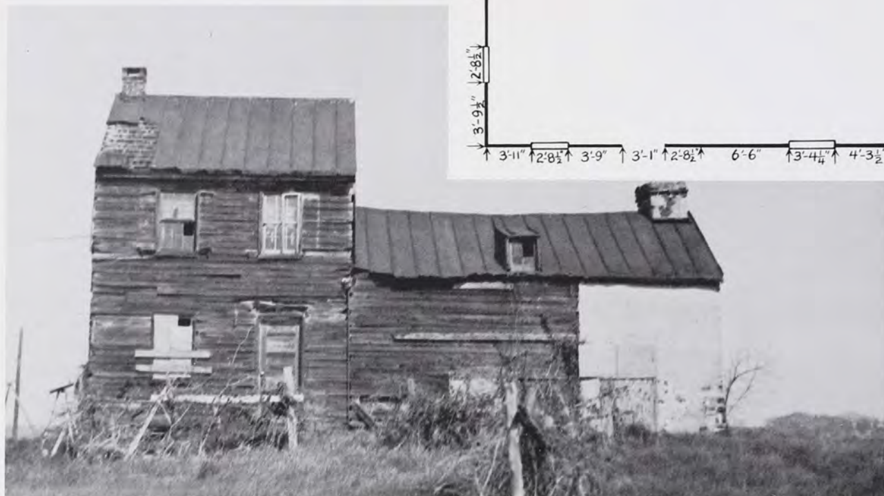
The Yost Log and Frame House. This structure, located in Central Montgomery County, is a significant field demonstration of the two standards of measurement. The older right-hand part is log construction, of English origin, and measured with the ordinary 12-inch foot. The frame left-hand portion is of a later date, and shows the Germanic (13-inch foot) measurements. Site documentation shows the later owners to be German.
