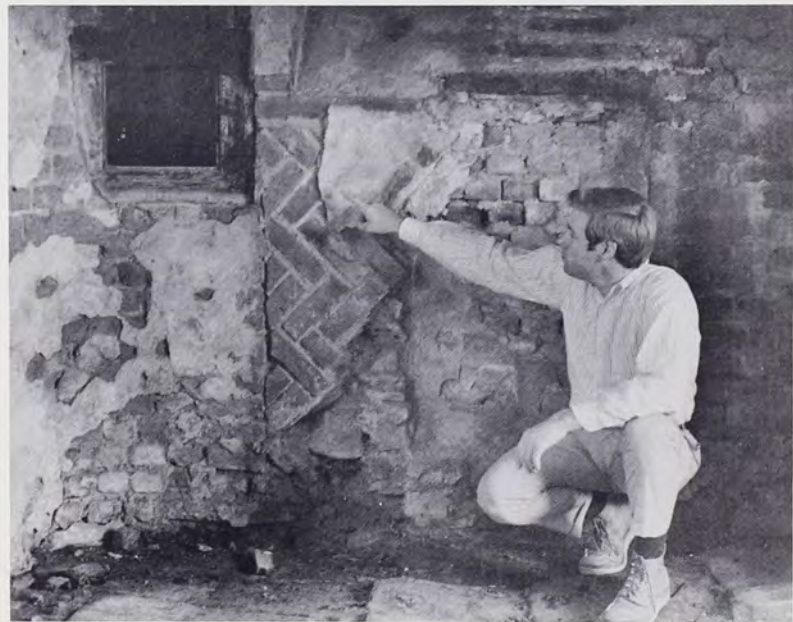
John D. Milner, restoration architect and co-author, points out herringbone brick fire-back and wood-framed niche in fireplace of Thomas Massey's 1696 brick house.
