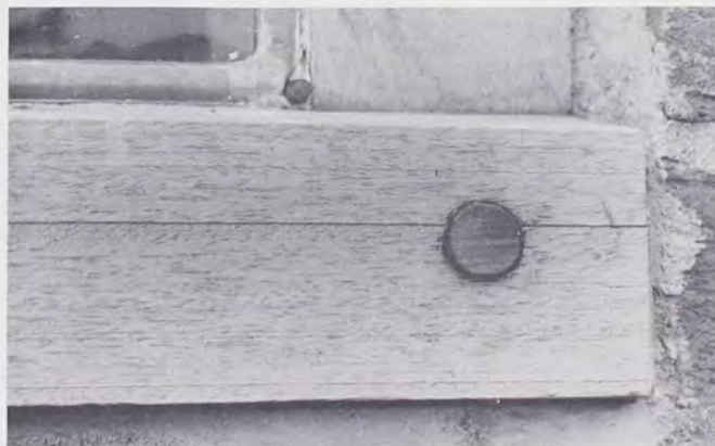
Windowsill detail of restored leaded glass window.
