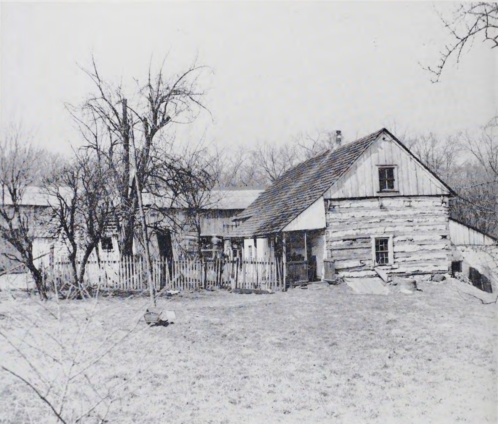
Early rural Pennsylvania buildings were overwhelmingly of log construction. Today few evidences of the eighteenth century log culture survive. Here is a photograph, taken some thirty years ago, of a small log farmstead near Fleetwood, Berks County.
