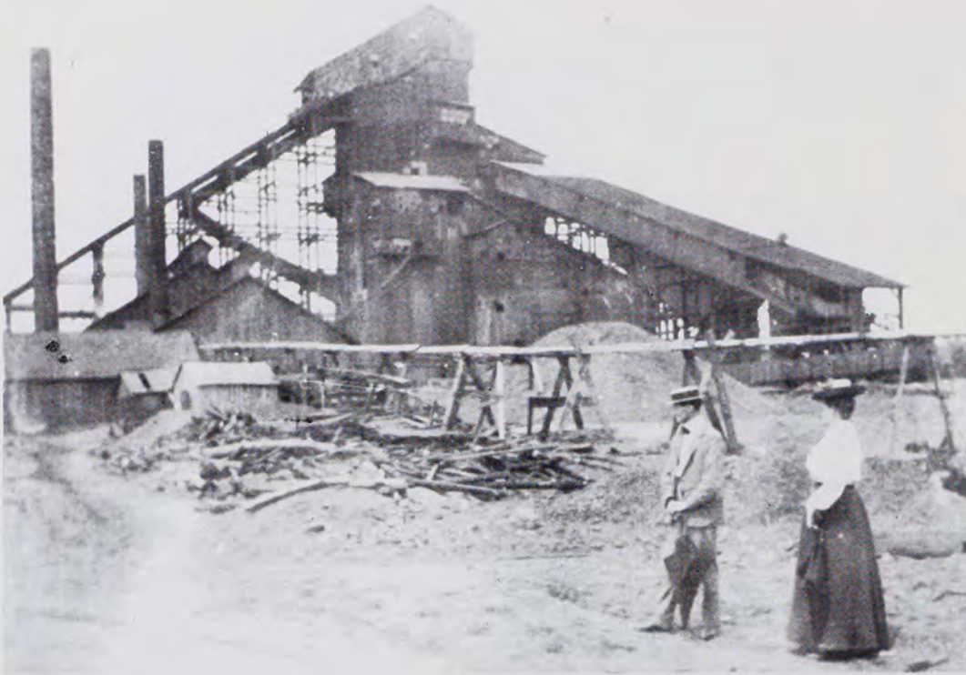
The coal breaker at Eckley, Pa. at the turn of the Century. It is the breaker which the tourist most often notes as the visible portion of the mining operation. The breaker, however, is only one small segment of the total mining operation. It is the final operation of the mining process wherein the coal is segregated from the rock, slate, and other foreign matter. A similar breaker on the site of this one was constructed by Paramount Studios for the film "The Mollie Maguires" in 1968.
