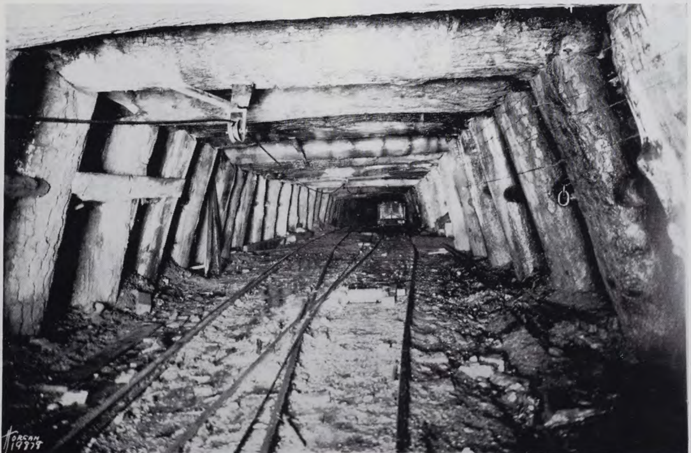
When the coal car is filled it is transported along the "gangway." This picture displays the size and number of supporting timbers which help to retard cave-ins. Unfortunately, however, mine disasters still occurred and many a miner's burial crypt rests under tons of earth and coal.
