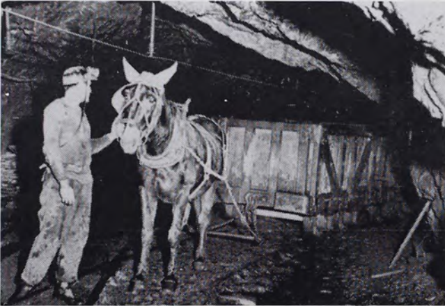
Until the introduction of "electric mules," the mule provided the energy to transport the coal from the mine to the surface. The mule driver and his mule spent a long day working together. This picture was taken in "No. 10" shaft near Eckley.
