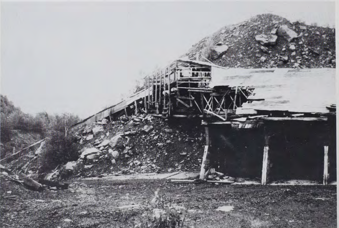
This abandoned slope located in Eckley, Pa., was operational into the 1950's. Until recently it stood as a reminder of Eckley's past importance as a "patch town." Stripping operations resumed on this site in late 1974, destroying these last vestiges.
