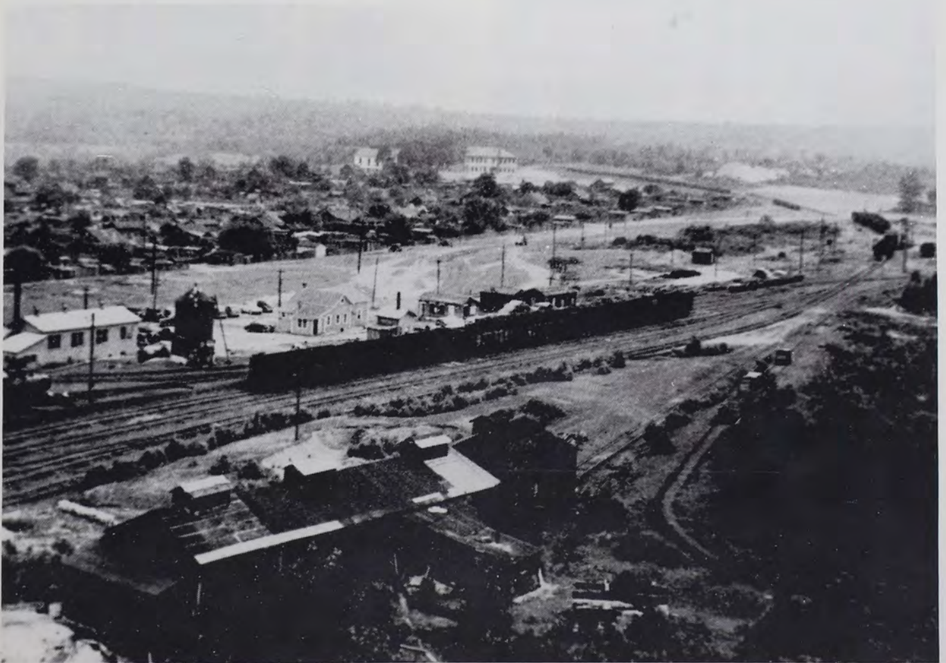
A ca.—1930 picture of Eckley's Colliery shows a shipment of coal waiting transport to Hazleton. This is one of the few panoramic views of Eckley ever taken. Many buildings pictured here do not exist today.
