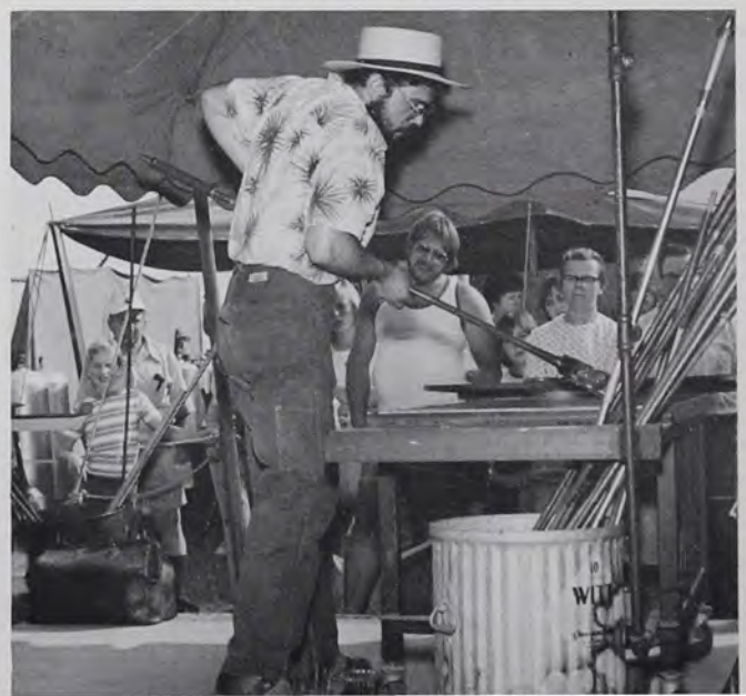
Then the blob of glass is rolled on a metal table to get a symmetrical shape.
