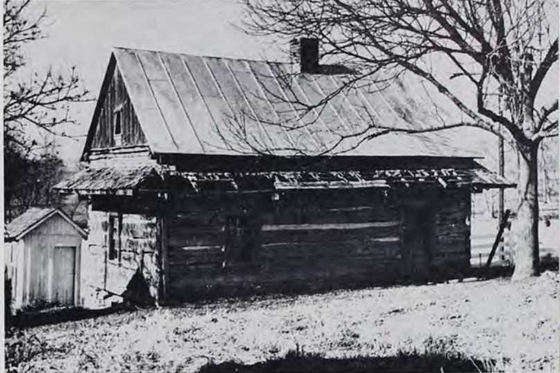
The Seibert Cabin—Lebanon County. Unusual pent roof, typical fenestration, original half doors in front.
