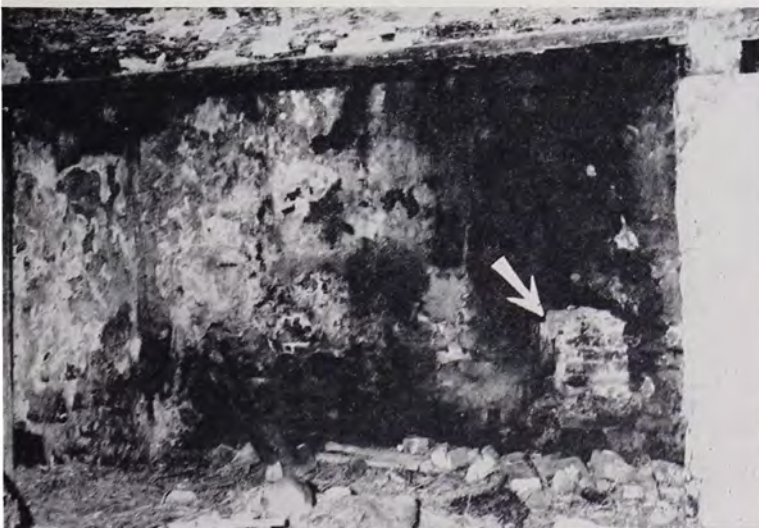
Fireplace in the Dietz Cabin, showing opening, in lower right corner, for the five-plate stove.
