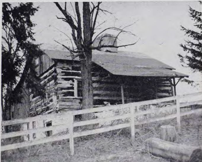
Log House—Lebanon County. Upper part destroyed by fire. Has two fireplaces of twelve-foot size.
