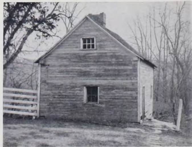
The Darkes Cabin—Berks County. A bank house with fireplaces on both levels. Note use of stone below ground level.
