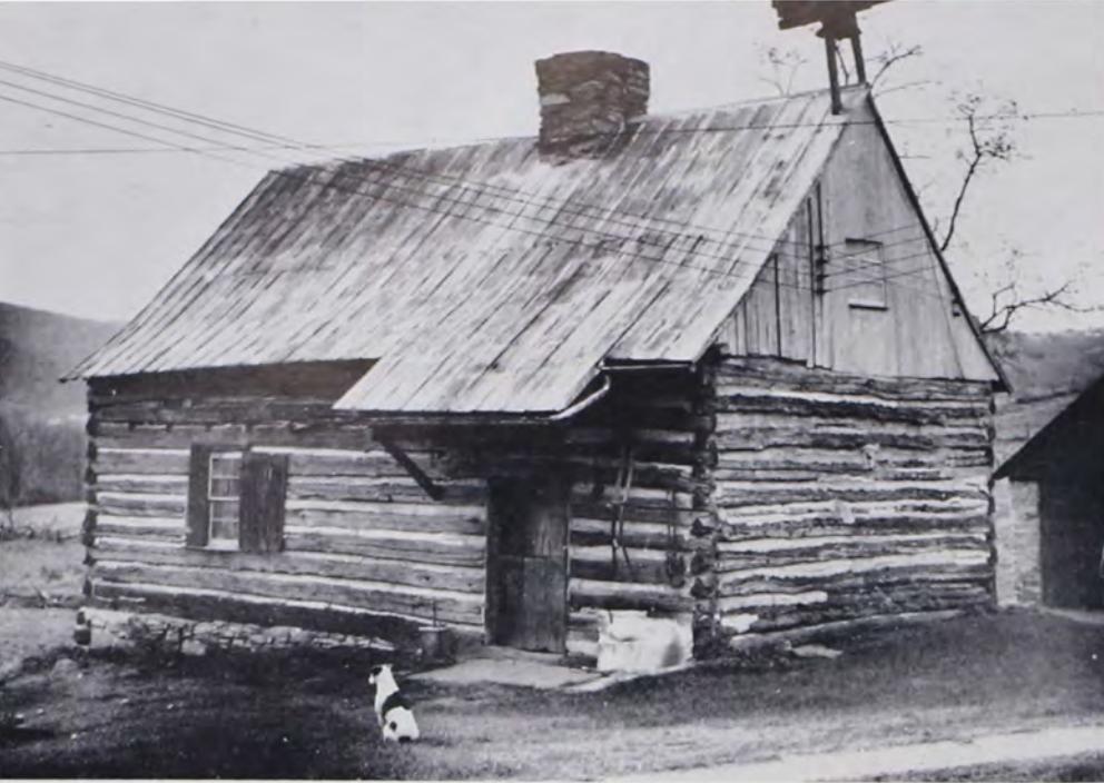
The Schneider Cabin—Oley Valley. Note the central chimney, vertical gable siding and few windows.
