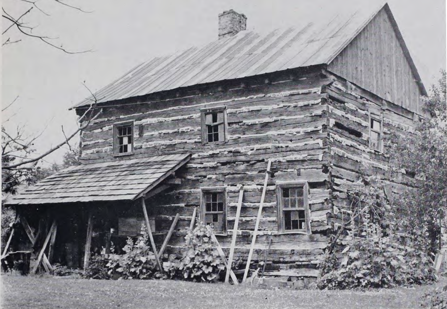
The Schultz House—Montgomery-Lehigh County line. Best known two and one-half story log house—of Schwenkfelder origin.
