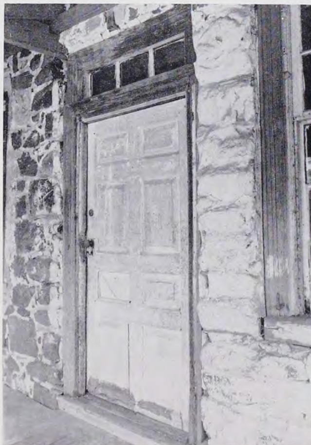
Exterior Front Door, Chadds House.
