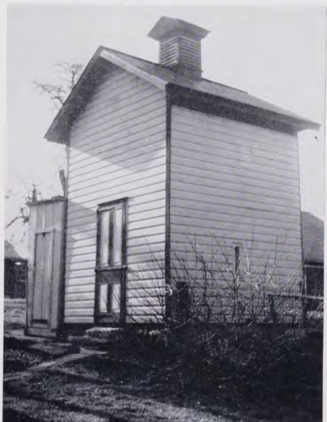
FRAME SMOKEHOUSE. On Allen Dundore Property, South Lebanon Township. Note slate roof, air vents on side and roof. Photographed 1960.
