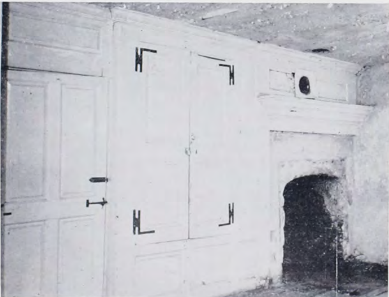
Fireplace, Closet, and Cellar Stairway Door—West Room of First Floor—Chadds House.
