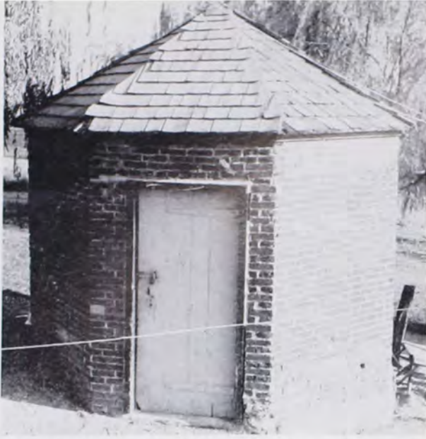
HEXAGONAL SMOKEHOUSE. Built about 1850 by Michael and Lucy Ann Killinger, on what is now the Millard Property, Northwest of Annville. Dimensions: 12 feet across inside; hexagon section: 5 feet; height: 8 feet to roof, 12 feet including roof; door 6½ feet by 3 feet. Now used for dog shelter.
