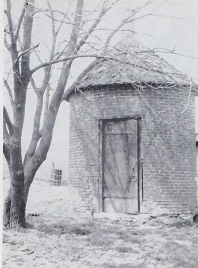
ROUND BRICK SMOKEHOUSE. Built about 1850 by Henry and Barbara Bowman. Located on Clinton Mark Property, North of Palmyra. Diameter: 8 feet; height: 10 feet; pit: 18 inches by 10 inches; door: 6½ feet by 2½ feet. Photographed 1969.
