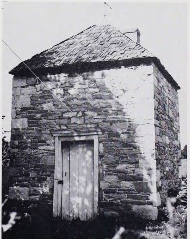
EARLY STONE SMOKEHOUSE. On Kingsley Property South of Annville on Route 934. Dimensions: 12 feet by 12 feet by 15 feet, including 3-foot roof. Photographed 1961.
