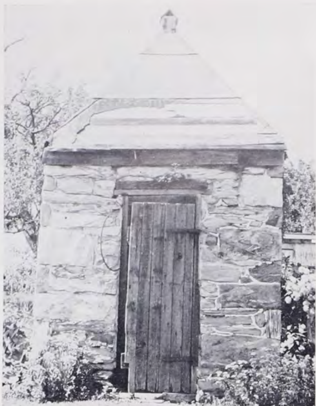
STONE SMOKEHOUSE. Located on Roy Shenk Farm on Route 934 in South Annville Township, over 100 years old. Dimensions: 8 feet by 8 feet by 12 feet, roof 4 feet high. The roof structure is unusually steep. Photographed 1961.
