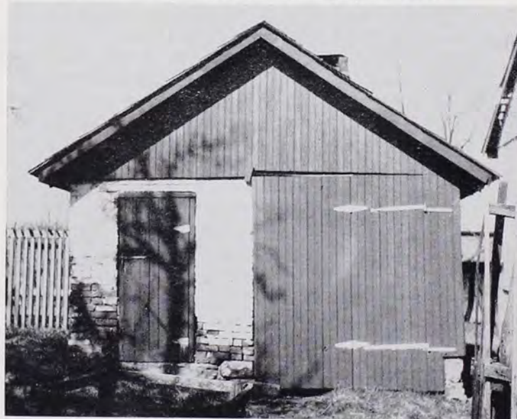
COMBINATION SMOKEHOUSE AND BUTCHER-HOUSE. On Benjamin Hoyer Property, East Hanover Township, near Harper's Tavern. Photographed 1960.
