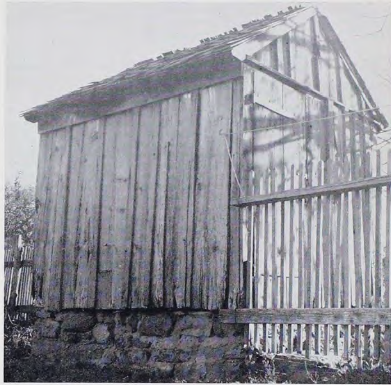
FRAME SMOKEHOUSE. Located on Harold Blecker Farm South of Kleinfeltersville, built in latter part of 19th Century. Dimensions: 7\frac{1}{2} feet long and 7 feet wide. Height: 8\frac{1}{2} feet to roof, foundation 33 inches, 10 feet including roof. Photographed 1960.
