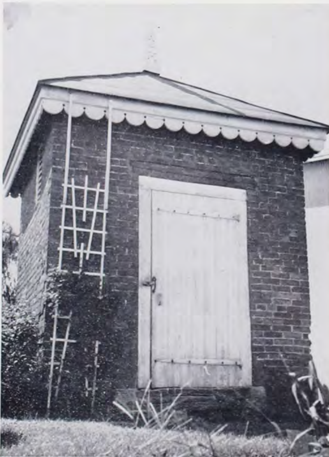
VICTORIAN BRICK SMOKEHOUSE. Located on Howard Schwenk Farm, East of Fontana on Route 322. Dimensions: 9 feet by 9 feet by 12 feet, roof two feet. Photographed 1961.
