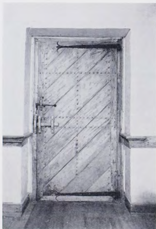
Paneled Door in Southeast Room, First Floor, Temple House.
