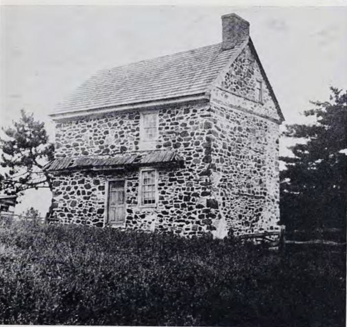
Chadds House about 1905. North Side Showing Pent Eave. Original in Chester County Historical Society.
