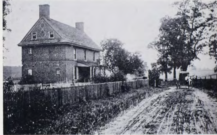
Early Photograph of Barnes-Brinton House, circa 1905. Original Print in Chester County Historical Society. Note pent roof and brick patterns on gable end.
