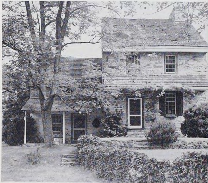
Temple House, West Bradford Township. Built by Thomas Arnold who bought land here in 1713 and lived here about half a century, erecting a fulling mill about 1730. The house is dated circa 1720-1730, and was rebuilt or remodeled, according to a date-stone of 1774, by William and Ella Cooper. The Temple Family owned it from 1822 to 1916, the Coopers from 1760 to 1818.
