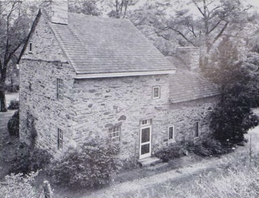
North and East Side, Temple House. In the kitchen there is still a hole in the wall where originally a stone sink stood.
