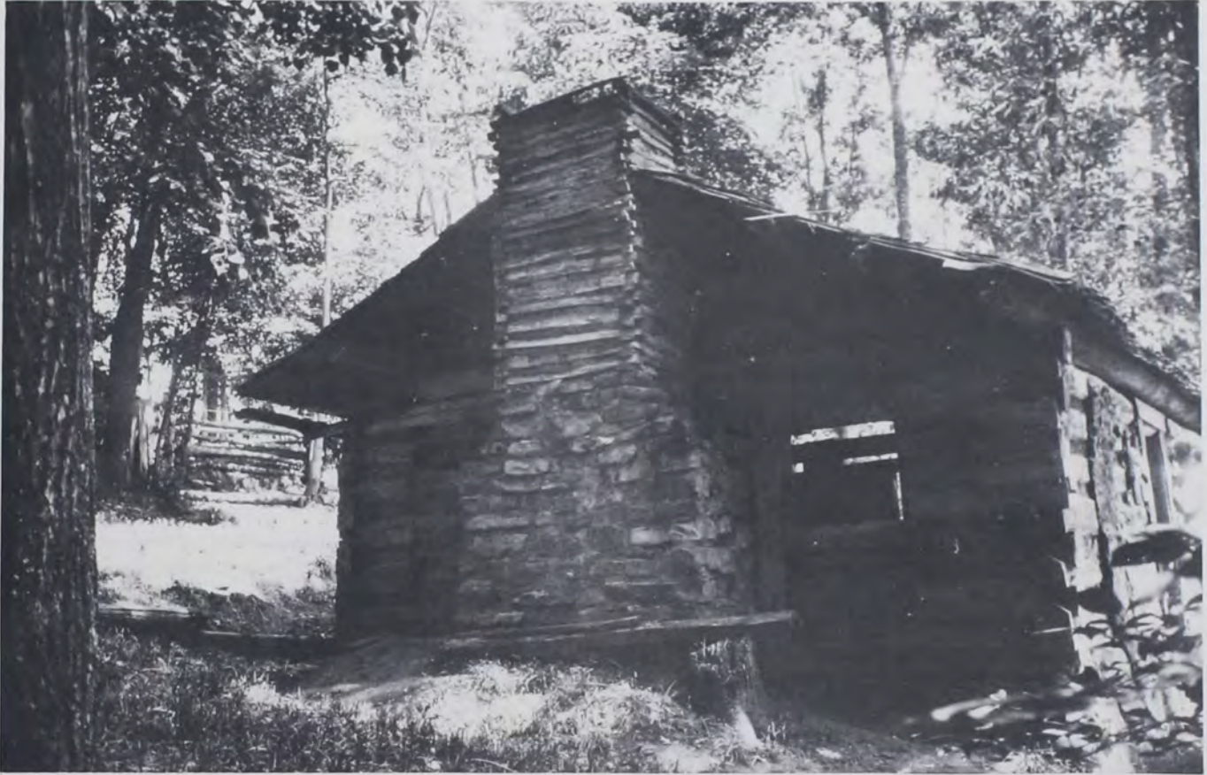
Fig. 4. The cabin-house from Anderson Co., Tenn., showing its chimney with stone base and stick-and-clay shaft. Windows and an overhanging roof, atypical of cabins, are used in this combined form. Museum of Appalachia, Norris Tenn. (PIC, 1990).
