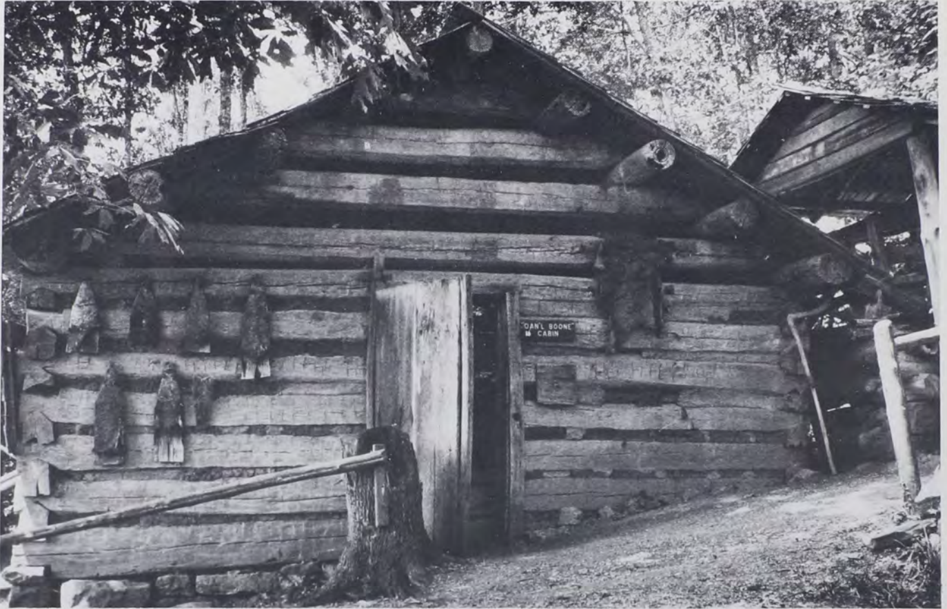
Fig. 3. A cabin-house from Anderson Co., Tenn., combining a cabin's hallmark purlin roof, typical dirt floor and low, one-story form with hewn logs (here V-notched), as in log houses. Now at the Museum of Appalachia, Norris, Tenn. (PIC, 1990).
