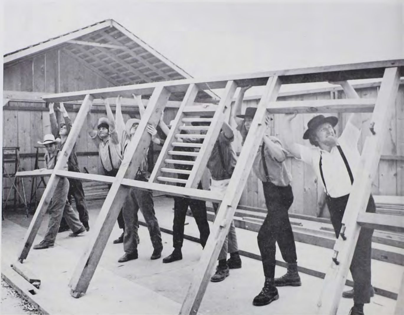
Here the section of wall, now completed, is being raised into position. Doing the raising are Roth, Schukraft, Tenaglia, Lilienthal, Gougler, Bond, Marc Williams, and Lutz.
