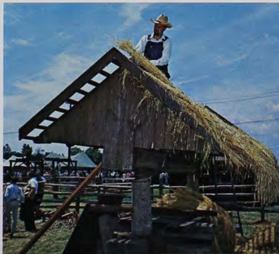
Richard thatches the roof of an 18th-century Cider Press.
