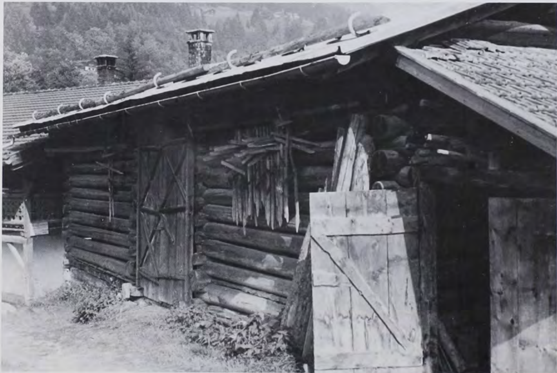
Fig. 3: The upslope eave side, or rear, of a double-crib forebay barn in Saas, Prätigau. Chink construction allows ventilation of this upper level, which contains the feed bins and a central wagon runway/threshing floor. A small artificial bank facilitates entry to the runway.
