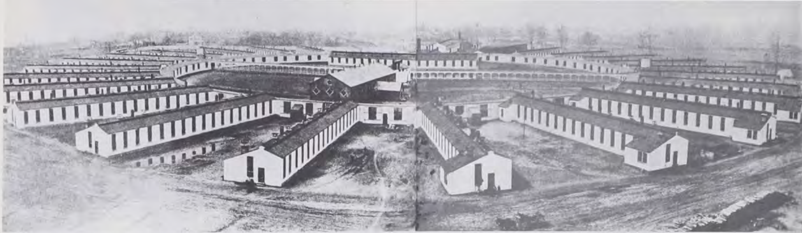
United States general hospital at Jeffersonville, Ind. "This type of hospital was highly recommended by the United States medical department . . . The wards radiate like the spokes of a wheel from a covered
