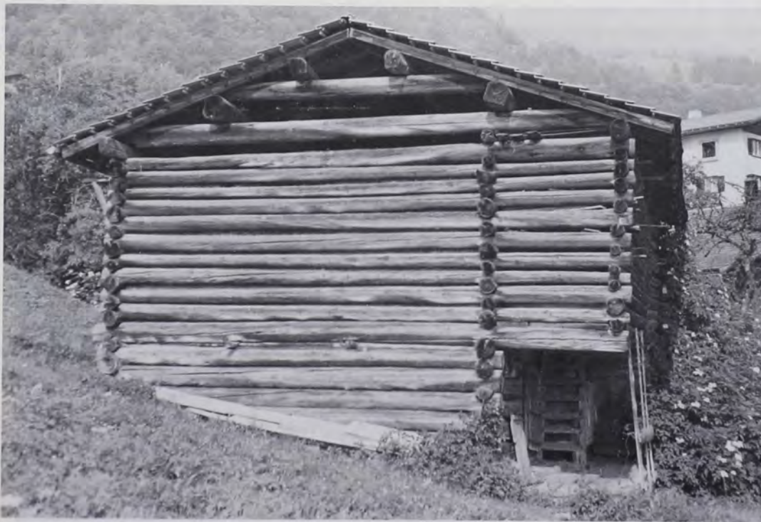
Fig. 1: Side view of double-crib log forebay barn in the village of Saas, in the Prätigau, Canton Graubünden, Switzerland. Stalls are below, feed storage on the upper level, accessible from ground level on the uphill eave side. Note the stair beneath the forebay, the log wall closing off the Talina on the forebay level, and the open chinks in the gable to ventilate the hayloft. (Photo by the author, 1978.)
