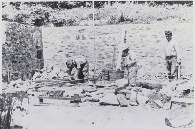
Laying up the stones for the base of the kiln.
