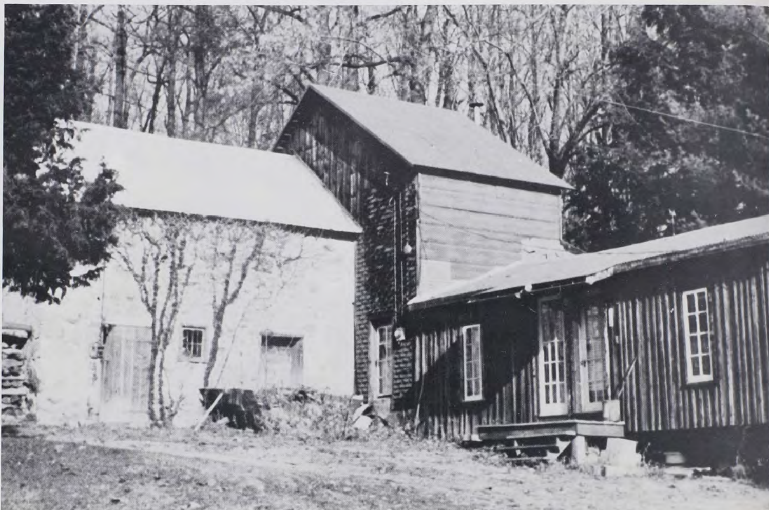
The Stahl Pottery. The stone section houses the pug mill, and the center section was where the pottery was turned and dried; Russell Stahl added the low section (foreground, right) at a later date.
