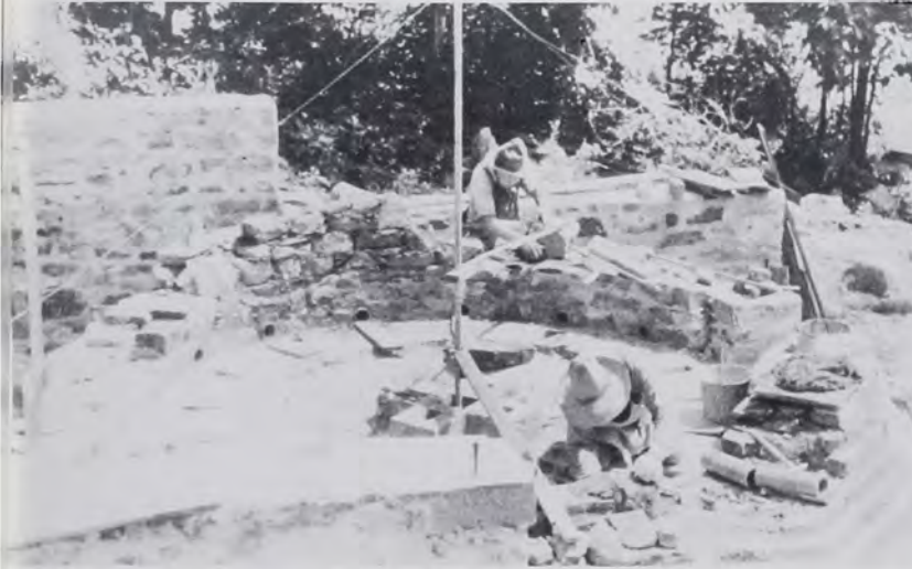
Beginning to lay the foundation of the Stahl brothers' kiln.
