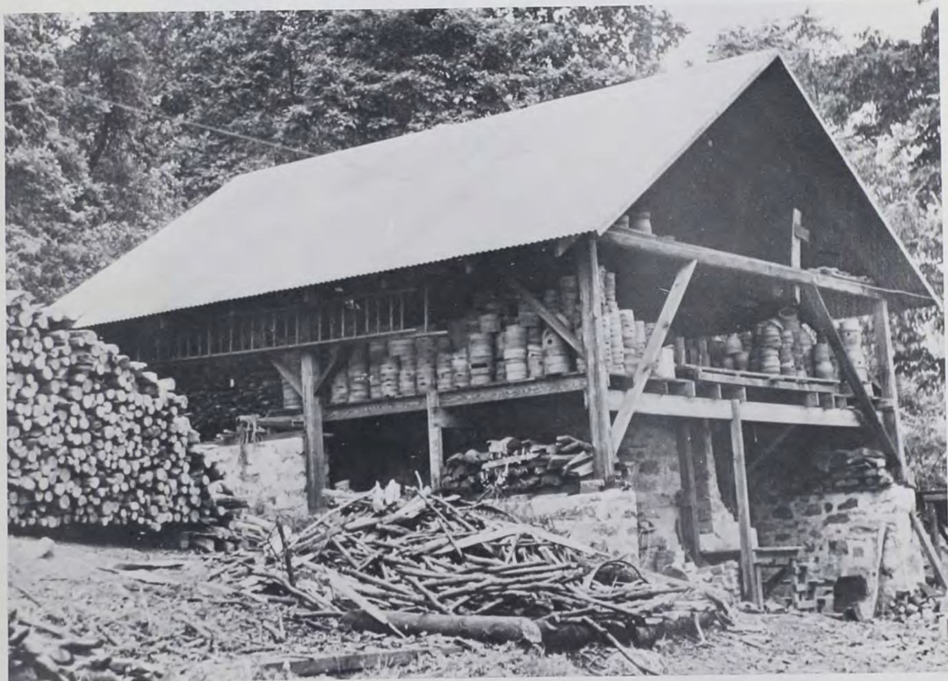
Kiln and shed with stacks of firewood and saggers; since this picture was taken a wing has been added at the left to protect the firewood.
