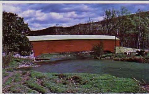
4 GRIESEMEMER'S MILL BRIDGE Over Manatawny Creek, 1 mi. s. of Pleasantville Bridge.
