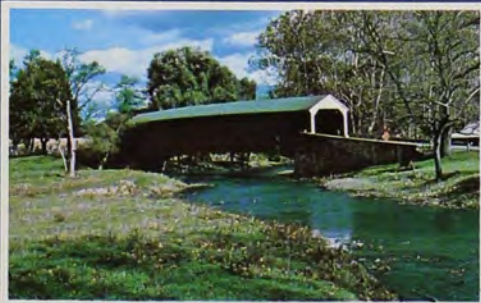
3 PLEASANTVILLE BRIDGE Over Manatawny Creek at Pleasantville. 8 mi. w. of Boyertown
