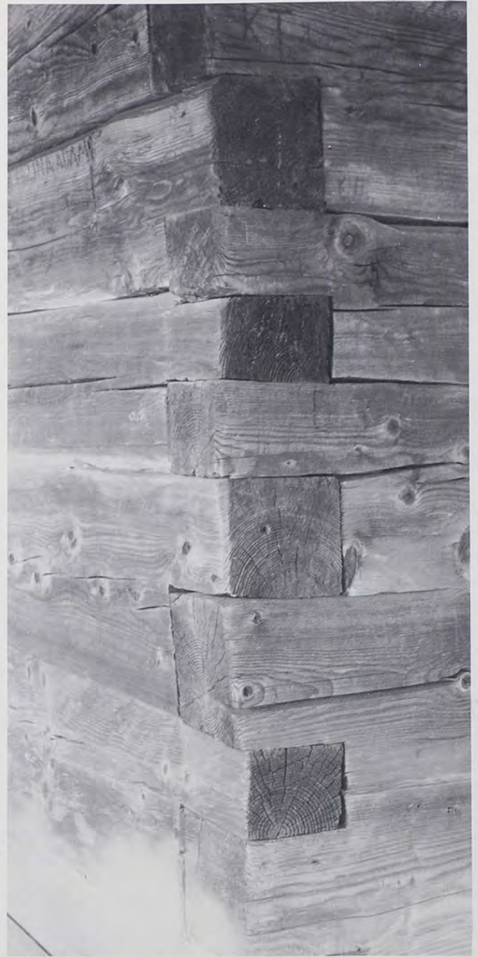
Fig. 18: Square notching, mixed with half notching, on the chinkless wall of the Chabowka church, near Rabka, south of Krakow, in Poland. The church dates from 1757. (Photo by T.G.J., 1982)
