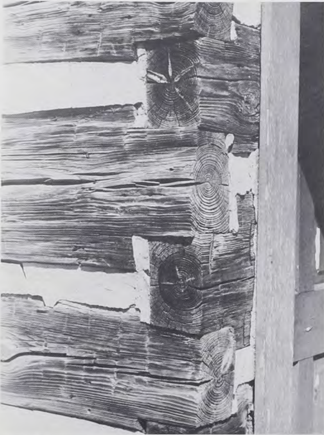
Fig. 1: Square notching on hewn logs, near Durant, Bryan County, Oklahoma. (Photo by T.G.J., 1981)
