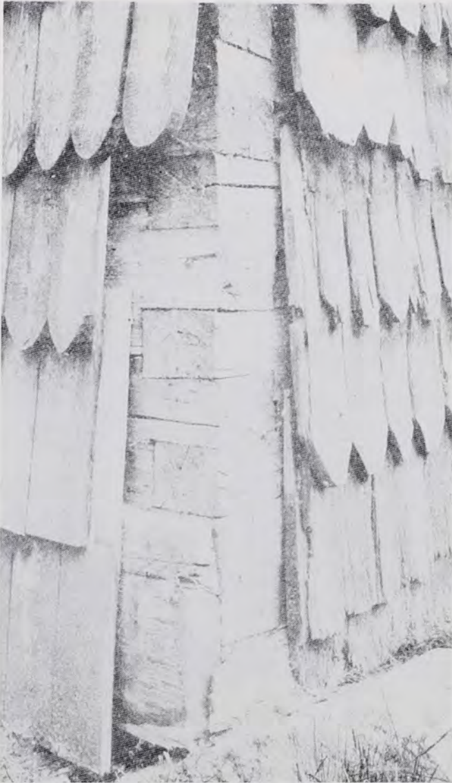
Fig. 5: Medieval Swedish square notching, mixed with full-dovetailing, on the 1323 Södra Råda log church in Värmland province, Sweden. The notching is normally covered with shingles, as during my 1981 visit, but this photograph was taken during restoration work. (Photo from Boëthius, Studier, cited in endnote 29, p. 319; copy courtesy the Harry Ransom Humanities Research Center at The University of Texas, Austin.)
