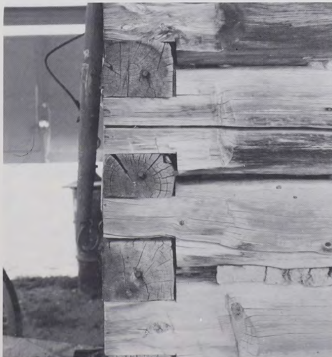
Fig. 9: Rocky Mountain square notching hewn only near the corners, with the greater part of each log left round. This technique, possibly an archaic Pennsylvanian frontier method now surviving only in the mountain West, has abundant northern European prototypes. The structure stands near Jackson, Beaverhead County, Montana. (Photo by J.T.K., 1989)
