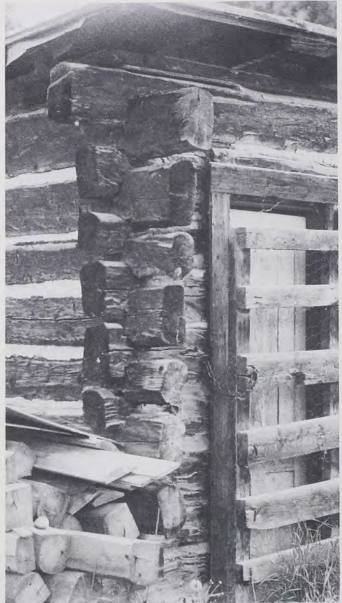
Fig. 26: Vertical double notching, Lake City, Hinsdale County, Colorado. Such notching, we feel, once co-existed with the square notch in the eastern United States, as part of the Pennsylvania carpentry tradition, and its presence in the Anglo Rockies, in our view, represents an archaic survival of a frontier type. The Anglo-American/Midland cultural context of this structure is revealed by the score marks left from typical Pennsylvania ax-and-adze hewing and by the chinked construction. (Photo by T.G.J., 1987)
