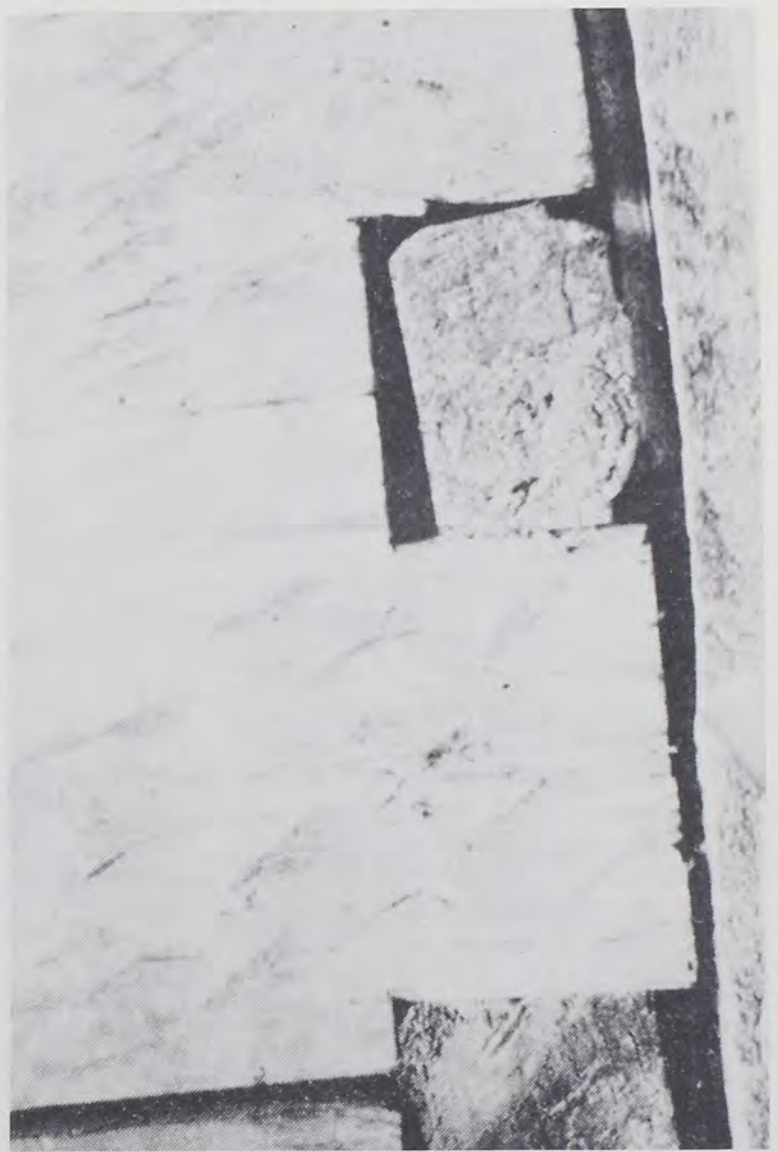
Fig. 13: Chinkless square notching in the New England garrison house carpentry tradition, alien to the Pennsylvanian culture complex. The structure, the Gilman Garrison House at Exeter, New Hampshire, allegedly dates to about 1650. Square notching was not used consistently in the building. This tradition apparently never spread westward, remaining confined largely to the Maine-New Hampshire border area. (Photo copied from Mercer, "Origin of Log Houses," see endnote 3, p. 12.)
