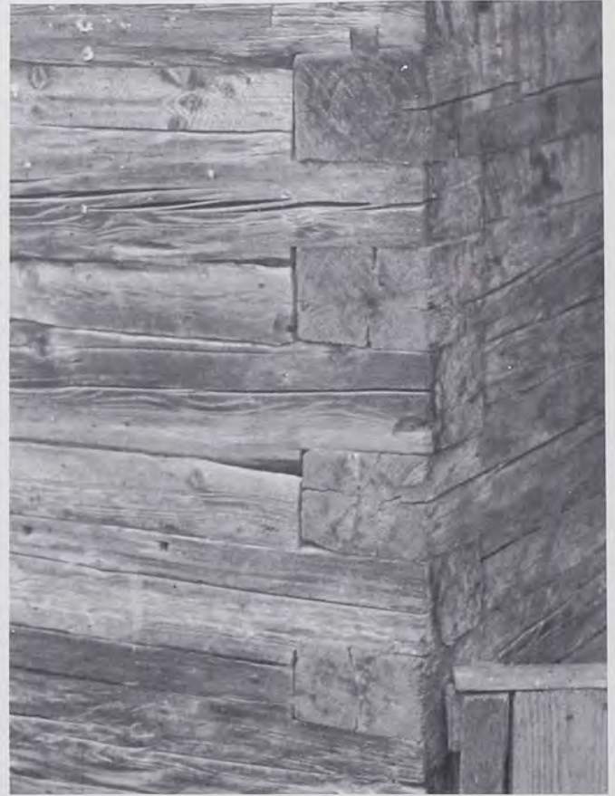
Fig. 2: Slavic square notching, in the village of Belá, near Žilina in western Slovakia. The narrow wooden strips conceal chinking. Square notching is common in many Slavic regions of eastern Europe. (Photo by T.G.J., 1982)
