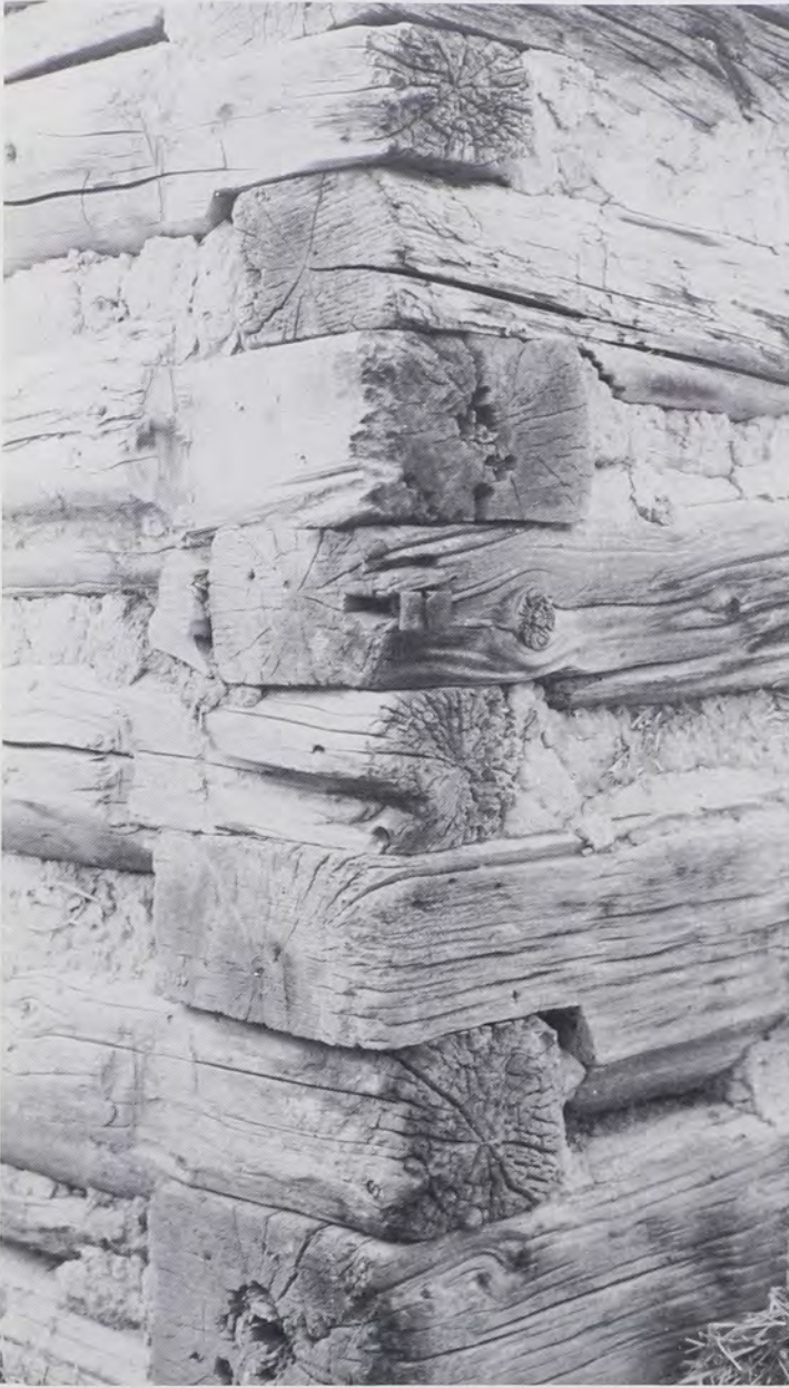
Fig. 10: Canadian square notching, on logs hewn only near the corners, at Black Creek Pioneer Village, Toronto, Ontario, a museum displaying the folk architecture of the northern shore of Lake Ontario. (Photo by T.G.J., 1984)
