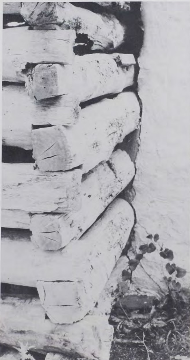
Fig. 7: Pioneer cabin with square notching applied to split-log construction. Dating to the 1830s, this cabin is one of the oldest structures in Gonzales County, Texas. (Photo by T.G.J., 1989)
