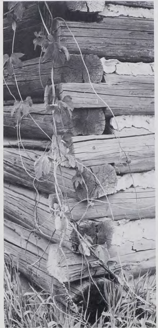
Fig. 6: Square notching on round logs, in the Rocky Mountains of Benewah County, Idaho, a common type in the western mountain districts of North America. (Photo by T.G.J., 1987)
