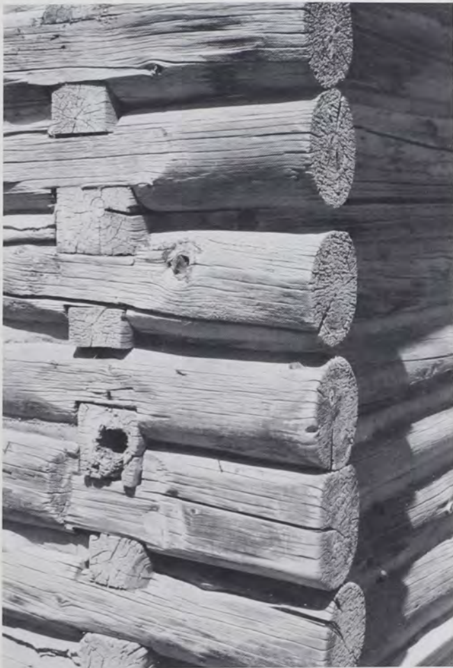
Fig. 23: Mixture of square and vertical double notching, hewn only at the joint, in the Grand Encampment open-air museum, Carbon County, Wyoming Rockies. This combination strongly suggests a genetic link between the two notch types within the Midland American carpentry tradition. Compare it to Fig. 22. (Photo by J.T.K., 1989)
