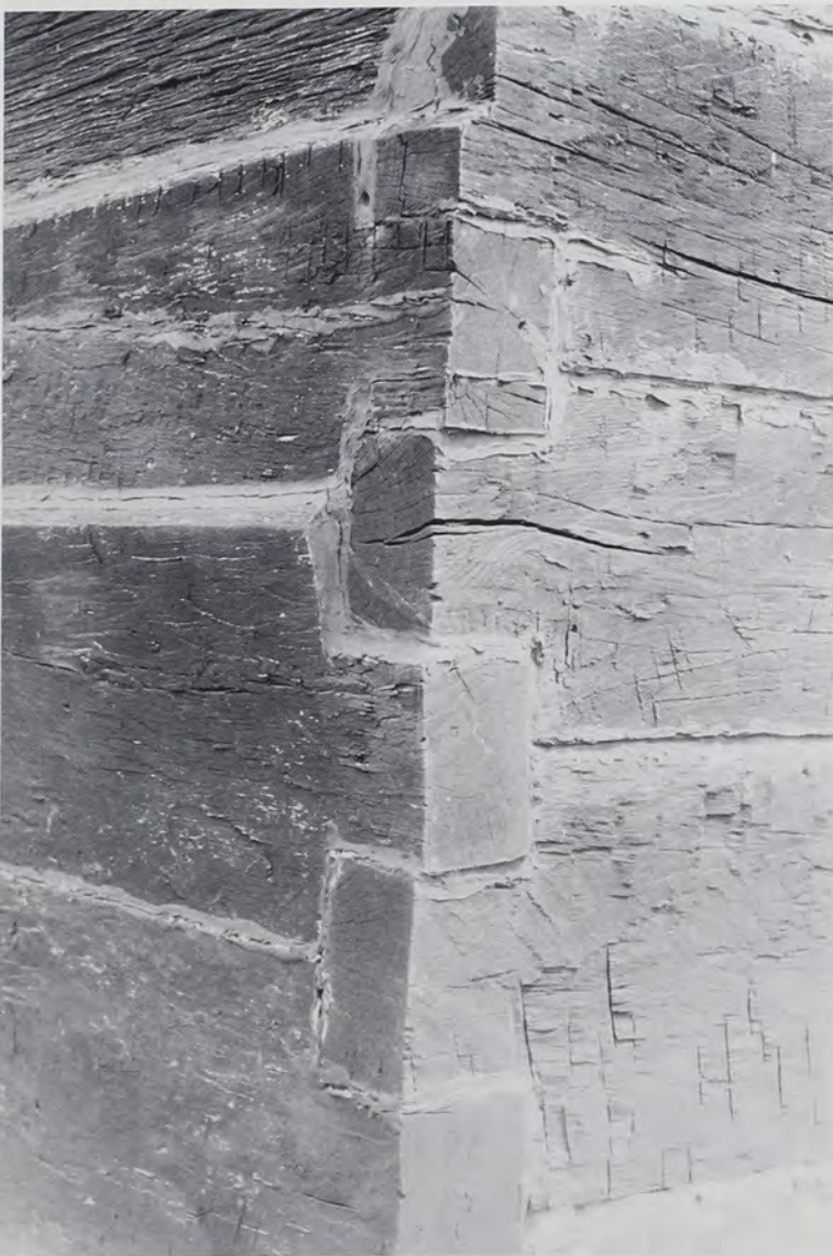
Fig. 12: Chinkless, square notched wall on the John Morton house, Prospect Park, Delaware County, Pennsylvania. This room of the house, built in the middle 1700s, ties square notching to the Pennsylvania hearth area of American notched log construction and to the area and people of the colony of New Sweden. (Photo by T.G.J., 1980)
