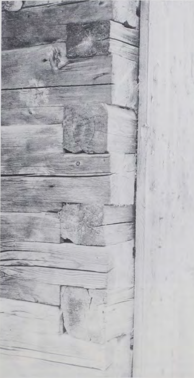
Fig. 19: Square-notched cowshed ( ladugård ) in Voxtorp open-air museum, near Värnamo in Småland province, Sweden. Built in the first half of the nineteenth century, the shed is typical of many in the area. (Photo by T.G.J., 1989)
