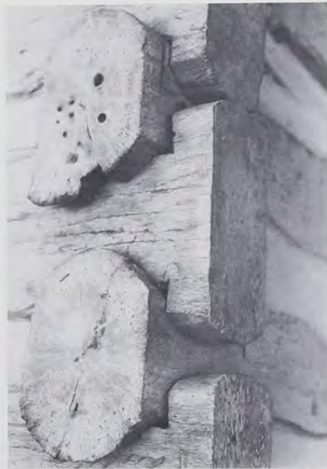
Fig. 24: Vertical double notching dating from about 1850 on the Campbell log house, 211 East Liveoak Street, Seguin, Guadalupe County, Texas. Note the thinness of the crowning. The Pennsylvania/Midland heritage of this dwelling is abundantly revealed in its "dogtrot" double-pen plan, chinking, two-sided planking of the logs, and score-marked ax/adze hewing. This structure attains importance as one "missing link" between the vertical double notching of the western mountain regions and the Pennsylvania hearth of Midland construction. Its presence strongly suggests that vertical double notching belongs in the Pennsylvania log carpentry tradition as an archaic type, now vanished from the East, and that square notching is genetically related to vertical double notching in Anglo-America, as in Europe. (Photo by T.G.J., 1989)
