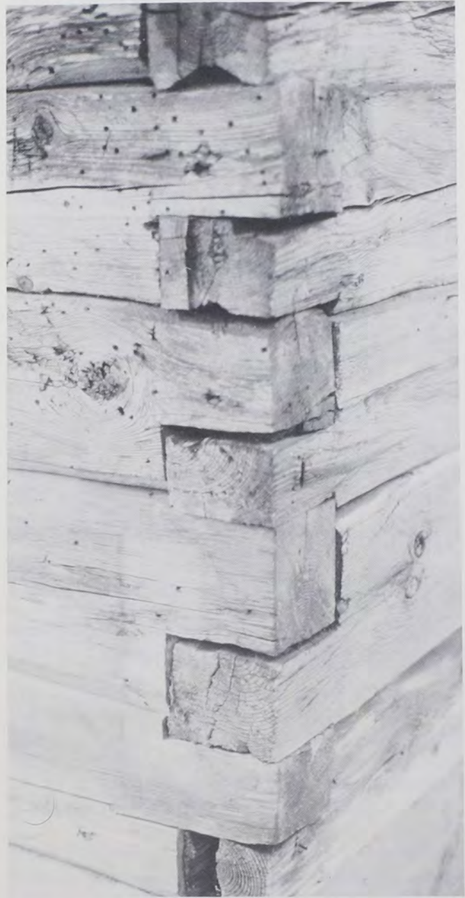
Fig. 20: Half-notched storage shed, built in the 1700s, at Voxtorp open-air museum, Småland province, Sweden. (Photo by T.G.J., 1989)
