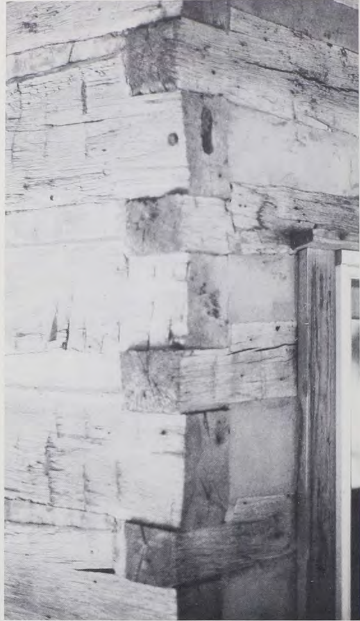
Fig. 11: Half-notching on a hewn-log house in Conway, Faulkner County, Arkansas. The half notch is best classified as a subtype of square notching. (Photo by T.G.J., 1988)
