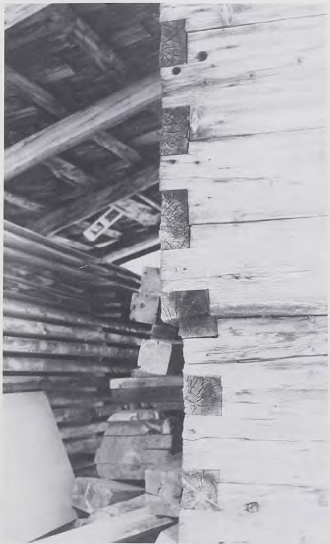
Fig. 16: Square notching on a barn near Kuhtai in the Sellrain Valley, North Tirol, Austria. This is the only structure observed in the entire Alpine mountain chain that displayed square notching throughout. (Photo by T.G.J., 1978)
