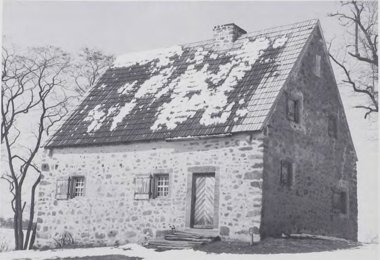
The Herr house was built in 1719 in a typically Germanic architectural style. It has a central chimney and a double attic.
