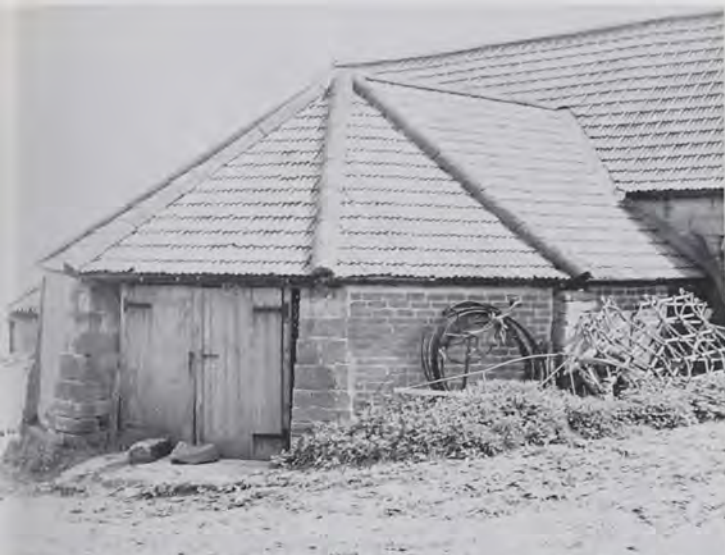
Threshing-wheel shed. Hinderwell, Yorkshire. The machinery has been removed and the building is now used for other purposes.
