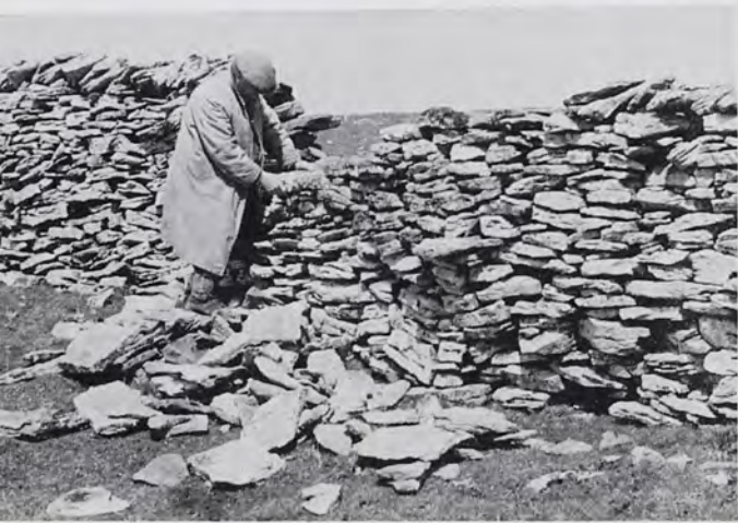
Drystone walling. Oughtershaw Side, Langstrothdale, Yorkshire. Farm worker filling a gap as best he can—regular coursing of the stones is often very difficult to achieve. "Wallheads" are however generally rebuilt.
