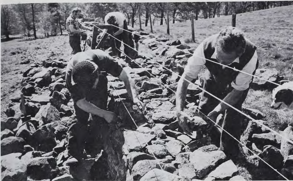
A team of dry-stone dykers at work in the Scottish Borders.
