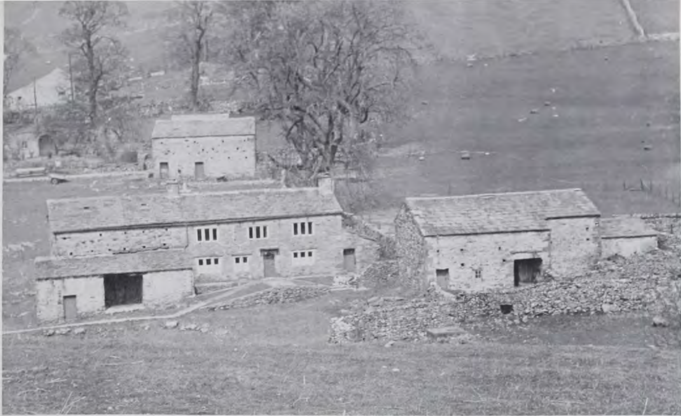
Farm house and buildings, Yockenthwaite, Langstrothdale, Yorkshire, England. Typical Dales farmstead with house and barn adjoining in one long building.
