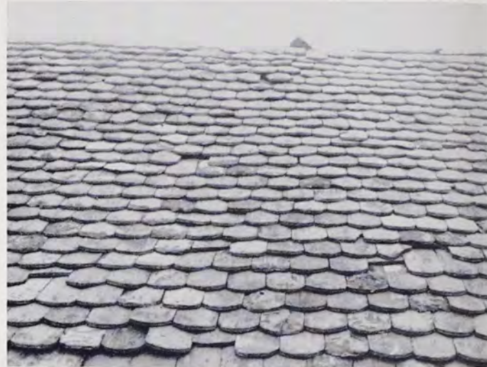
Another "staggered" tile roof on Bernville Road, north of Womelsdorf. Note the ridge tiles.
