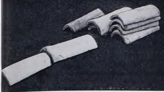
Close-up of ridge tiles. Two tiles in foreground show method of laying tiles on peak of roof.
