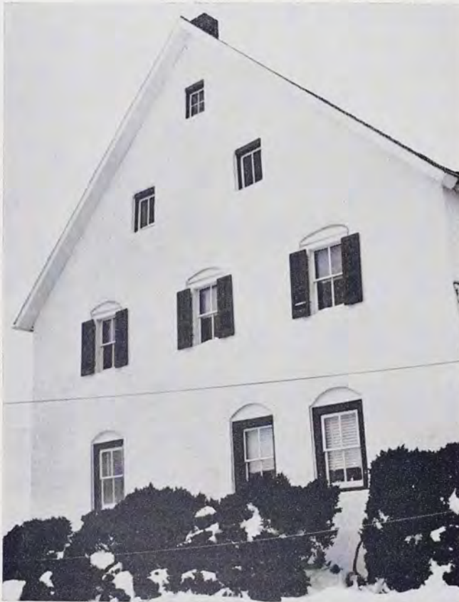
Beautiful gable of Isaac Long House, Landis Valley. Steep roof and deep arches over the windows. Double row of windows in gable is evidence of the original two-story garret, a feature of Colonial Pennsylvania Dutch architecture.
