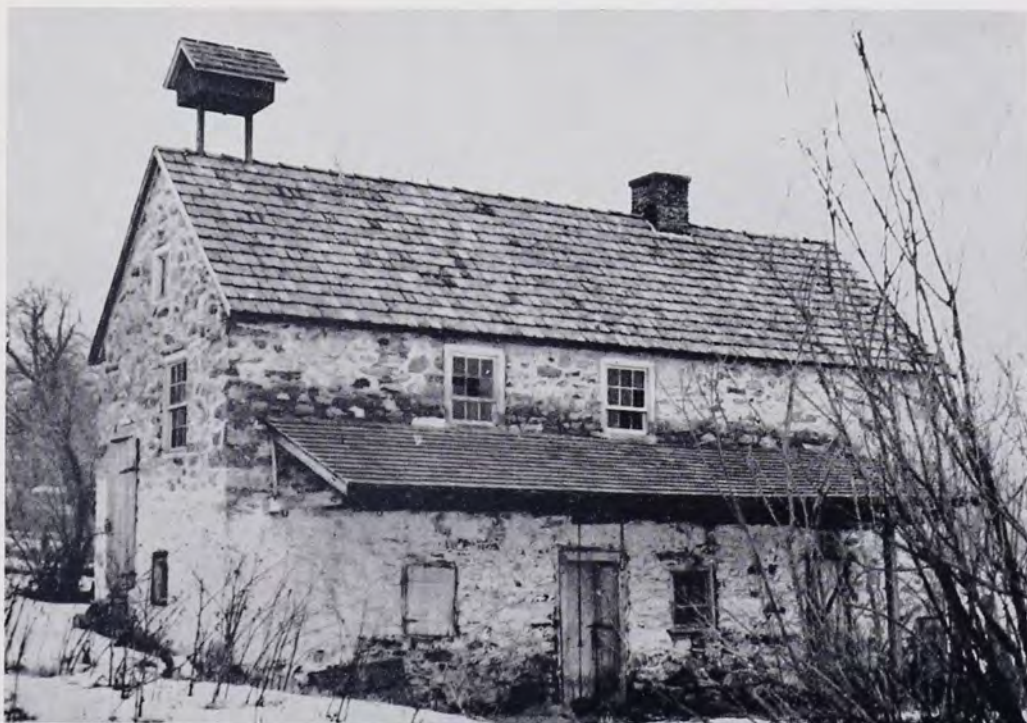
Knabb-Bieber stone cabin, Oley Valley, Berks County. Note the ridge tile and the vertical joints.
