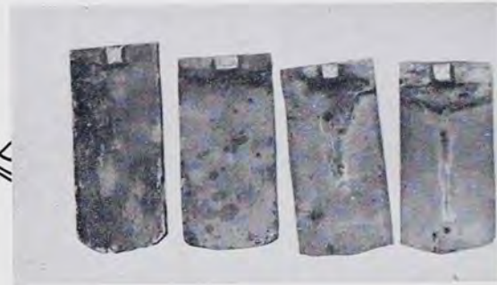
Under side of tile, showing lugs, called shnovvel in Pennsylvania Dutch. Tiles were hung by hooking lug over the horizontal roof laths.
