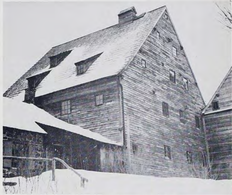
The Saal, Ephrata Cloisters. Medieval Germanic features: steep roof, "kick" at the eaves, many-storied gable and shed-roof dormers.
