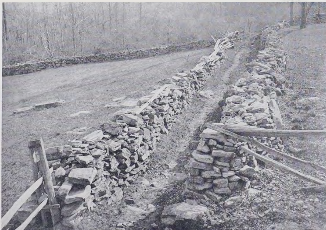
Stone fences dividing fields on a Berks County farm around 1900. Note the rail and rider built on top of the low stone fence in background, left.
