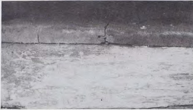
Figure 11. Splined floor boards on second floor.
