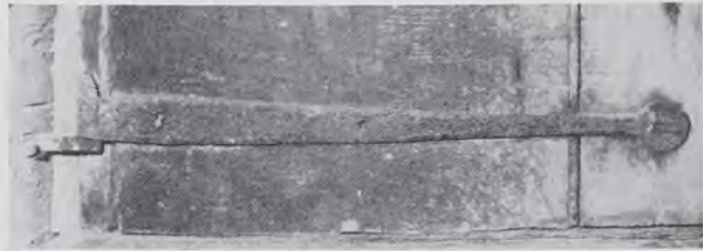
Figure 7. Dovetail, pinned strap hinge on storage area door between fireplace and doorway to upstairs.
