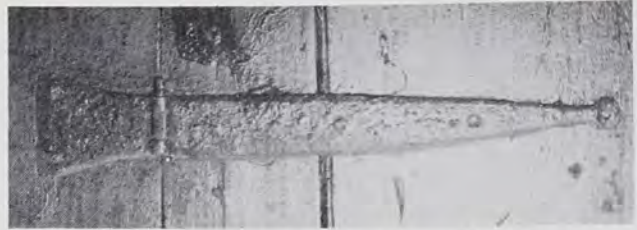
Figure 6. Strap hinge and pintle on doorway to upstairs.
