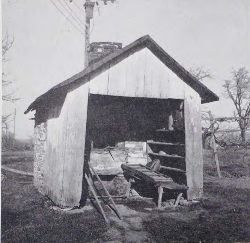
This outdoor bakeoven, located on the Urias Urich farmstead, South Annville Township, Lebanon County, is a combination stone and frame structure with brick chimney. Below, the interior view shows large ashpit beneath oven chamber, wooden drying trays inside oven and one resting on bench. Baking utensils, on left, are scraper and peel.
