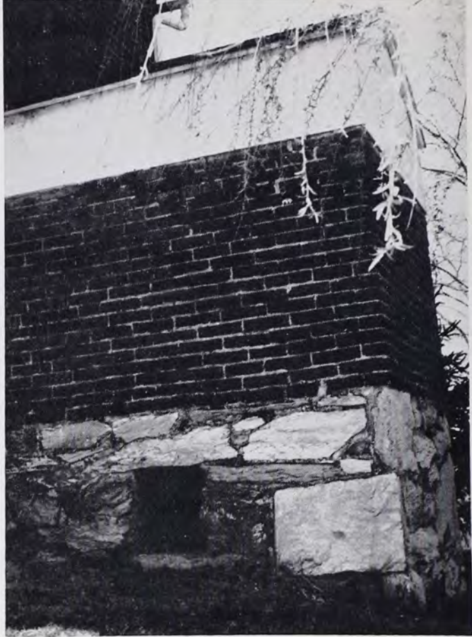
19th-Century attached bakeoven located on the James Monteith farm, North Annville Township, Lebanon County. Note opening into ashpit.
