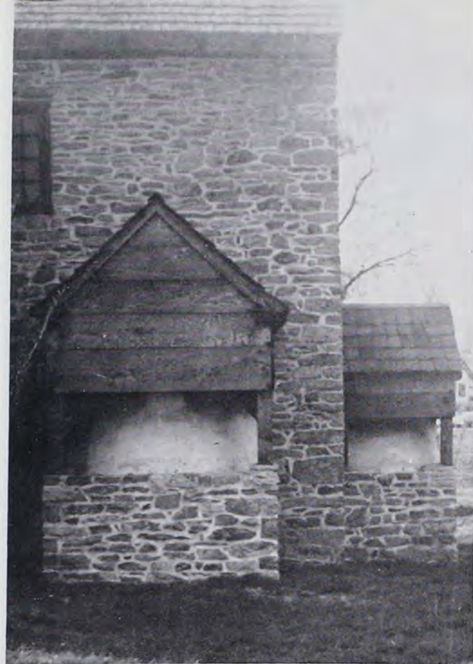
Restored attached bakeovens at Ephrata Cloisters, Lancaster County, constructed of stone and wood with tile roof.
