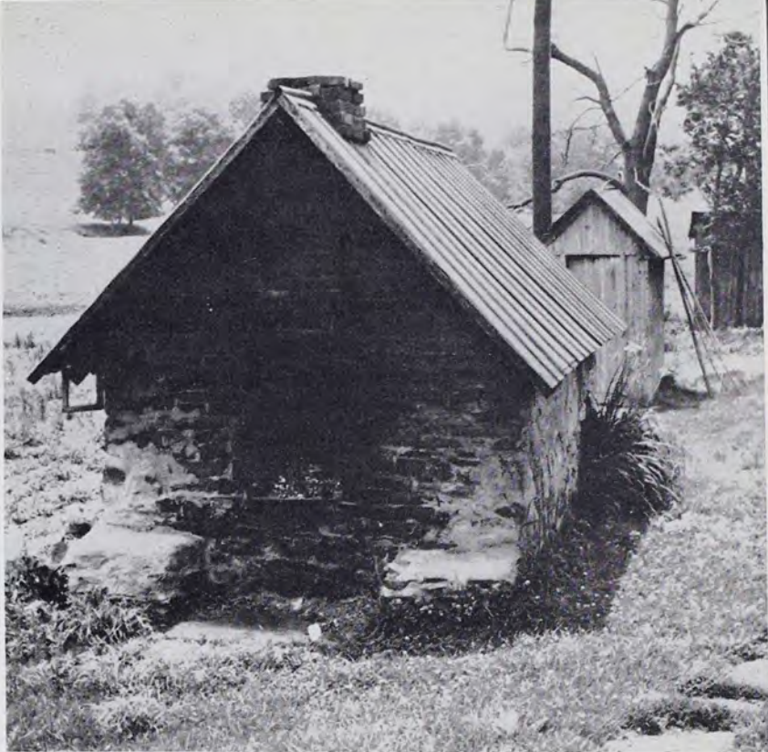
Bakeoven-smokehouse, on the Clarence Naftzinger property near Bernville, Berks County, measures 16 feet long, 7½ feet wide and 9 feet high.
