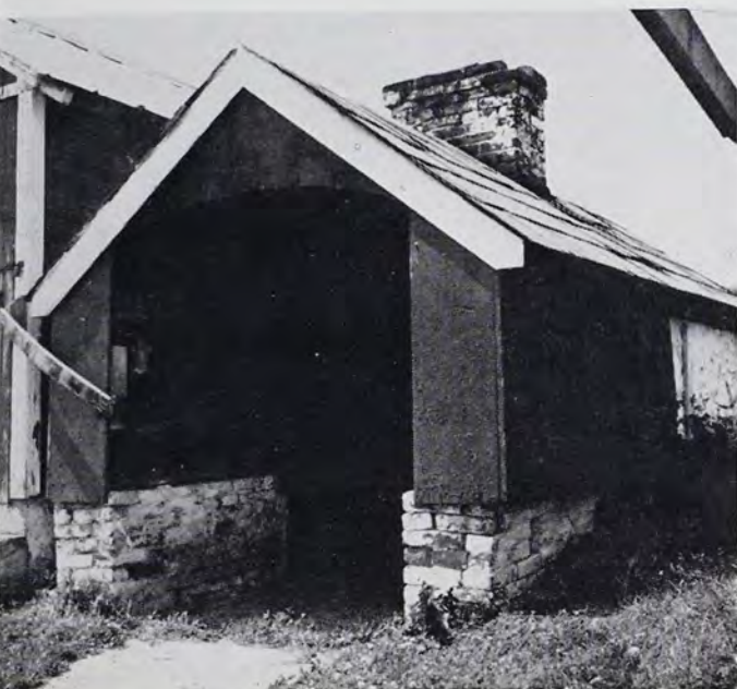
Stone, brick and frame construction were used in this outdoor bakeoven in the Bernville area, owned by Leroy Forry.
