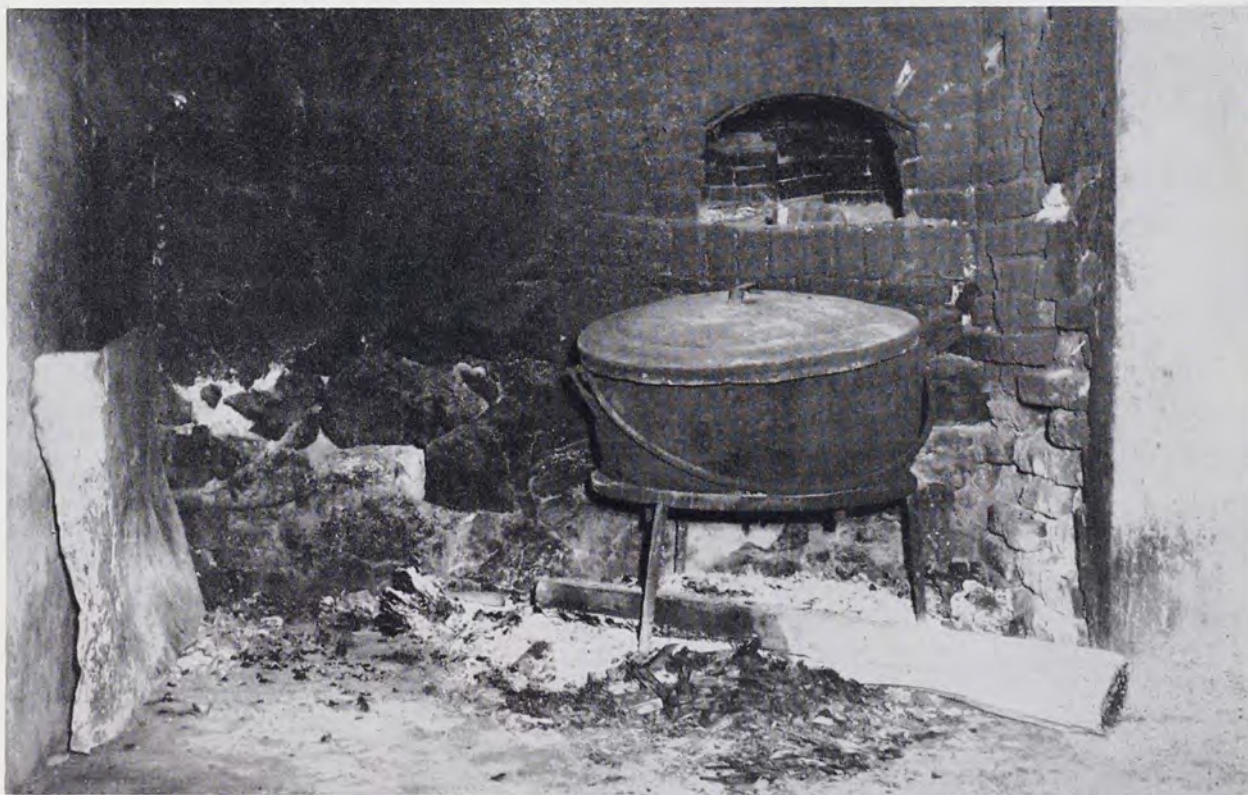
Fireplace bakeoven located in the summer house of the Edward Hartman property, north-east of Reading. The iron kettle in front of the oven is used to heat water for the laundry.
