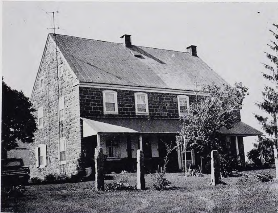
The Valentine Viehman house in Milbach Township, Lebanon County. Grain was hoisted to attic through opening in gable on left.
