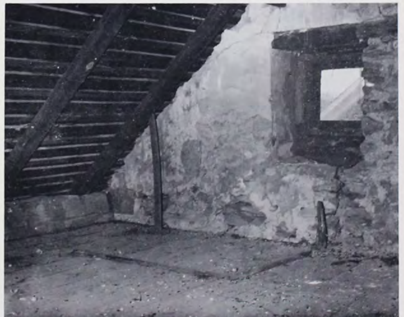
North end of Handwerk attic, showing outline of original grain bin.
