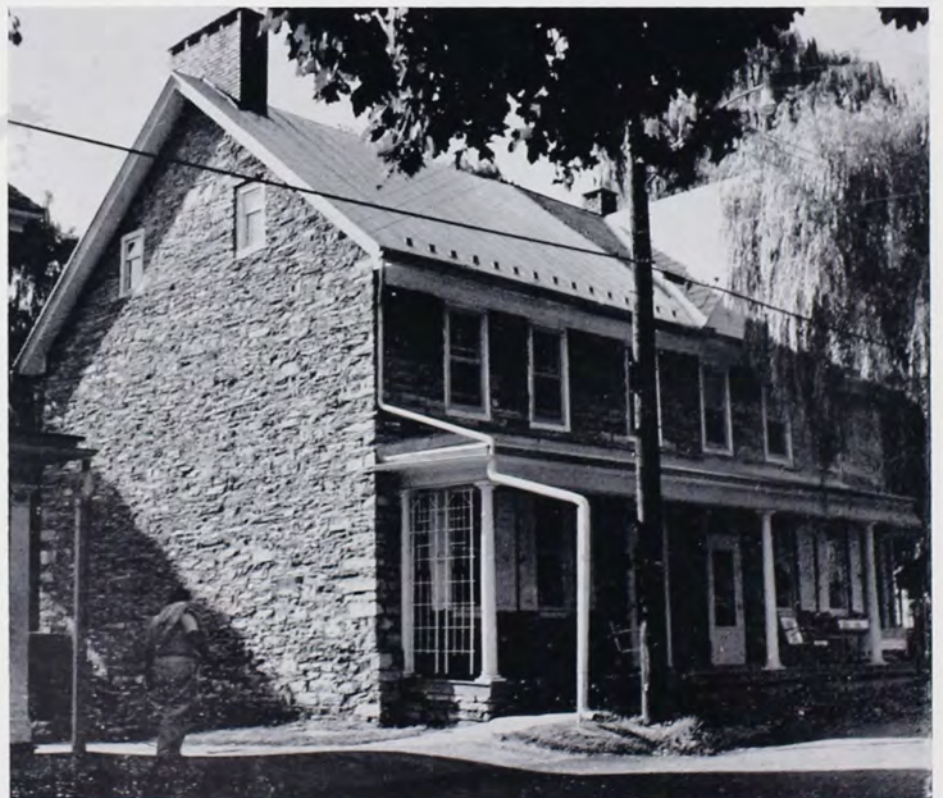
Exterior of Charles Mock House in Schaefferstown, Lebanon County. Much evidence of grain storage in attic, unusual roof structure. House had tile roof originally.
