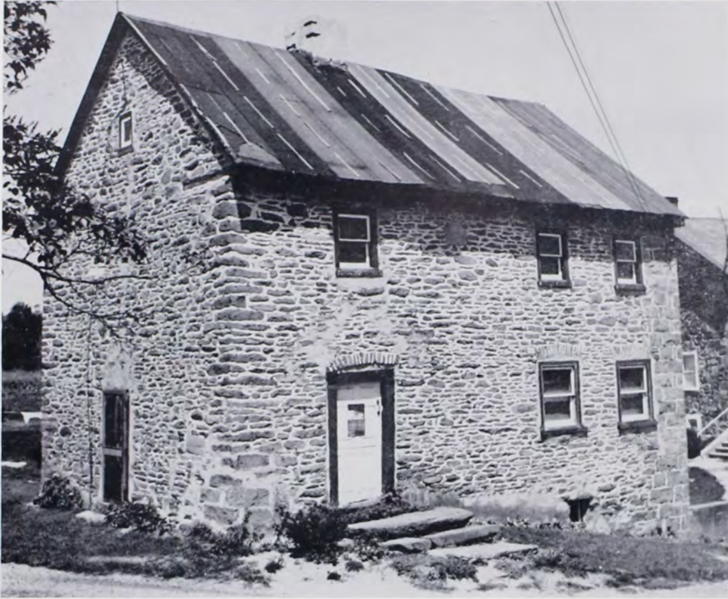
The Handwerk house, 1769, near Germansville, Lehigh County. House has rare reception hall inside front door (white).
