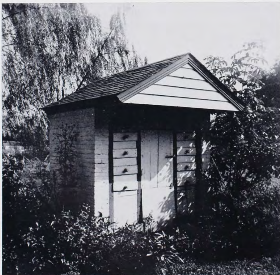
LANCASTER COUNTY DRYHOUSE. Built about 1850, this attractive brick dry-house stands on the Noah Getz Farm, Route 3, Lancaster. It was last used in 1946. Measurements: length 5 ft., width 7 ft., height 8 ft., height to overhang 6 ft. Four top drawers are 5 ft. long and 24 in. wide. The eight drawers, four on each side, are 5 ft. long and 16 in. wide. The overhang extends two ft. forward. Photo taken 1961 by Amos Long, Jr.
