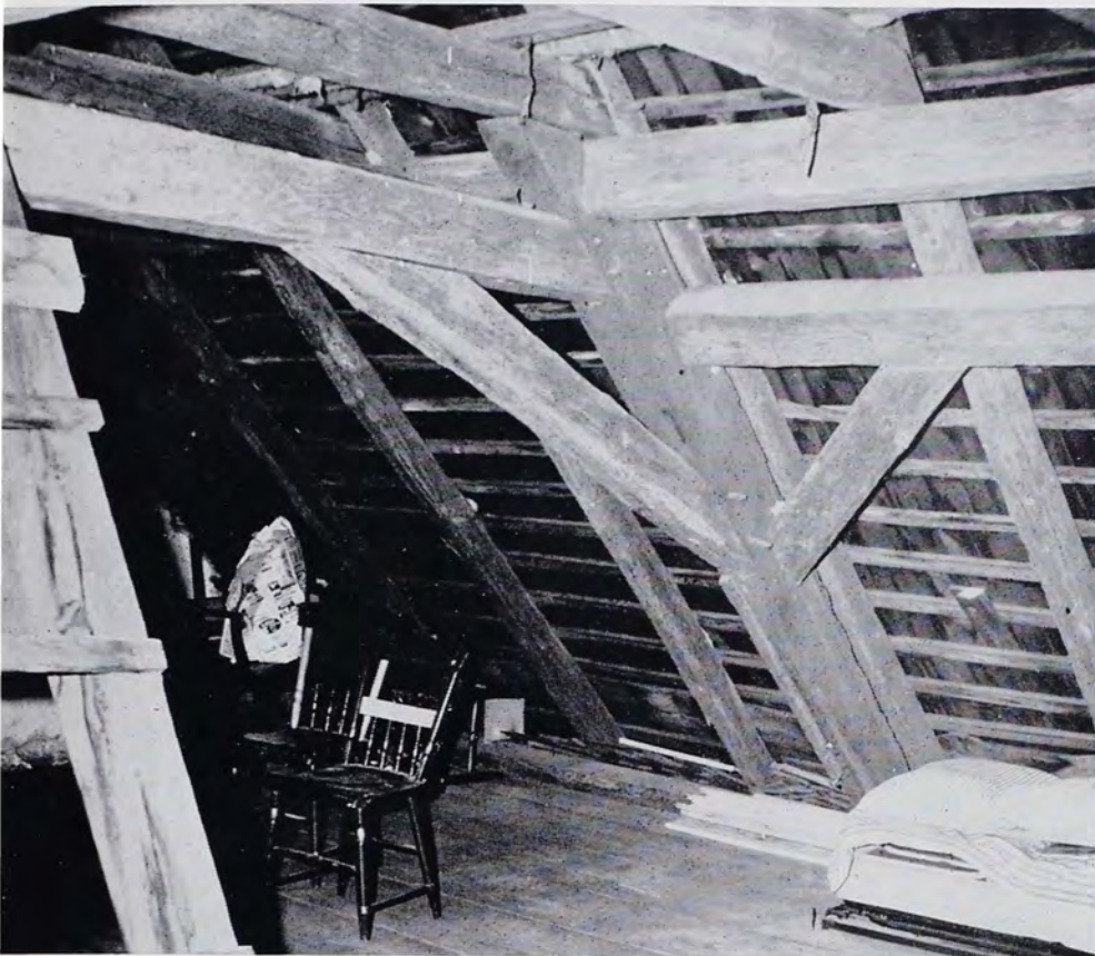
Attic of Viehman house showing 1" x 3" strips on under side of king rafter, just above floor level on right. These strips held board sides of grain bin in place. Full width of attic was used for grain storage between strips and stone wall in rear of photo.
