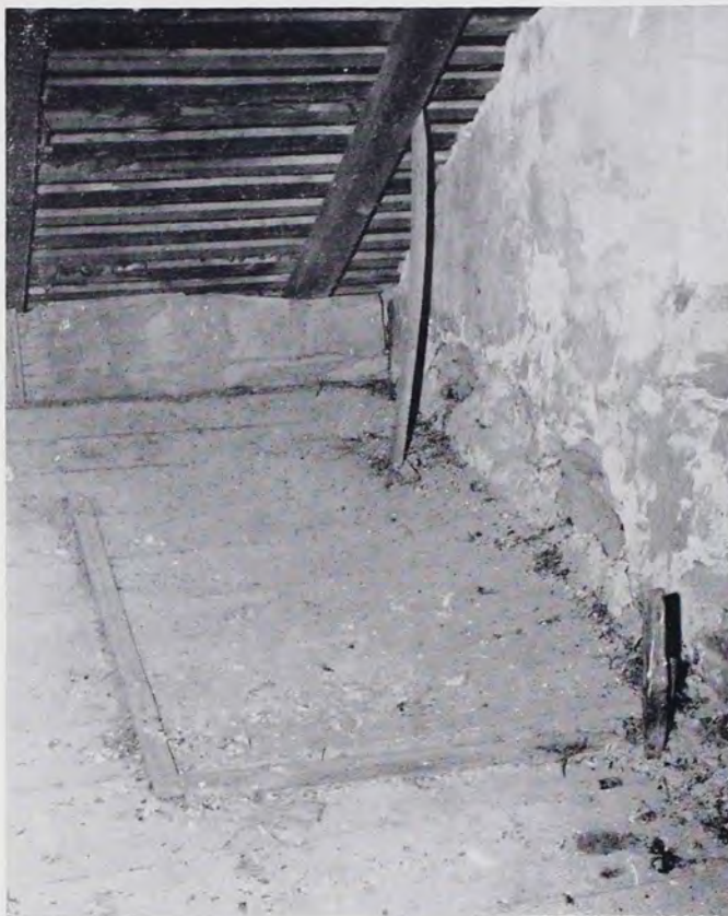
Close-up of grain bin area in Handwerk house. Bins originally had wooden board sides about 3 feet high.
