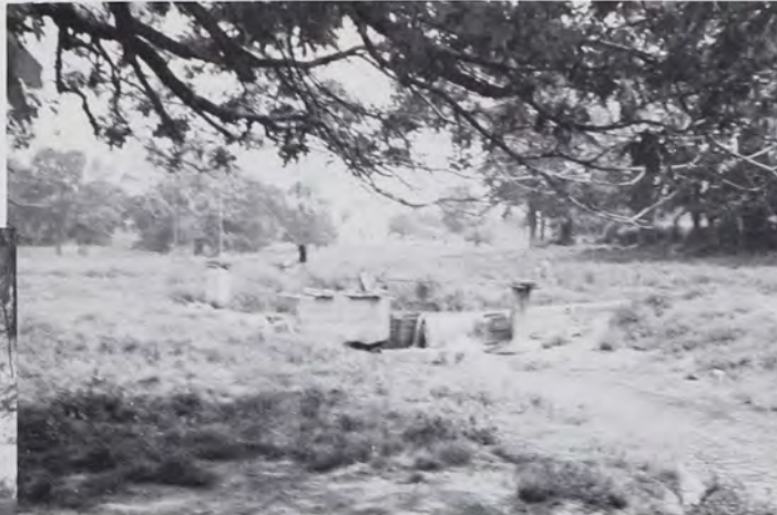
Early pump in a Lancaster County stream used for irrigation and other farm purposes.
