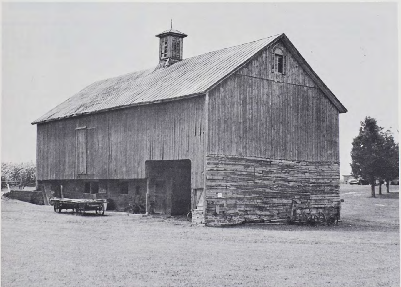
FIG. 9—Pennsylvania Barn Type F-G. Located west of Hereford, Baltimore County, Maryland. At the right end is a wagonway with a corner crib to one side (August, 1965).
