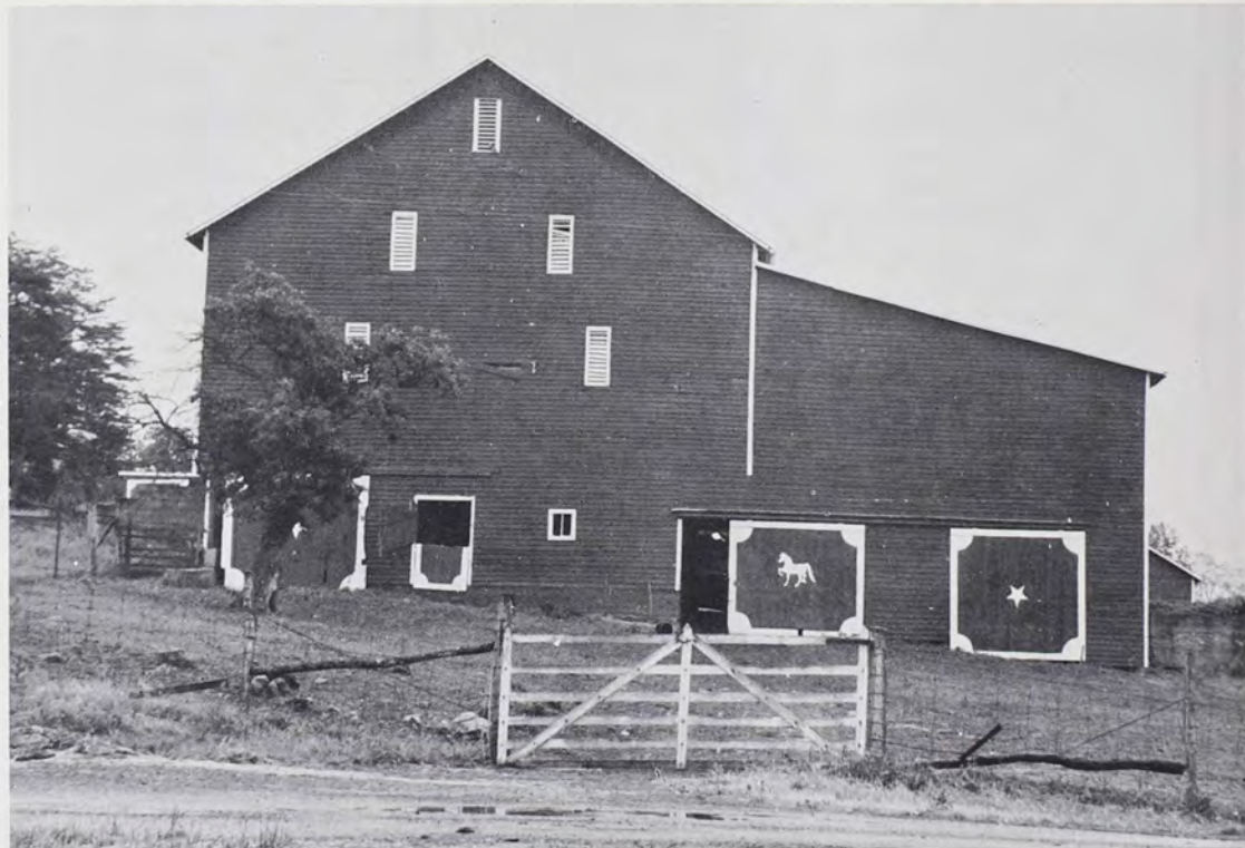
FIG. 16—Pennsylvania Barn Type F-G With Rear Shed. Located between Parnassus and Churchville, Augusta County, Virginia. The decorative painting on this barn is typical of the central Valley of Virginia (June, 1964).
