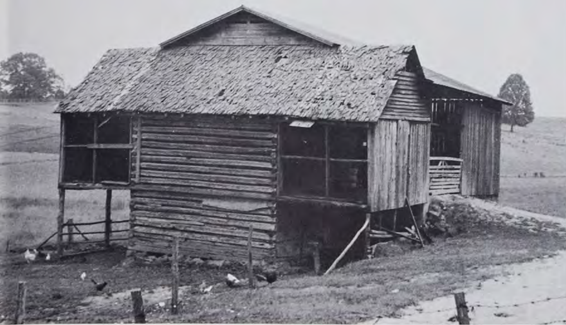
FIG. 25—Double-Crib Barn with Overhanging Loft. Located across the French Broad River from Alexander in Buncombe County, North Carolina. This barn appears to be transitional between the double-crib barn with overhanging loft and the Pennsylvania barn type F-G because of the presence of the ramp; compare it with the barns in Figures 17, 18, and 6 (June, 1963).
