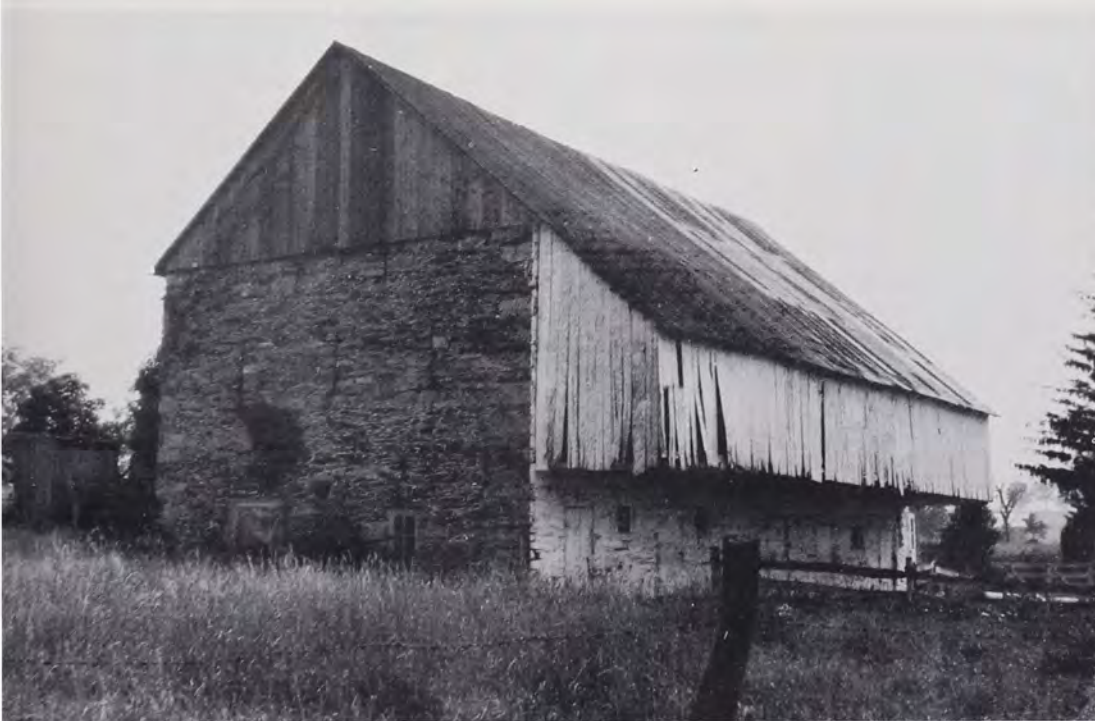
FIG. 21—Pennsylvania Barn Type F-G. Located in Wolfville, Frederick County, Maryland. Like the stone barn in Fig. 12 and the brick barn in Fig. 8, this barn has loopholes for ventilation (July, 1963).
