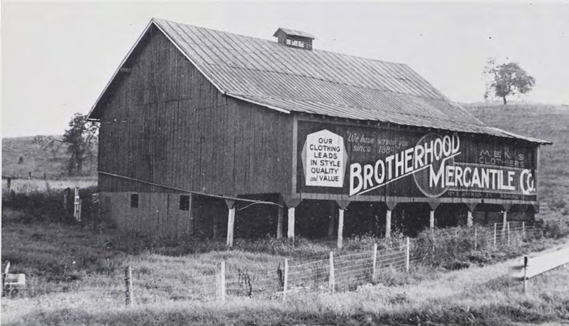
FIG. 15—Pennsylvania Barn Type F-G With Extended Forebay. Located south of Buchanan, Botetourt County, Virginia. The vertical board siding and extended forebay are typical of this section of the southern Valley of Virginia (August, 1965).
