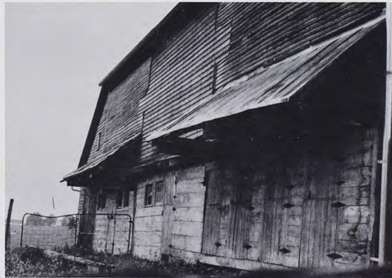
FIG. 2—Pent Roof on the Rear of a Pennsylvania Barn Type E Located between Harrisonburg and Dayton, Rockingham County, Virginia. Note that the rear of the stabling area is sided with horizontal planks as is often the case in Maryland and Virginia (June, 1964).
