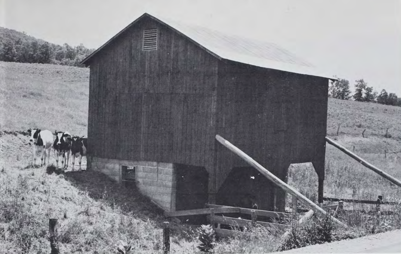
FIG. 5—Pennsylvania Barn Type F-G. Located between Augusta and Rock Oak, Hampshire County, West Virginia. The Pennsylvania barn tradition remains strong in this part of the Alleghenies; this small barn is typical of those recently constructed in the area (note the cement block basement). If no hillsides are available an artificial hill is constructed for the barn, rather than building it flat on the ground with a ramp up to the second level. Barns with the forebay supported in the rear by posts in exactly this manner (the poles set in at an angle are an afterthought necessitated by heavy modern traffic) are found in western Pennsylvania, western Maryland, northeastern West Virginia, and the southern Valley of Virginia (June, 1964).
