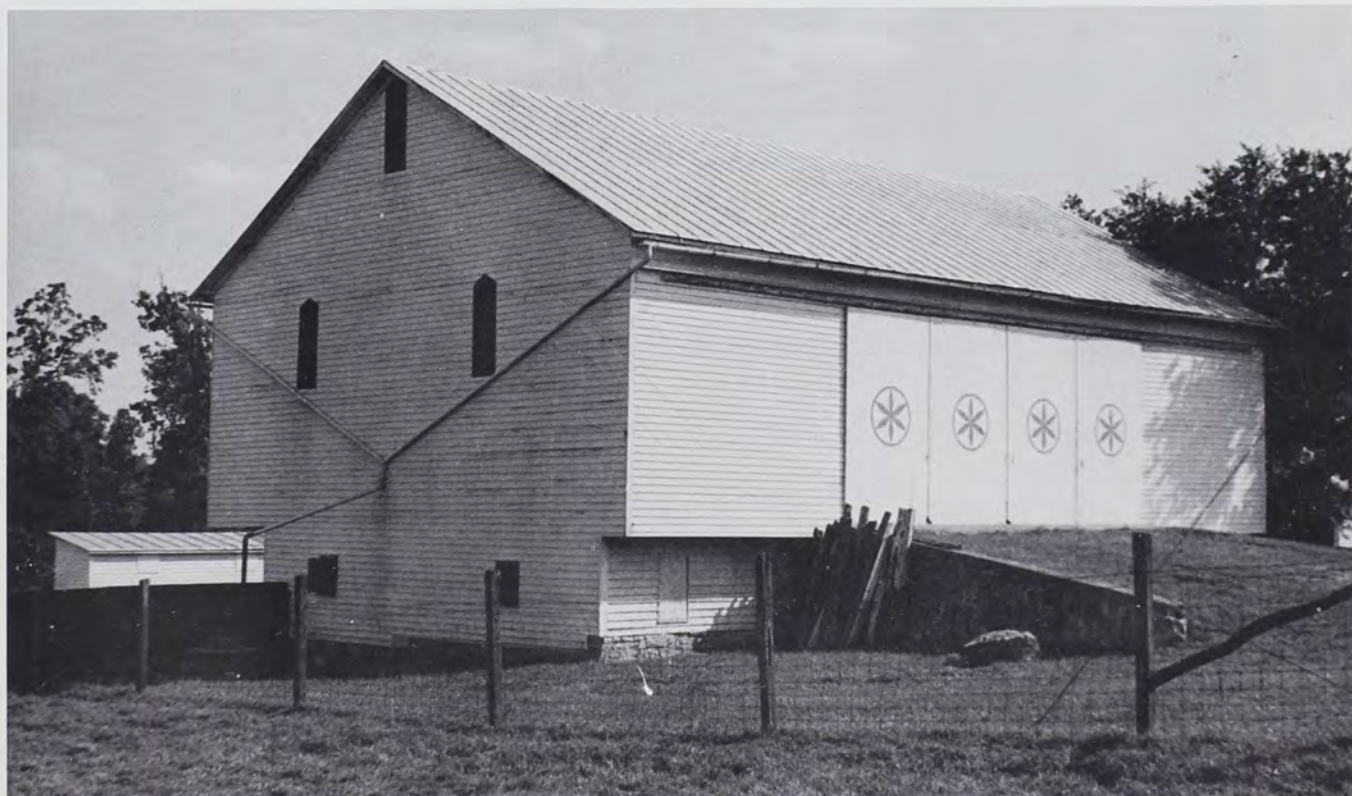
FIG. 6—Pennsylvania Barn Type F-G. Located north of Mount Sidney, Augusta County, Virginia. The overhang on the front, the clapboarding, and the Gothic louvers are typical of the central Valley of Virginia. The decorations on the door, painted in green, are of a type more usual in Pennsylvania than in Virginia (August, 1965).
