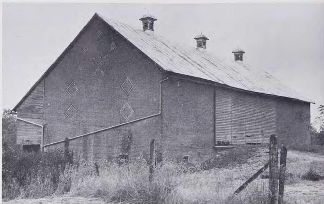
FIG. 22—Pennsylvania Barn Type F-G. Located in Timberville, Rockingham County, Virginia. This barn is the most southerly example yet discovered of a brick Pennsylvania barn. It is laid entirely in Flemish bond. The hollow diamond motif does not seem to be usual in Pennsylvania; the solid diamonds and the X, however, are common (July, 1964).
