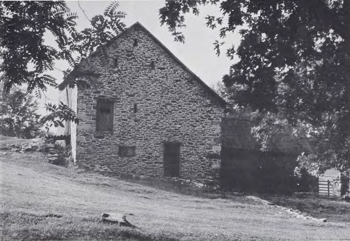
FIG. 12—Pennsylvania Barn Type H. Located south of Purcellville, Loudoun County, Virginia. The low rear ell for additional stabling is a common feature of older barns in this area (August, 1964).
