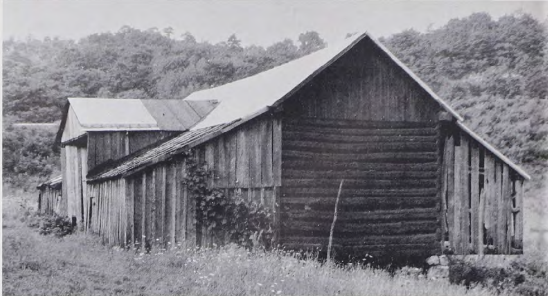
FIG. 18—Pennsylvania Barn Type F-G. Located at the crest of the Blue Ridge in Nelson County, Virginia. The upper level is composed of two eighteen foot square V-notched log cribs with a central threshing floor and a frame forebay on the rear and frame sheds on the front. The basement is composed of stone piers at important structural points with the intervening areas covered with vertical boards (August, 1964).
