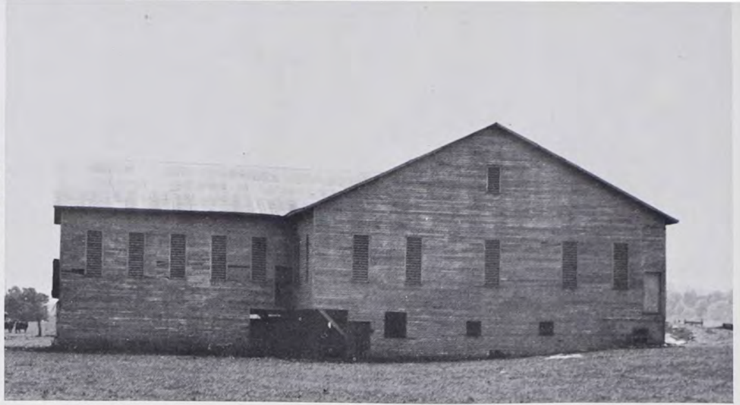
FIG. 14—Pennsylvania Barn Type F-G With Central Rear Ell. Located south of Cumberland Gap, Claiborne County, Tennessee. This is the Pennsylvania barn which has been located in the South at the greatest distance from Pennsylvania (June, 1964).
