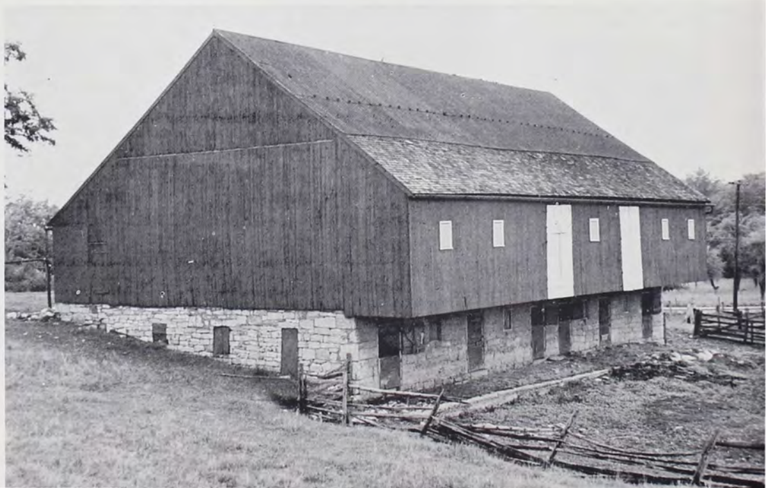
FIG. 20—Pennsylvania Barn Type F-G. Located between Cavetown and Hagerstown, Washington County, Maryland. Note that this barn has sheds on the front which balance the forebay in the rear, and a full stone basement (contrast with Fig. 1). Like the majority of the barns in Pennsylvania and Maryland it is painted red (August, 1965).
