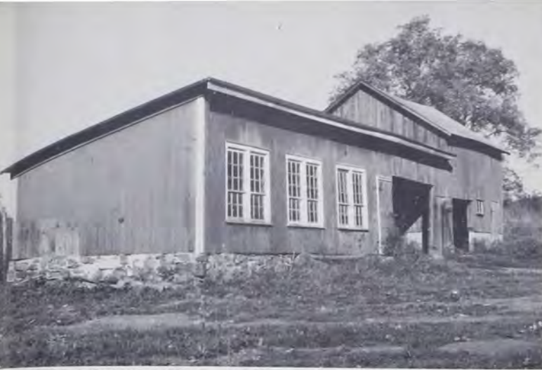
Frame Chicken House attached to small barn on author's farm, North Annville Township, Lebanon County, 1967. Dimensions: 30' x 16'; height 10' in front, 6' in rear. Note stone foundation and 9 over 6 glass windows.
