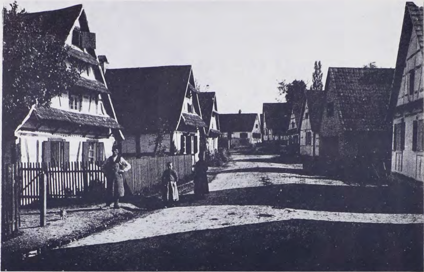
Quiet reigns in Scheibenhart. Note half-timbered houses, also pent roofs to protect walls and window frames from weathering—the continental root of Pennsylvania's "Germantown Pent Roof"
