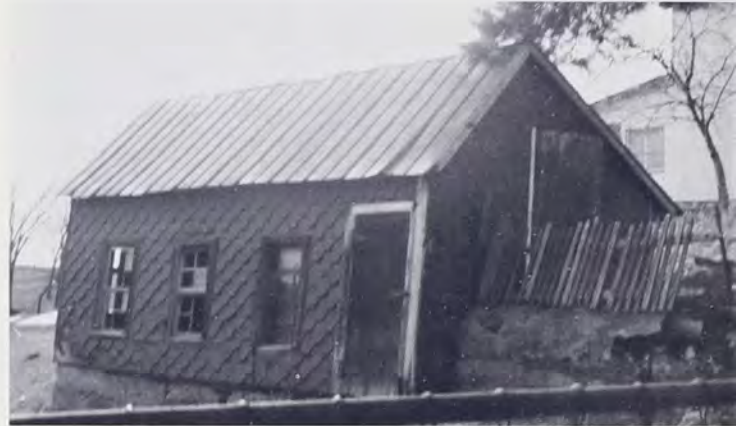
Frame Chicken House built into hill with recessed floor, Noah Redcay Farm, near McGillstown, Lebanon County, Pennsylvania, 1968. Length 22', width 12'. Note two levels of entrance. This structure is no longer in use, and demolition is planned.
