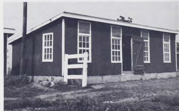
Frame Chicken House, Harold G. Ryder Farm, Route 7, Chambersburg, Franklin County, Pennsylvania, 1967. Length 34', width 15', height 8' in front, 6' in rear.
